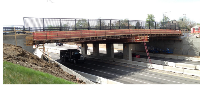
Knox Court bridge
