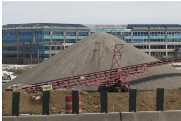
Stockpile of recycled asphalt to be used for road base
