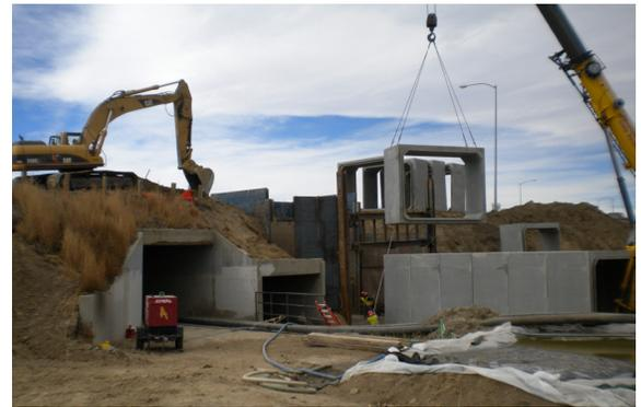
Installation of drainage and a pedestrian tunnel on Big Dry Creek Trail
