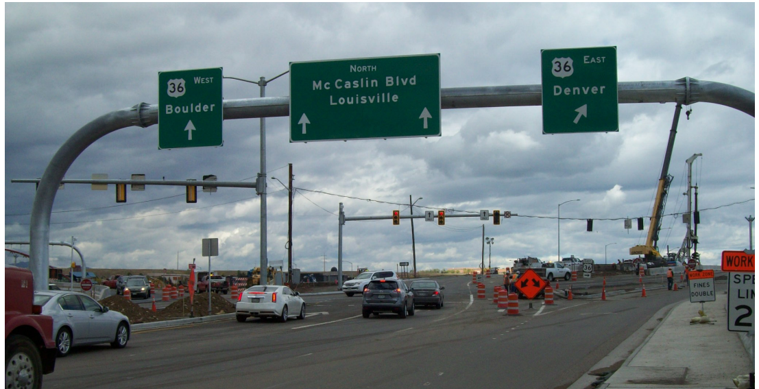
McCaslin Boulevard's Diverging Diamond Interchange
