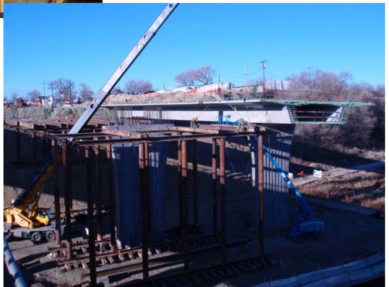
Figure 11 – Span 1 EB CIP Superstructure Construction– February 4, 2009:
