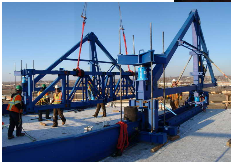
Figure 8 – Pier Table 3 WB Form Traveler Erection– January 27, 2009:
