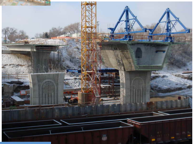
Figure 7 – Pier Table 3 WB Form Traveler Erection – January 27, 2009:
