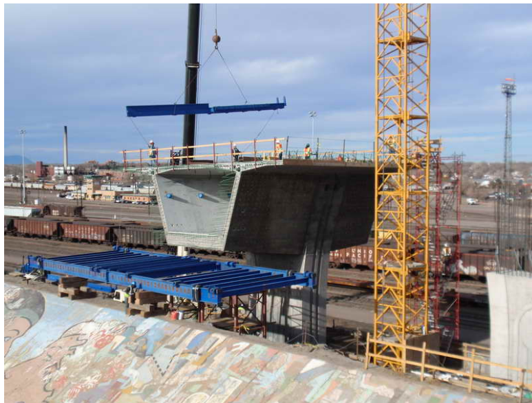
Figure 6 – Pier Table 3 WB Form Traveler Erection – January 22, 2009:
