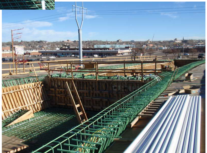
Figure 5 – Span 5 WB CIP Superstructure Construction – January 22, 2009:
