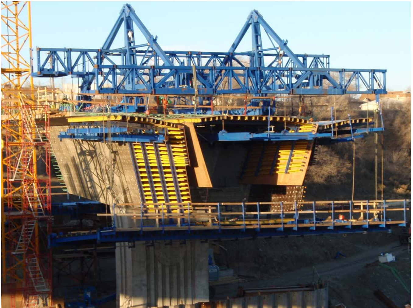
Figure 12 – Cantilever 3 WB Form Traveler Erection– February 6, 2009:
