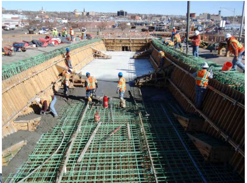
Figure 9 – Span 5 WB CIP Superstructure Construction– January 29, 2009:
