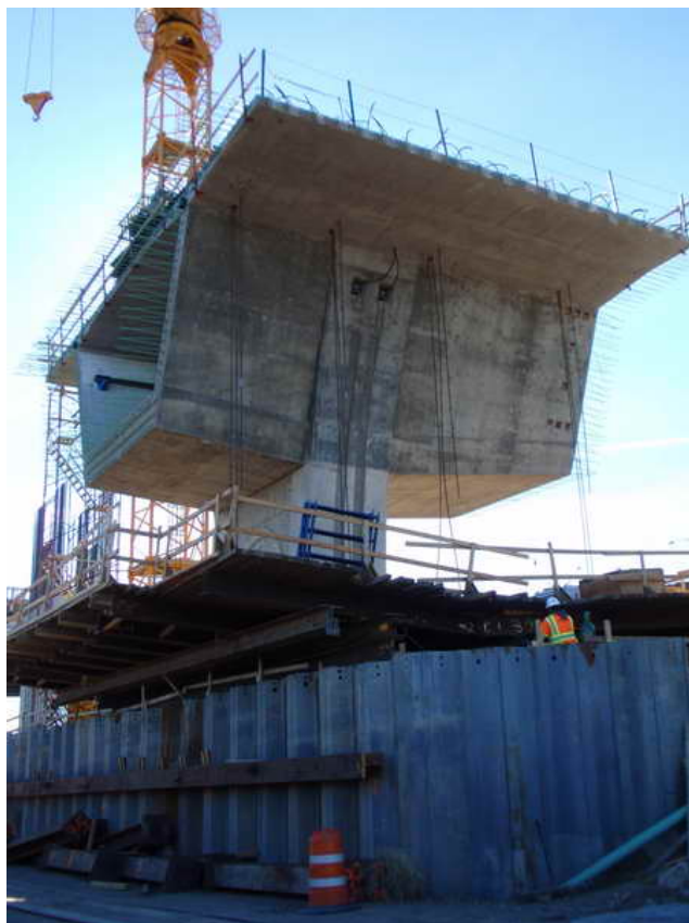
Figure 2 – Pier Table 3 WB Falsework Removal – January 19, 2009:
