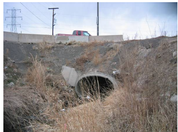
52 EXHIBIT 5-4: DRY GULCH CULVERT
