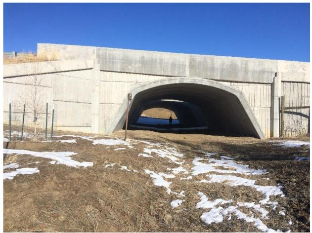
Figure 3. Monitored Wildlife Crossing Structure US 160 MP 97.42. The Monitoring Camera and Post at the South Entrance are in the Foreground. Cameras Faced the Entrances.
