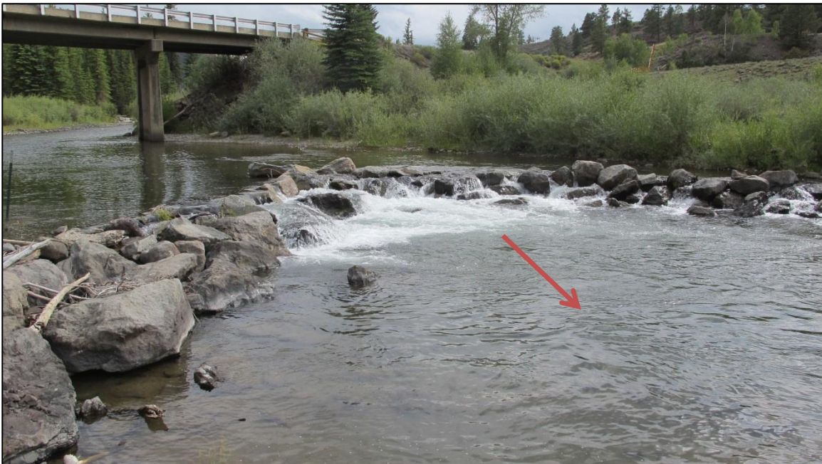
Figure A.13.10. Looking at drop structure downstream of bridge
