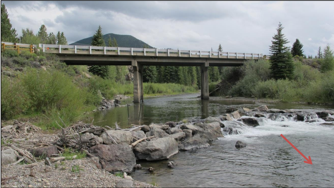
Figure A.13.9. Looking at drop structure downstream of bridge
