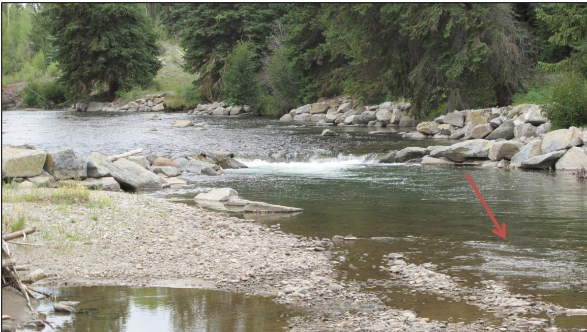
Figure A.13.12. Looking at drop structure and dikes upstream of bridge
