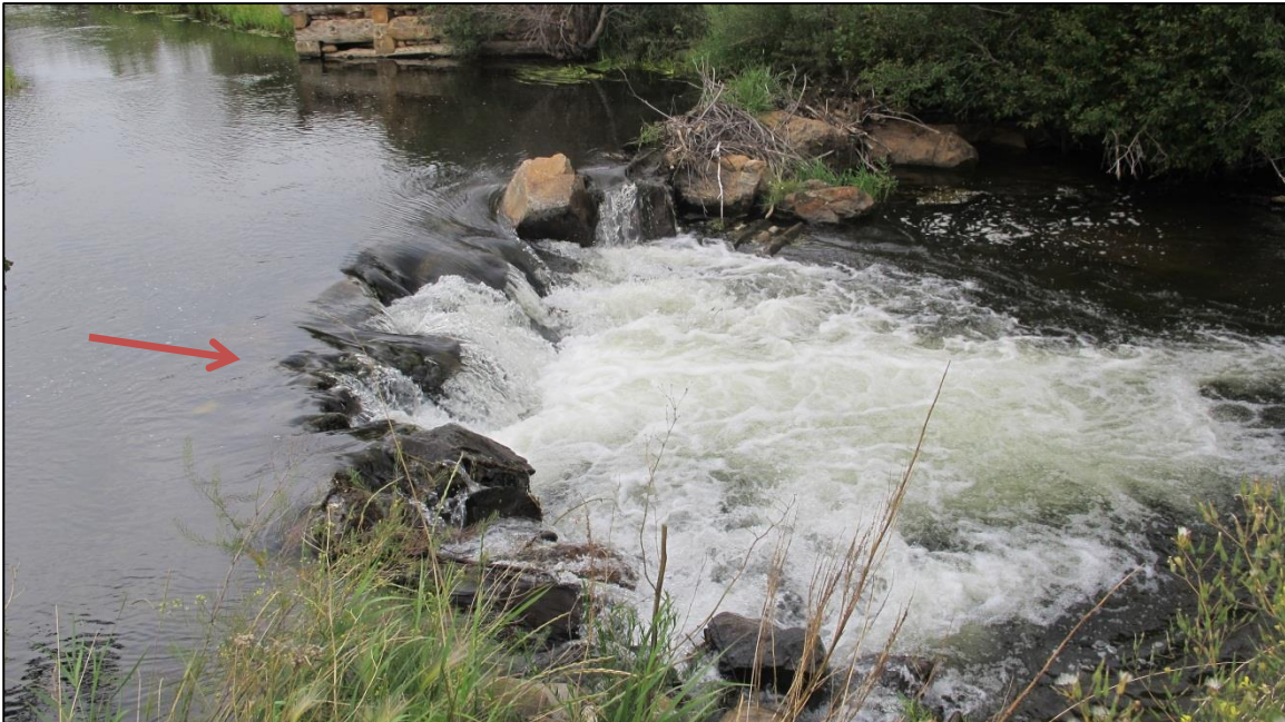
Figure A.12.10. Looking at drop structure downstream of bridge
