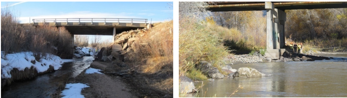
Figures 3.1 and 3.2 Field inspection of scour-critical bridges
