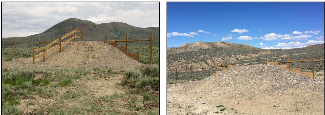
*Figure 17.* Examples of escape ramp with 2:1 slope and rail fence (left) and 3:1 slope with no rail fence (right).
