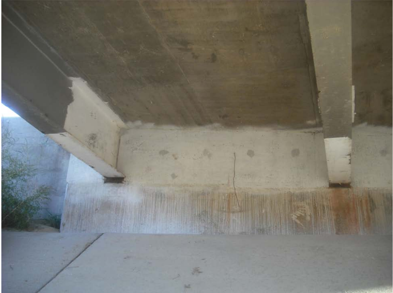
Figure 7: SB Abutment Typical SCC Finish
