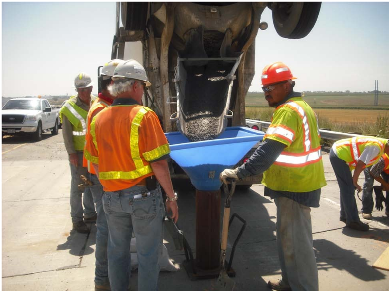
Figure 2: SCC Placement Funnel
