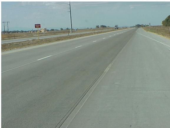
**Figure 4. At accel/decel lanes the stripes were placed outside the grooves.**
