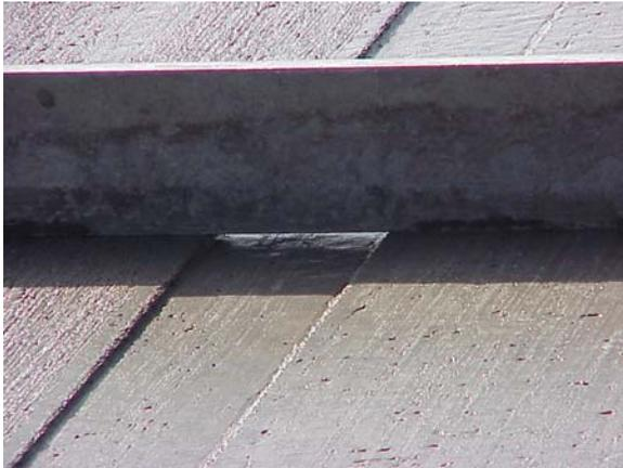
**Figure 1. Shoulder stripe groove formed in plastic concrete.**
