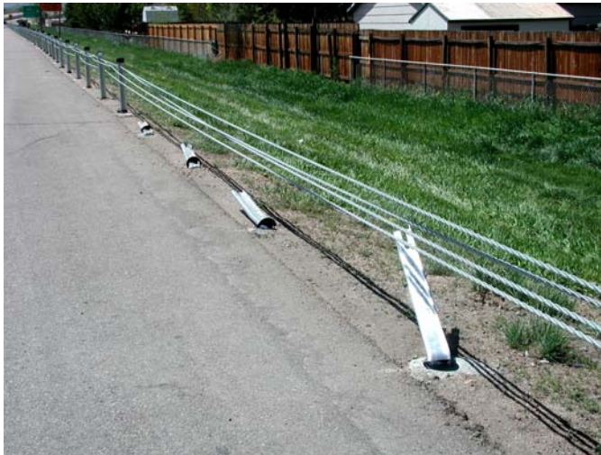
Figure 2. Only four posts were bent in this drive-away accident on US-285 at Kipling.
