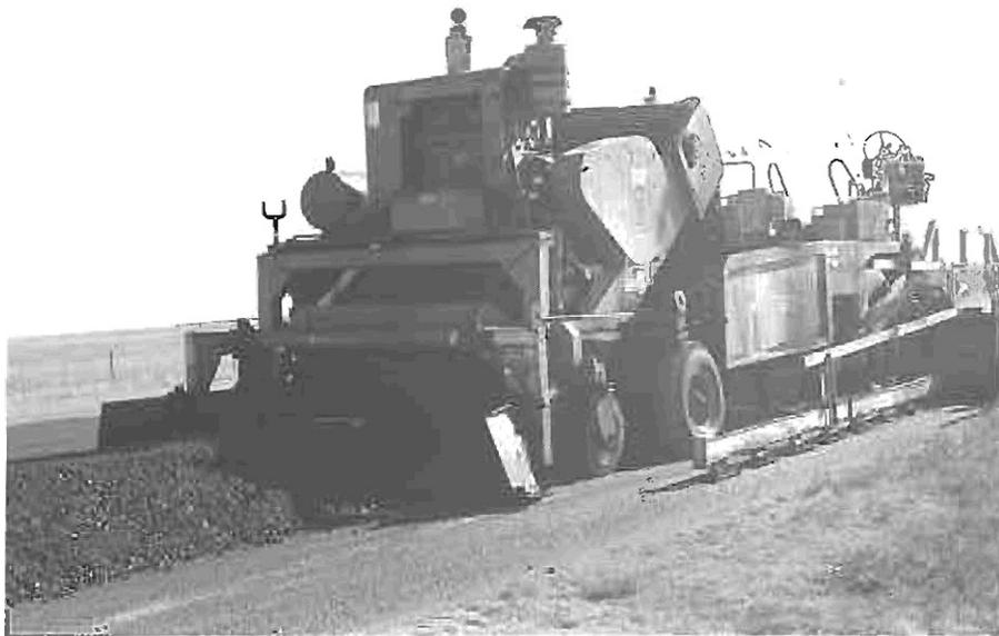
Figure 13 - Elevating loader used to load mix into paver hopper on SH-40.
