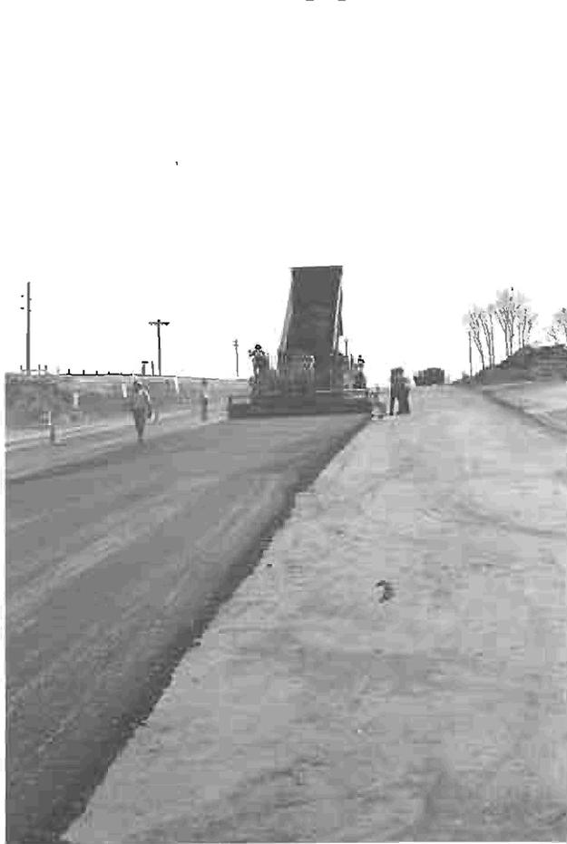
**Figure 4 - End dump used to place mix directly into paver hopper on SH-14.**
