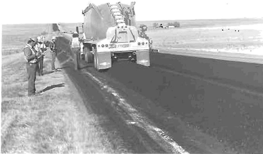
Figure 12 - Bottom dump placing mix in windrow for an elevating loader to place material into the paver hopper.
