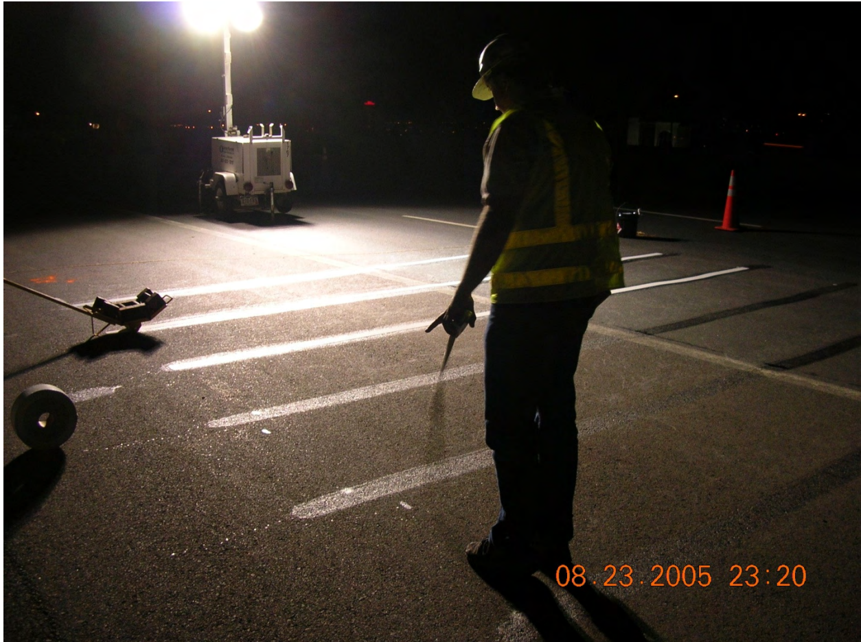
Figure 1. Applying the Lines
