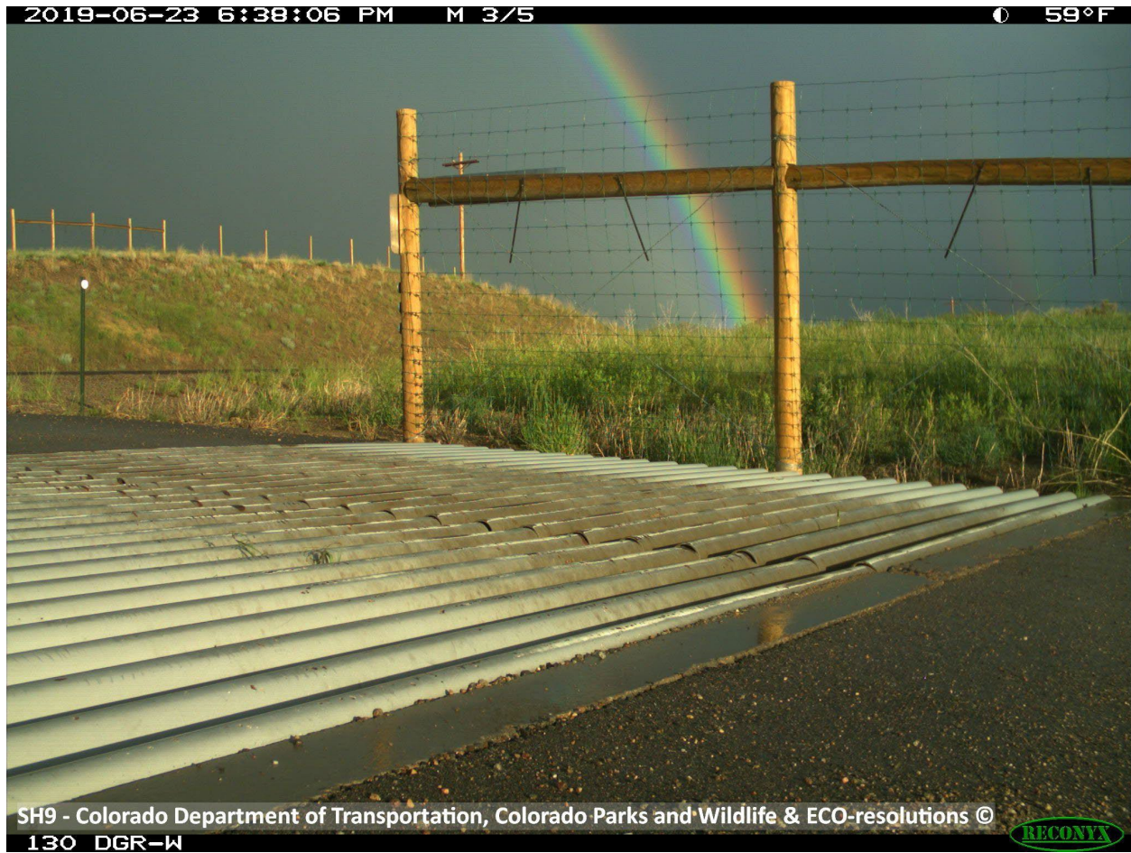
Figure 9. CDOT has tested a variety of wildlife exclusion grates. Is there a pot of gold under this one?
