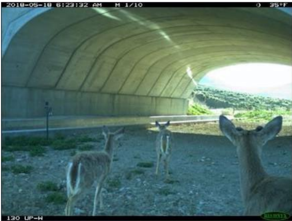
Figure 6. Mule deer approaching the new wildlife underpass for State Highway 9. CDOT research documented a 92% reduction in wildlife-vehicle crashes following the addition of wildlife crossings, fencing, escape ramps, and other treatments at key locations along SH9.
