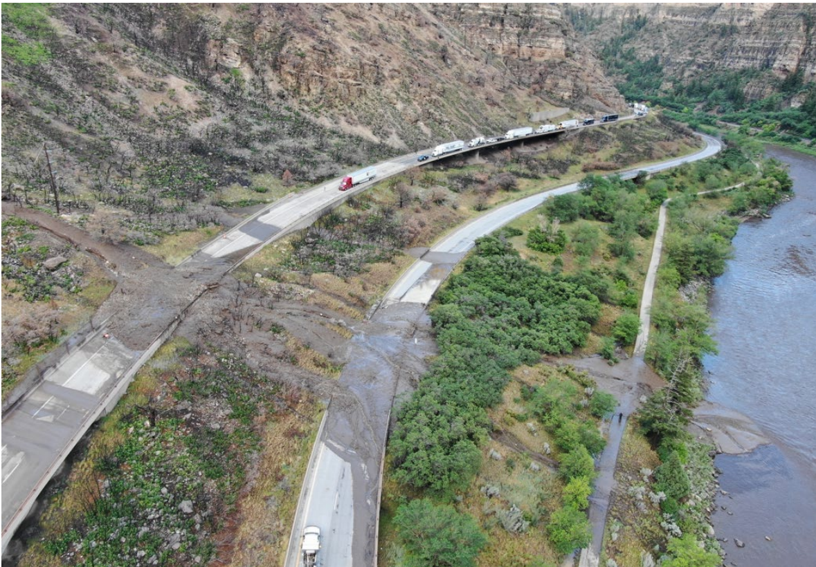
Figure 5. Debris flow damage to Interstate 70 through Glenwood Canyon, CO following heavy rain on the Grizzly Creek fire burn scar.
