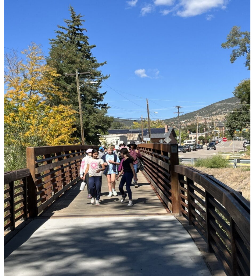
Lyons, Colorado, Pedestrian Bridge
