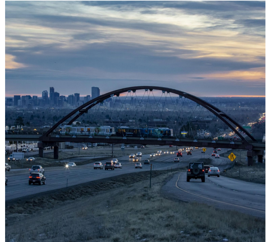
Light Rail bridge over 6th Avenue with view of downtown
