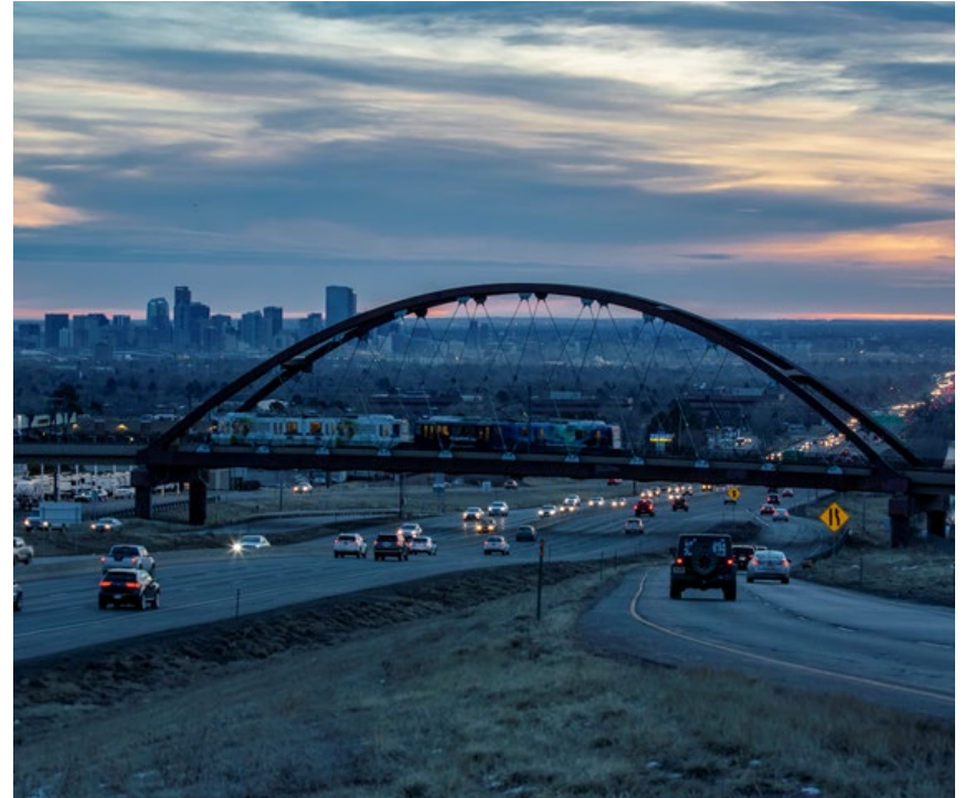
Light Rail bridge over 6th Avenue with view of downtown
