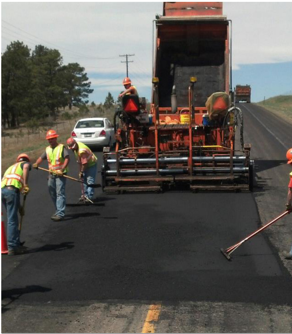
Construction on US 287 in Lamar.
