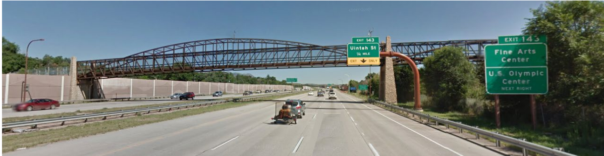
Figure II.11: CDOT-Built Pedestrian Bridge across Interstate 25 in Colorado Springs
