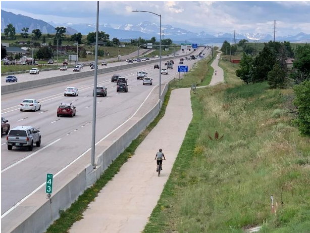
US 36 Bikeway: Separated pedestrian/bike (shared use) facility
