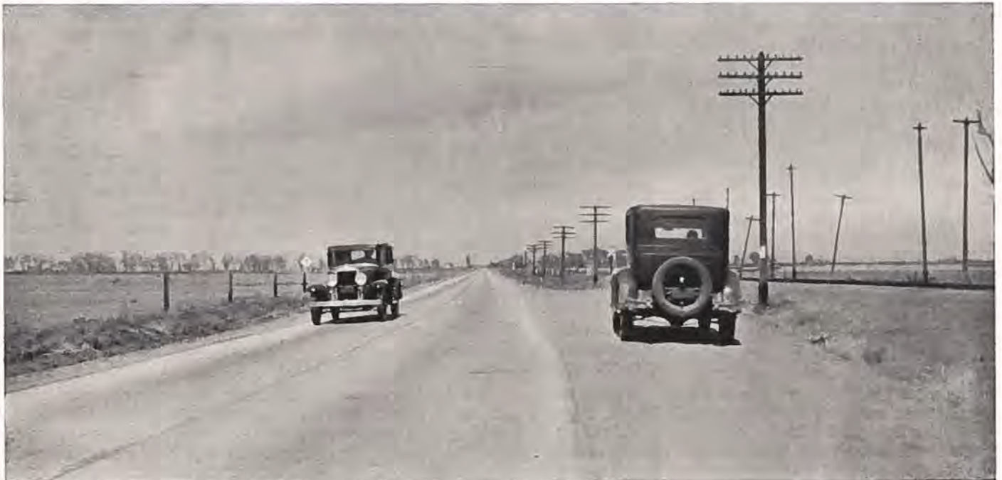
Concrete paved highway between Eaton and Greeley in Weld County.
