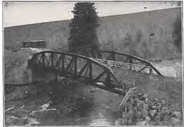
100 ft. Riveted Low Truss Span, Dillon, Colo.
