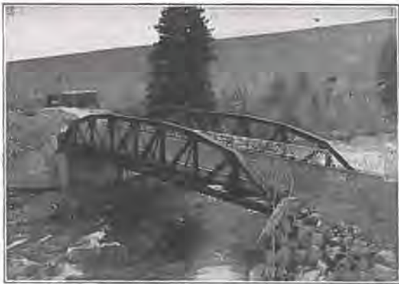
100 ft. Riveted Low Truss Span, Dillon, Colo.
