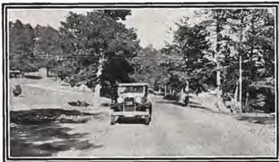
At Bottom — Beautiful Mt. Vernon Canon is now free of dust since this splendid road has been treated with STANDARD Asphalt Road Oil.
