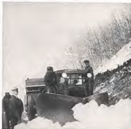
A giant Coleman four-wheel-drive truck clearing snow from Berthoud Pass.
