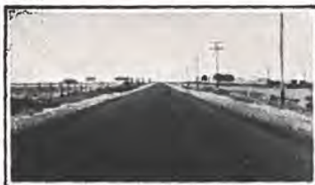
View of the improved highway between Alamosa and Monte Vista—another Midwest Asphaltic Road Oil "Mixed-in-Place" job.
