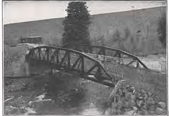
100 ft. Riveted Low Truss Span, Dillon, Colo.
