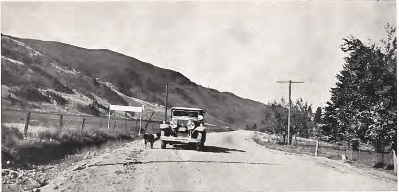
This fine stretch of gravel surfaced highway, located near Avon in Eagle County, was recently completed by the State Highway Department with Federal co-operation.
