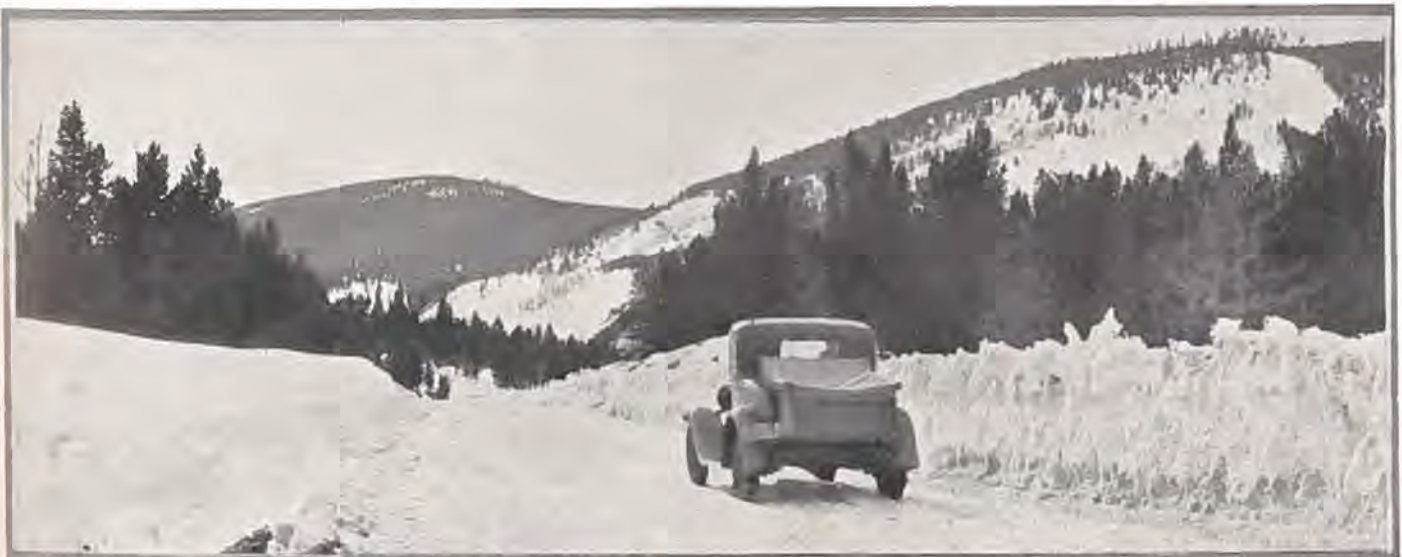
Showing a stretch of the highway over Tennessee Pass, over which traffic moves throughout the winter months. Except for a few hours after an unusually heavy snowstorm motorists have been able to travel this pass day and night. Snow-removal work is handled by state forces. Photo by George Toupain.
