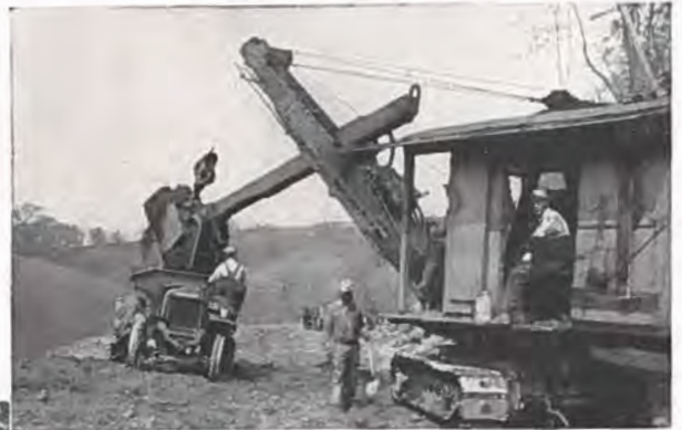
Above: McCormick-Deering Industrial Power is used to operate loading and hauling equipment in road construction work.
