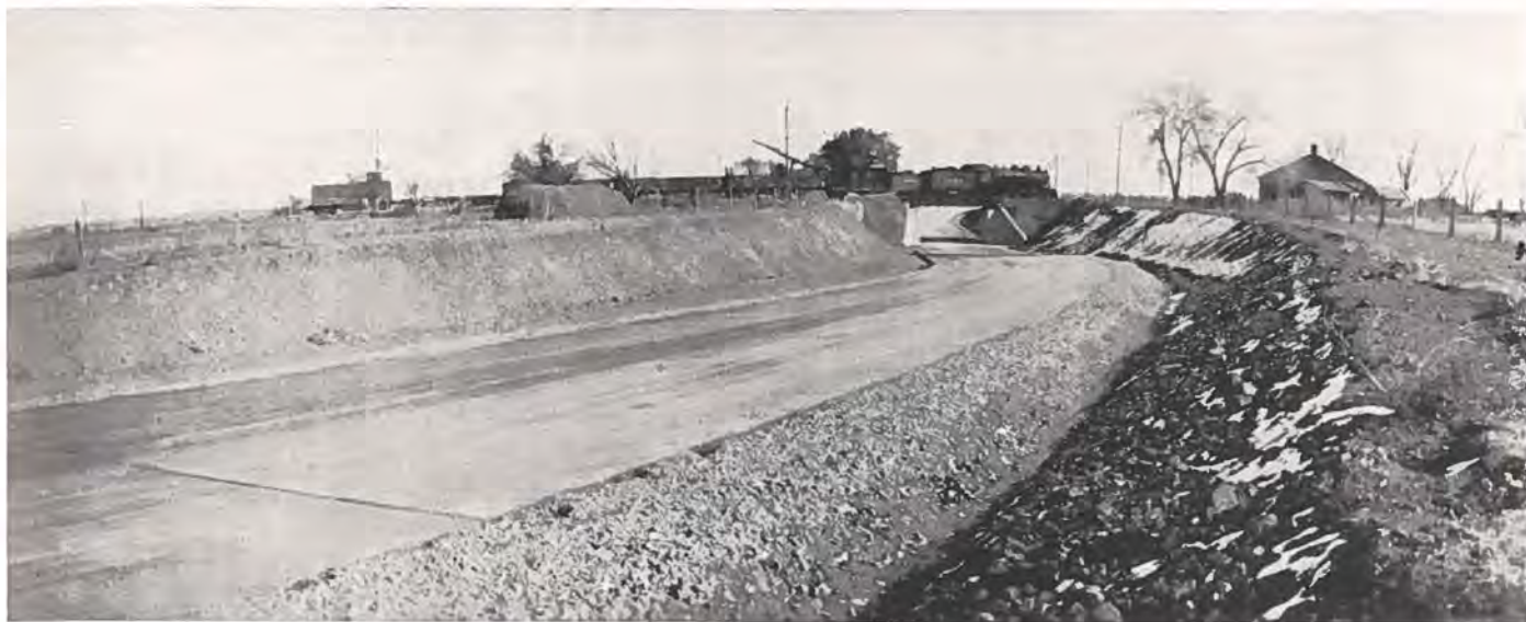
Concrete paved under-crossing near Manzanola, U. S. Route No. 50. Paving project built by Colorado State Highway Department with Federal co-operation.
