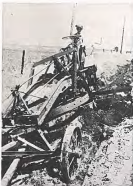
An Adams Leaning Wheel Grader in tough going on State Highway No. 8. Owned by the State Highway Department.
