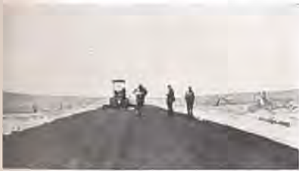
Colorado State Highway Engineers inspecting the Nunn-Wyoming State Line "Mixed-in-Place" highway. This road, made with Midwest (Standard) Asphalt Road Oil, has caused widespread and favorable comment.
