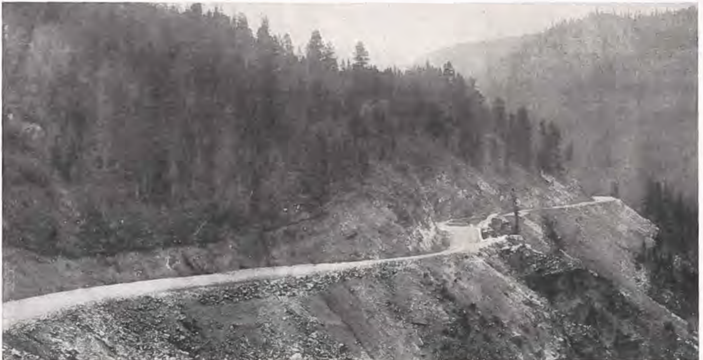
A view of the modern highway over the famous Battle Mountain near Redcliff.—Photo by H. L. Jenness.
