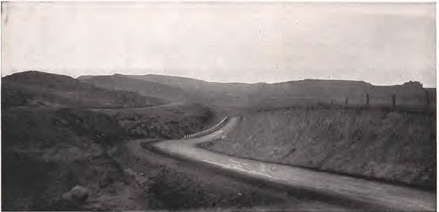
A stretch of oil-processed highway northeast of Fort Collins in Larimer County, near Virginia Dale, recently opened to motorists. This work was accomplished by state highway forces under the supervision of Engineer Clyde Walters.
