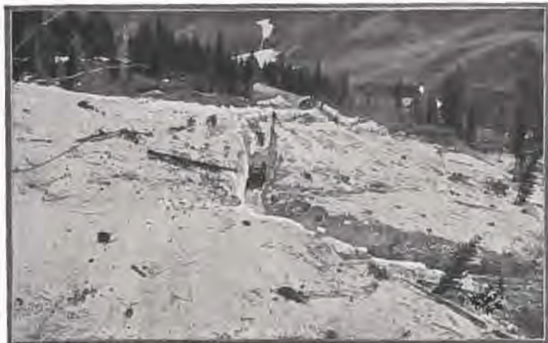
A snowslide—to be more exact—"Slippery Jim Slide," located between Ouray and Silverton on the Million Dollar Highway—just one of the many snow-fighting jobs for the state maintenance forces. Photo submitted by George Toupain.
