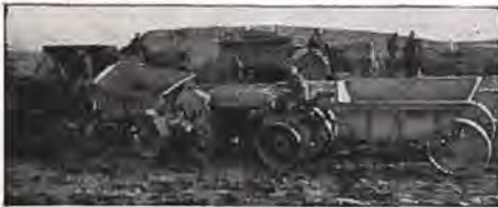
The St. Croix Construction Company, Stillwater, Minn., uses tractors with dump trailers. The wagons windrow and pack the dirt, leaving little work for graders and loaders.
