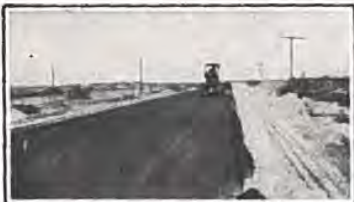
A delight to motorists—the "Mixed-in-Place" Road between Nunn and the Colorado-Wyoming state line, made with Midwest Asphaltic Road Oil.
