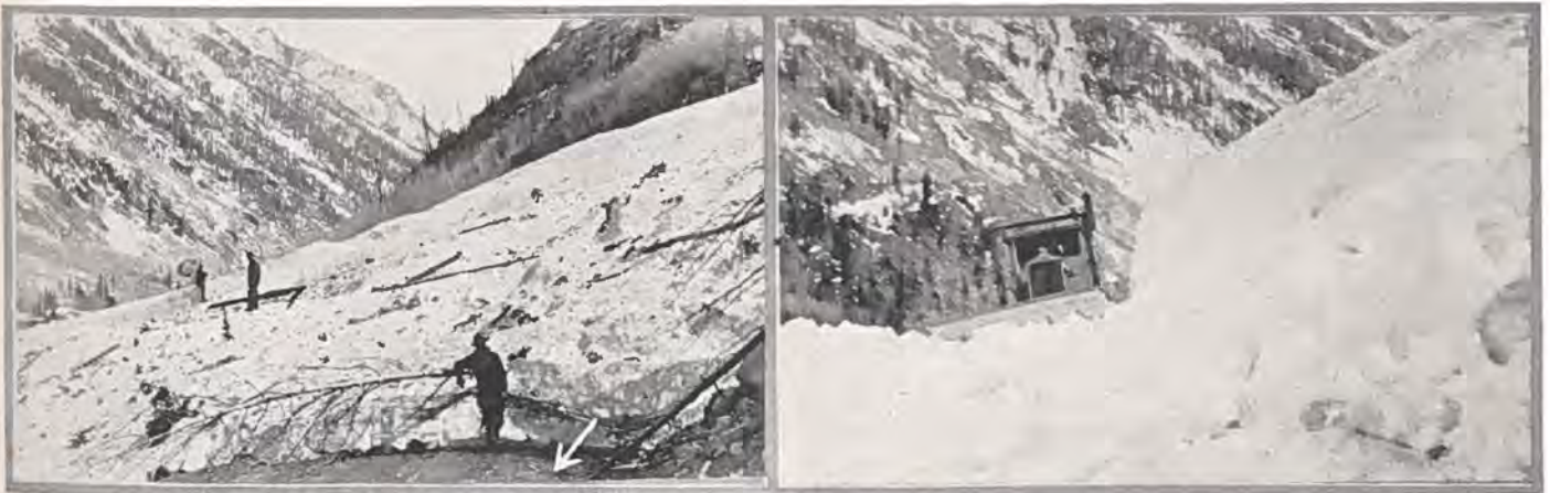
A snow-removal problem at Lime Creek Slide, between Durango and Silverton. Note roadway marked by arrow. Just fourteen feet of snow, that's all. Picture at the right shows snow plow in tough going. These pictures show one of the problems that state maintenance forces face throughout the winter months. Photos by D. Kirk Shaw.
