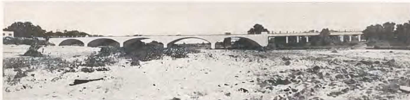
Concrete arch bridge over the Fountain River, near Pueblo, which forms a connection with State Road No. 96.
