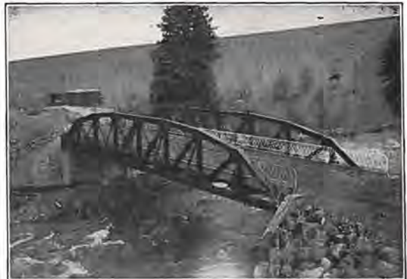
100 ft. Riveted Low Truss Span, Dillon, Colo.
