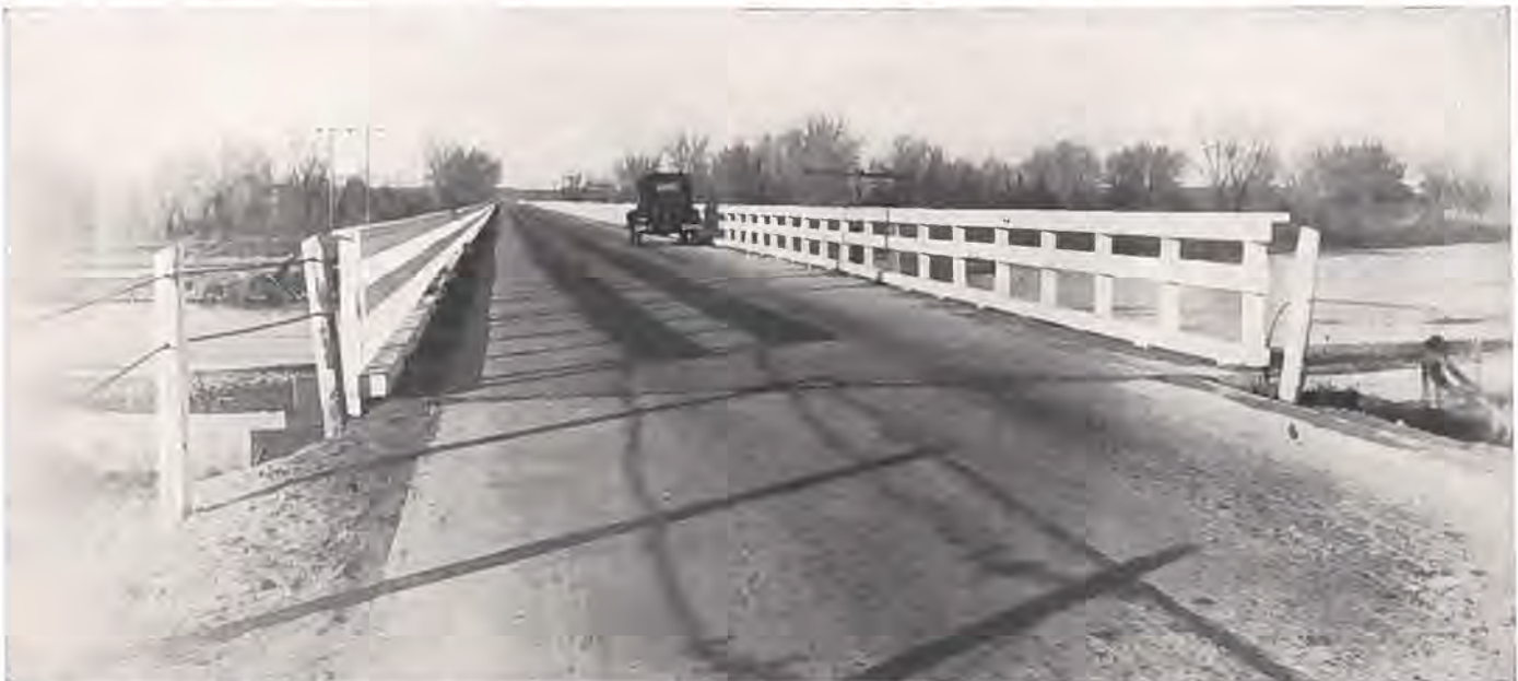
A section of the Sterling-Fort Morgan concrete highway, showing a bridge over the Platte River; pavement and bridge constructed with Federal Aid co-operation.
