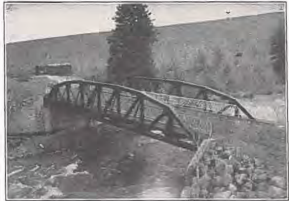
100 ft. Riveted Low Truss Span, Dillon, Colo.
