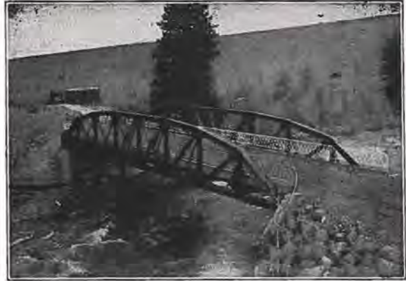
100 ft. Riveted Low Truss Span, Dillon, Colo.
