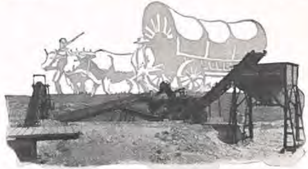
No. 12 Pioneer Screening, Crushing and Loading Plant in special hookup with Primary Breaker, operating in Texas. The Zempter Construction Company of Amarillo, Texas owns two Pioneer "setups" like this. On the left in above picture is 40' by 24' feeder conveyor leading up to a scalping screen and No. 1536 Universal Crusher, mounted on trucks. All oversize is reduced in Primary Breaker to 3 1/2-inch material, which goes over another conveyor to No. 12B Pioneer Plant, where it is screened, crushed to required size and delivered to 21-yard storage bin. The fines are screened out and carried to dump in conveyor.
