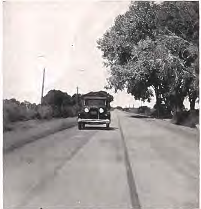
Another view of the new concrete pavement located east of Greeley. Seven and one-half miles of this standard pavement were recently opened to traffic. It extends east to Kersey from Greeley and provides a modern roadway through a rich dairy and agricultural section of Weld County.
