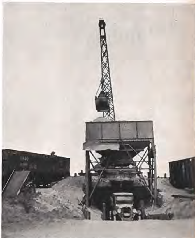
Central proportioning plant which enables contractor to speed up work.
