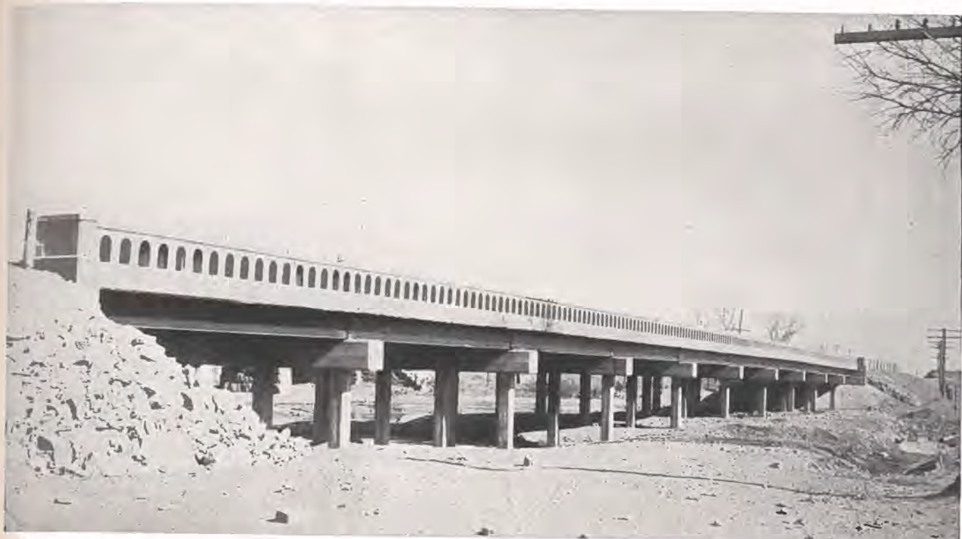
Newly completed Clay Creek concrete bridge, consisting of ten 30-foot spans, located about three miles east of Lamar in Prowers County. Photo by Paul Bailey, State Highway Bridge Engineer.
