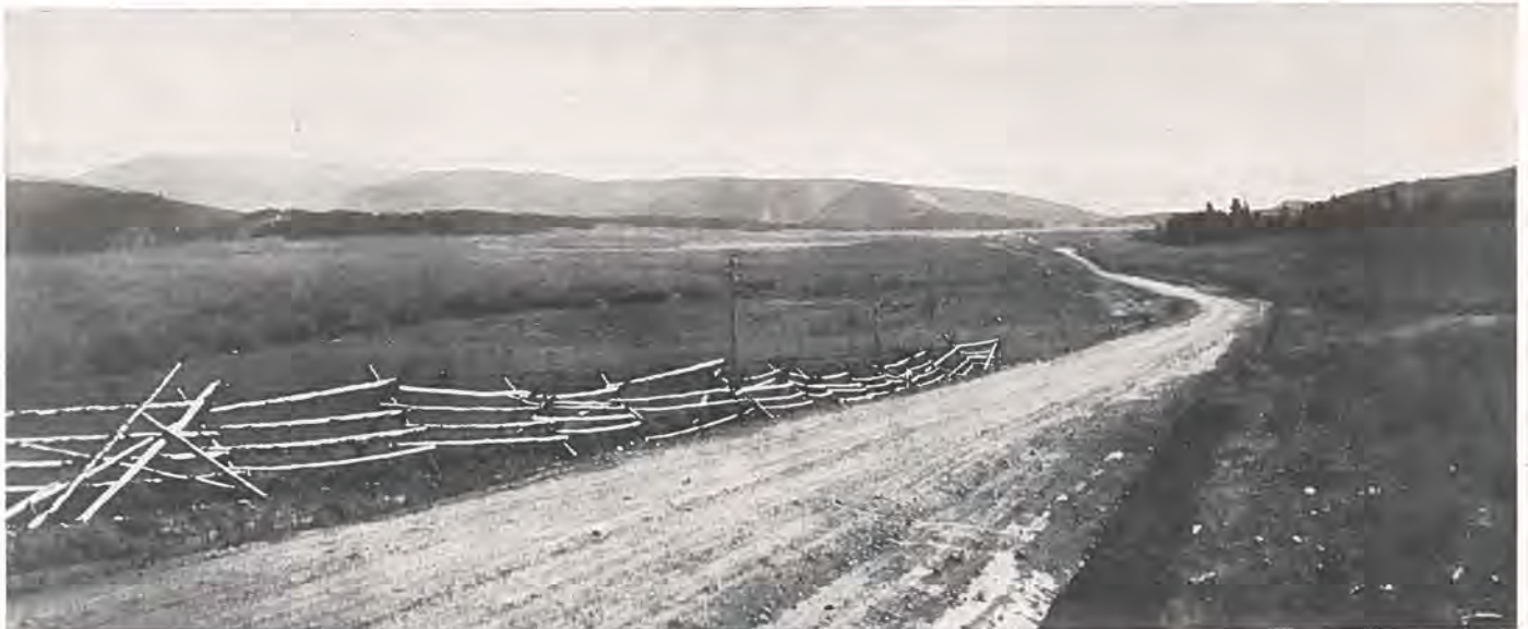
Section of newly constructed road between Granby and Grand Lake, forming a link in the Fall River circle trip from Denver.
