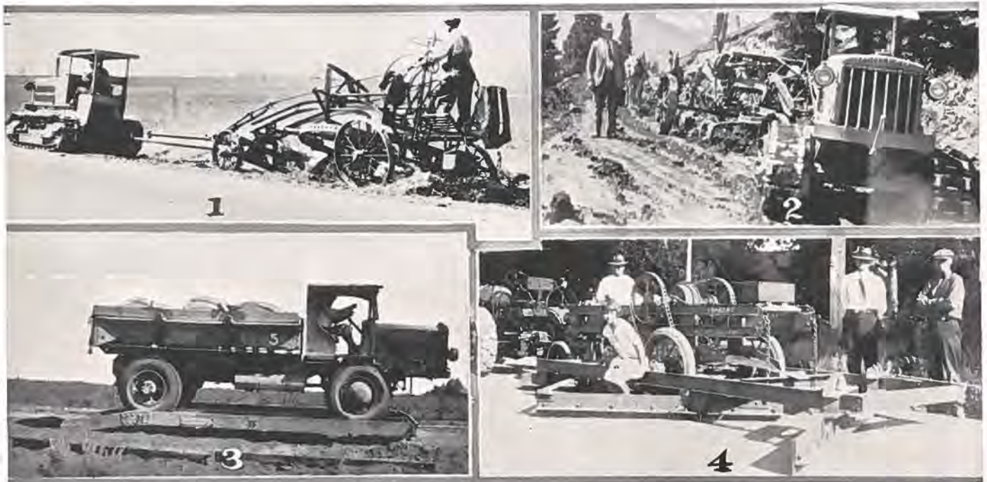
1. Here's an Adams Leaning Wheel Grader on "shoulder" work west of Denver. Picture by Elton T. Fair Company. 2. This picture submitted by the Wilson Machinery Company shows a Monarch "50," in close quarters near Creede. 3. A Coleman "four-wheel-drive" truck on turntable hauling cement for one of Edw. Selander's contracts. 4. Up in Larimer County they go in for modern maintenance equipment. Here's a Baker maintainer with a McCormick-Deering tractor. Photo, H. W. Moore Equipment Co.
