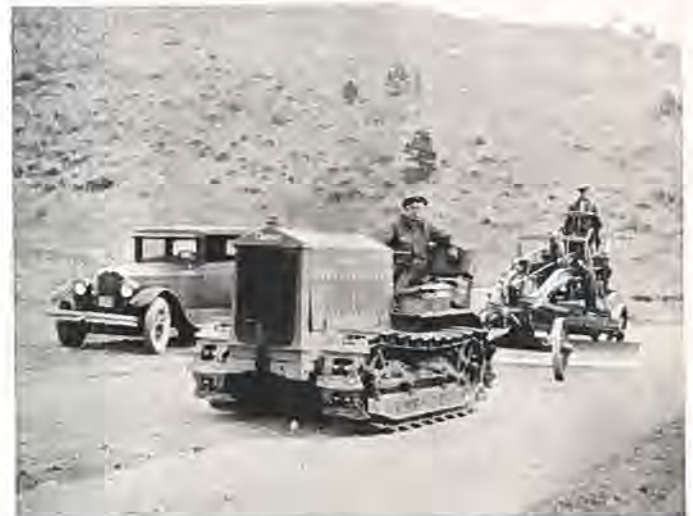
One of the state's maintenance crews working on Vernon Canon route—recently oil surfaced.
