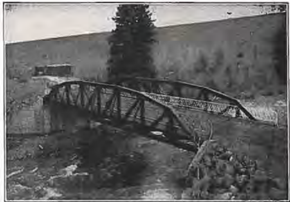
100 ft. Riveted Low Truss Span, Dillon, Colo.
