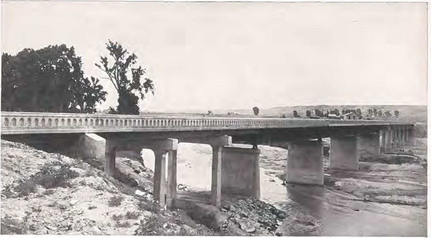
Picture of the new steel and concrete bridge constructed by the state highway department with Federal co-operation over the Fountain River near the town of that name in El Paso County, forming a link in the new concrete pavement now under construction between Colorado Springs and Pueblo. It will soon be open to traffic.
