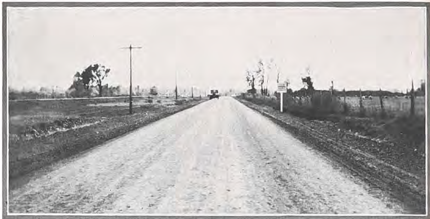
Type of mixed-in-place oil road being constructed in Colorado.
