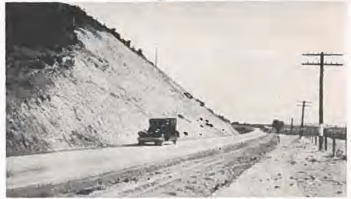
The side of a mountain was cut away to make room for this paved road near Sedalia.
