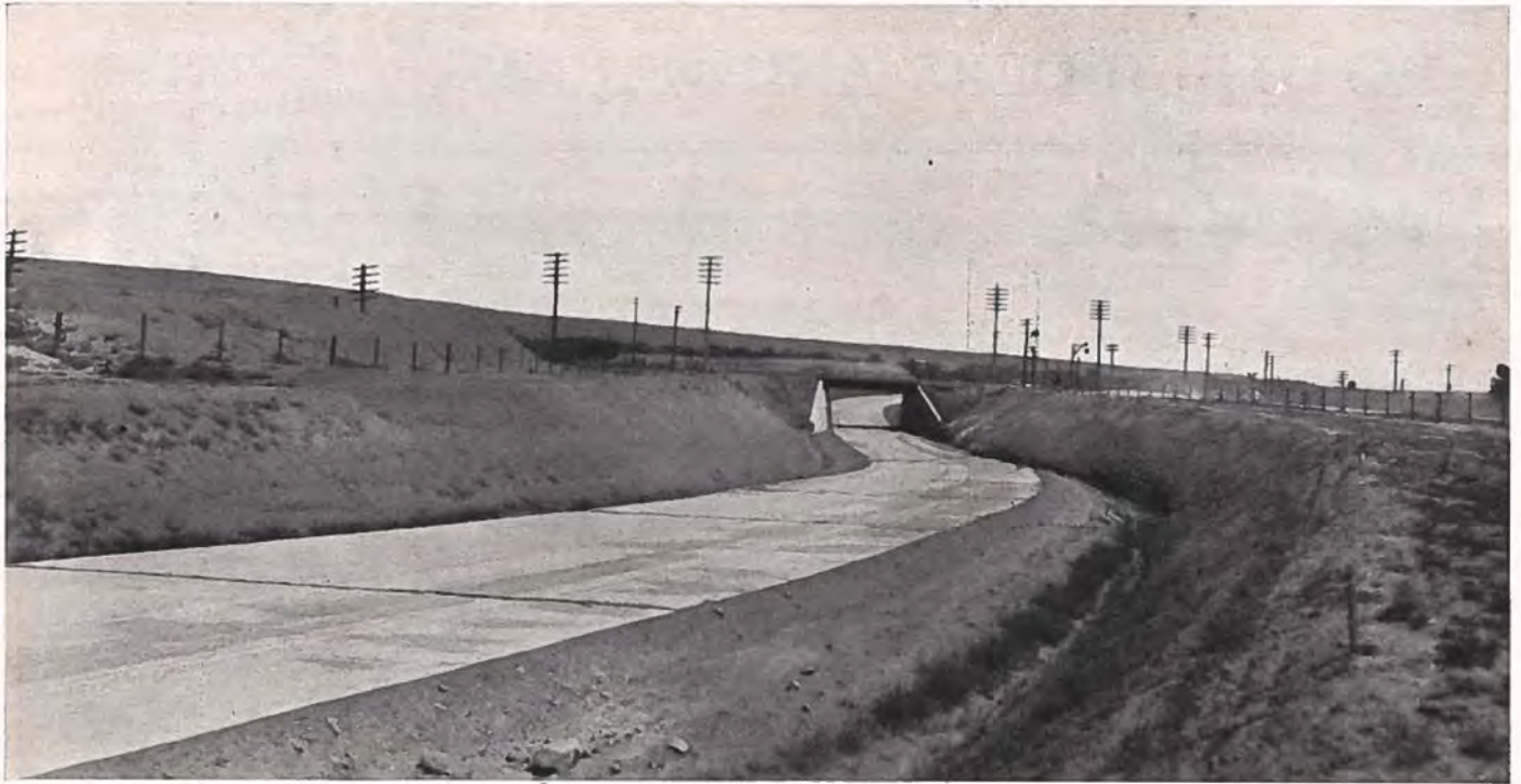
Concrete-paved underpass, eliminating grade crossing at Bragdon, Colorado Springs-Pueblo highway. Ideal Portland Cement used exclusively.
