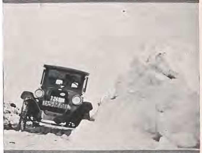
"Uncle Sam must go through, rain or shine." Here we have the mail truck "surrounded" by snow east of Fairplay on Red Hill, during the month of January. Yes, it got through by the help of state crews.
