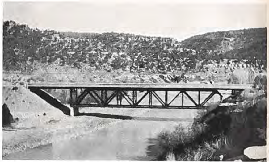
Looking downstream at Animas River bridge, located near Bondad, on highway between Durango and Farmington, New Mexico. This beautiful structure was recently completed by the state with Federal co-operation. Photo by J. R. Cheney.
