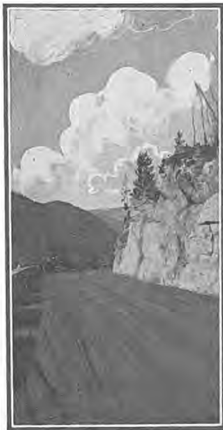
Showing a section of the Independence Pass highway, now open to traffic—the highest pass road in Colorado.
