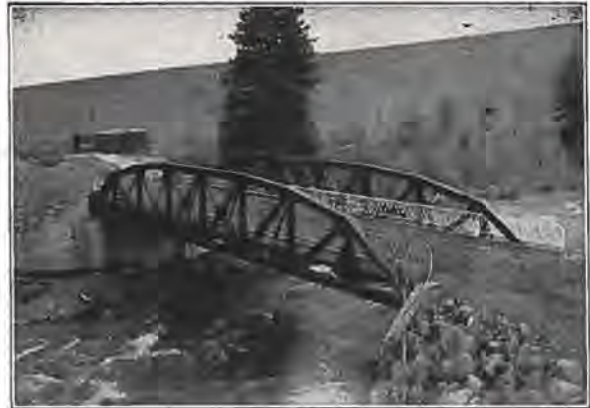
100 ft. Riveted Low Truss Span, Dillon, Colo.
