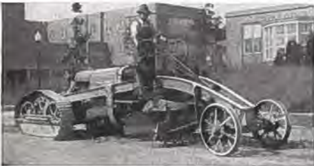
This McCormick-Deering-powered grader and scarifier is favorite equipment for street and road work
