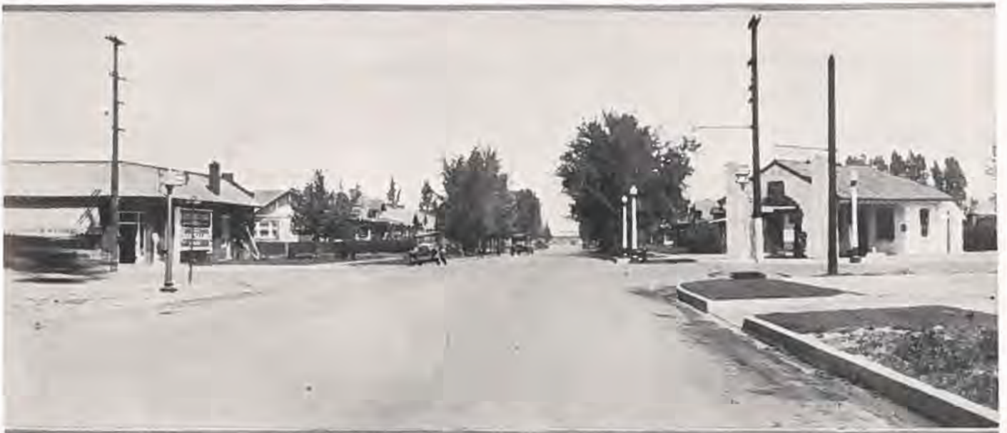
A scene on York Street in Denver which was treated with the "mat" method of oil processing by highway forces of the City and County of Denver. This street carries an average of 4,000 vehicles per day.
