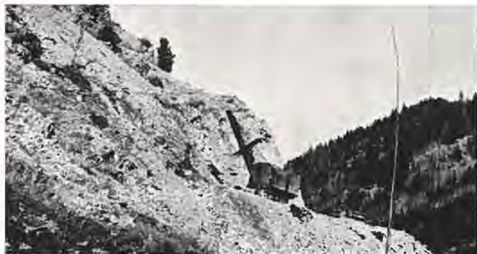
Tearing away 100,000 yards of rock on a new road over Kenosha Pass in Park County.
