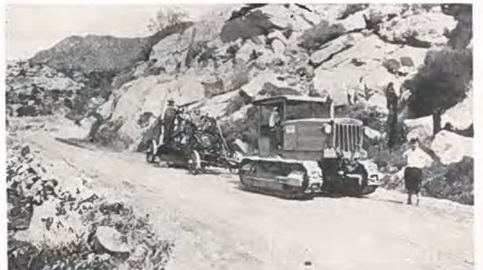
A state highway maintenance patrol near Texas Creek in Fremont County.
