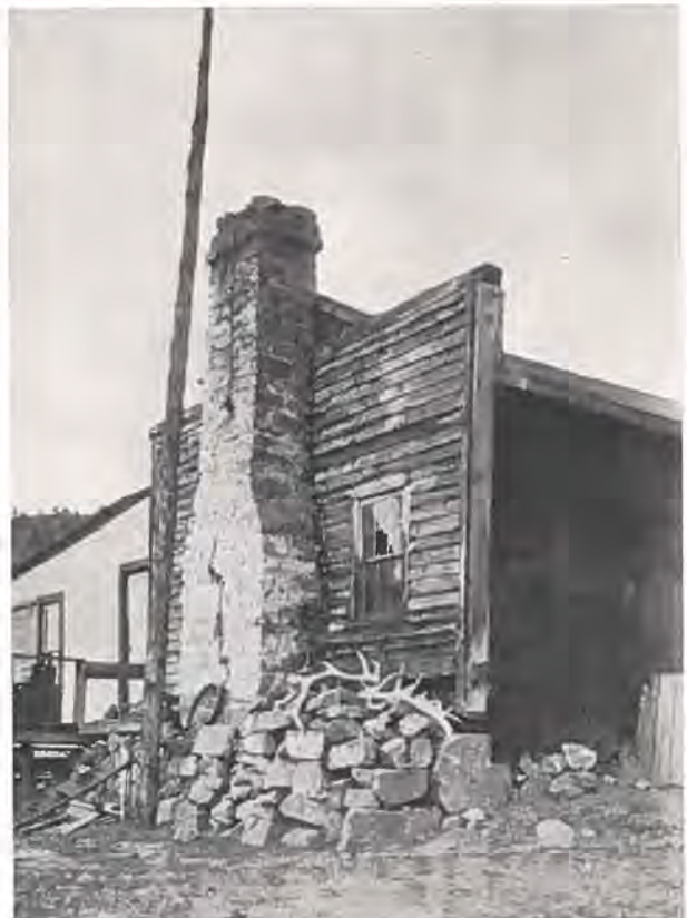
Showing original building and chimney constructed by Slade.
