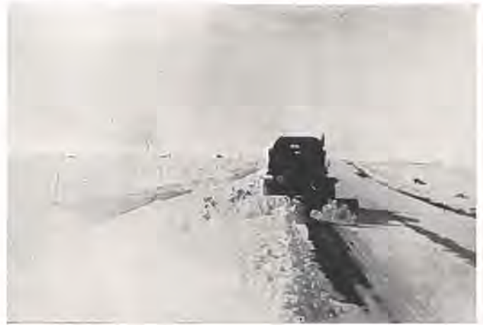
Showing how snow-removal is handled in Eastern Colorado—picture on the left shows a tractor and pull-grader working east of Sterling, and the one on the right is a truck with plow removing snow from the oil pavement north of Nunn. Photos by John Stamm.
