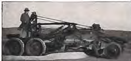
McCormick-Deering-operated road grader. Scores of types of road construction equipment are powered by McCormick-Deering.
