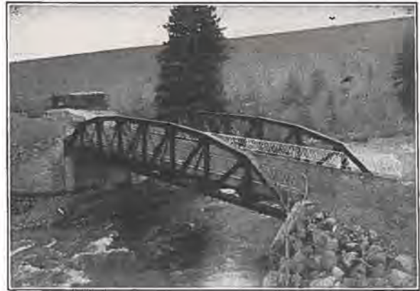
100 ft. Riveted Low Truss Span, Dillon, Colo.
