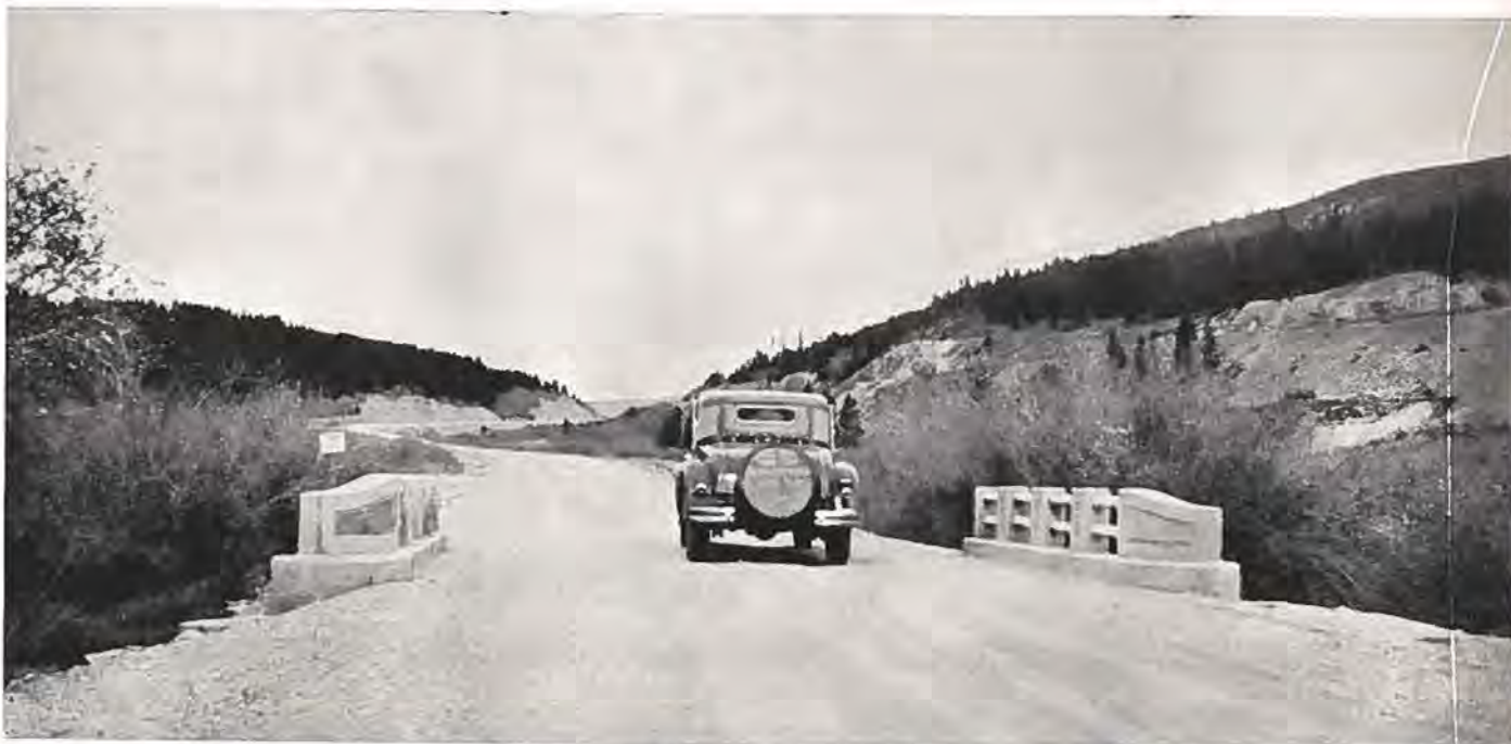
Showing a stretch of gravel surfacing on Tennessee Pass recently completed, giving a fine, wide, smooth highway from Leadville to Red Cliff. Photo by Joseph Roma.
