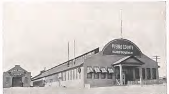
New highway shops recently purchased and fitted up by Pueblo County, for maintenance and repair of all road equipment owned by the county.
