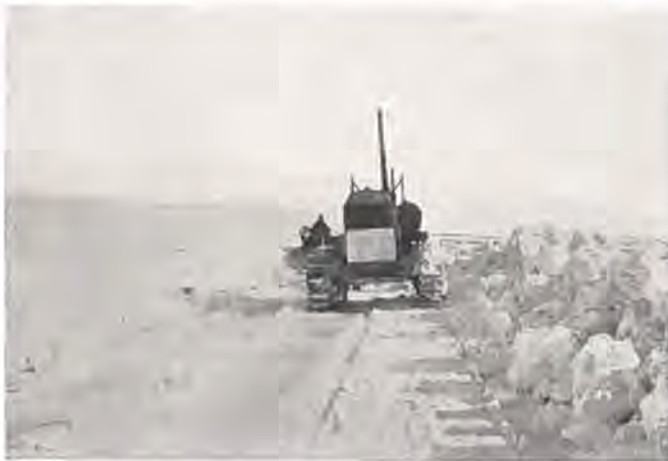
Showing how snow-removal is handled in Eastern Colorado—picture on the left shows a tractor and pull-grader working east of Sterling, and the one on the right is a truck with plow removing snow from the oil pavement north of Nunn. Photos by John Stamm.
