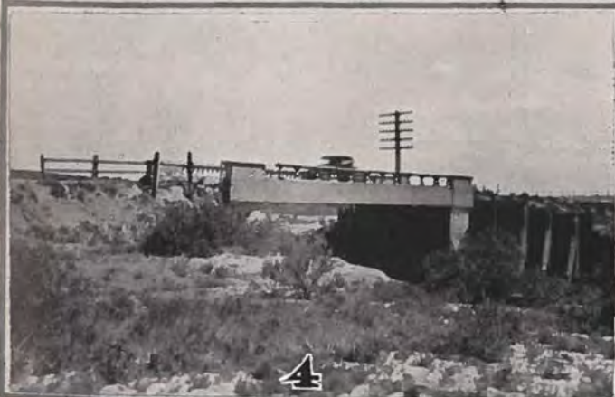
BEFORE AND AFTER , might well be the title to this group of photos showing old and new bridges on the new road between Colorado Springs and Pueblo. The new bridges form a part of the concrete pavement now being laid between the two cities. They run from 100 to 200 feet in length, and are 20 feet in width, being constructed of steel and reinforced concrete. These improvements were made by the State Highway Department in co-operation with the Federal government. M. E. Carlson was the contractor. Photos by M. W. Bennett.
