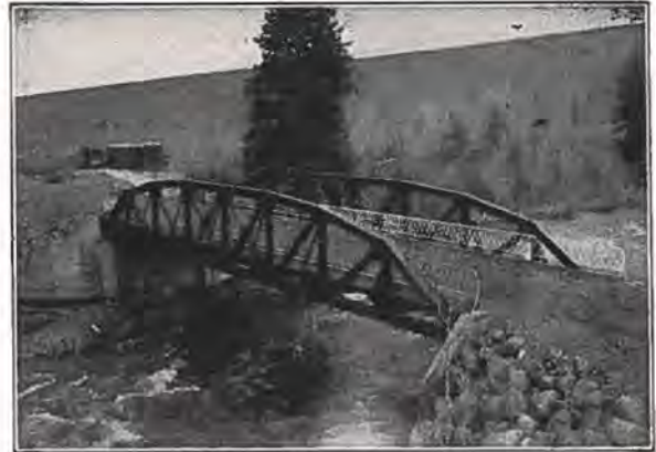
100 ft. Riveted Low Truss Span, Dillon, Colo.
