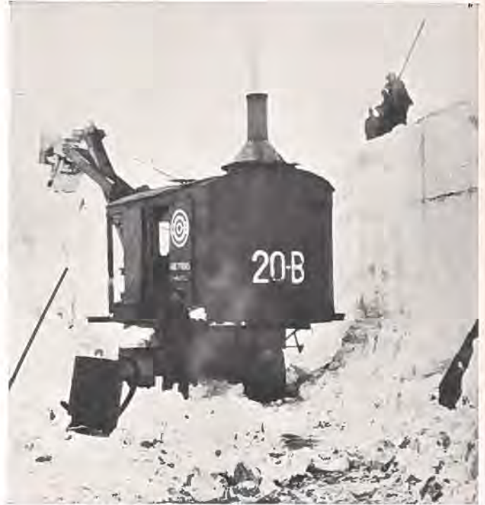
Showing how snow was removed from Milner Pass, located between Estes Park and Grand Lake. Snow twenty-five feet in depth was encountered in places. The work was done by the forces of the Rocky Mountain National Park.
