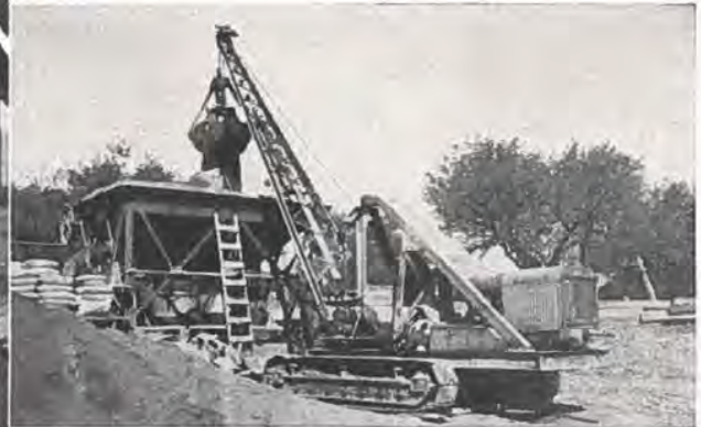
One of the many applications of the McCormick-Deering Industrial Power Plant is shown above where it is operating a derrick shovel on a big road project.
