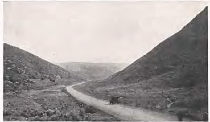
A fine piece of Federal Aid gravel roadway north of Meeker on Road No. 13.—Photo by H. L. Jenness.
