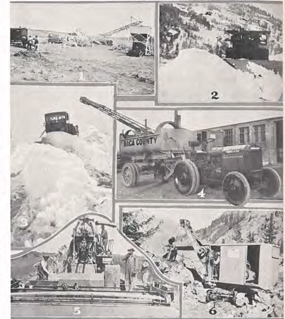
1. Crushing and screening rock for a state road near Lamar with a Cedar Rapids one-piece outfit. Photo by Hamilton & Gleason, contractors. 2. Bucking snow with a Cletrac north of Durango. Photo by Liberty Trucks & Parts Co. 3. A FWD truck clearing snow in Washington County. 4. One of Baca County's maintenance units—a McCormick-Deering industrial tractor and gravel trailer. 5. Ord concrete finisher working on pavement west of Ft. Morgan. Edw. Selander, contractor. 6. A General excavator in heavy rock on one of Winterburn & Lumsden's jobs near Grand Junction.
