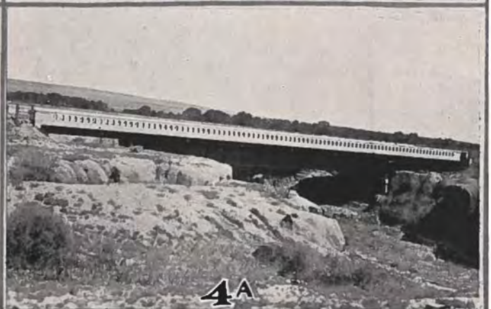
BEFORE AND AFTER , might well be the title to this group of photos showing old and new bridges on the new road between Colorado Springs and Pueblo. The new bridges form a part of the concrete pavement now being laid between the two cities. They run from 100 to 200 feet in length, and are 20 feet in width, being constructed of steel and reinforced concrete. These improvements were made by the State Highway Department in co-operation with the Federal government. M. E. Carlson was the contractor. Photos by M. W. Bennett.
