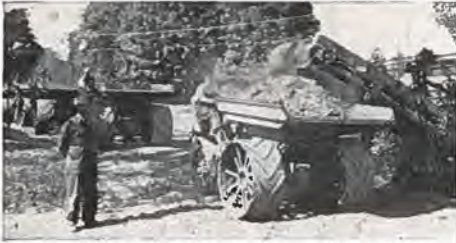
A fleet of McCormick-Deering-powered dump bodies moving dirt on a road construction job in Illinois
