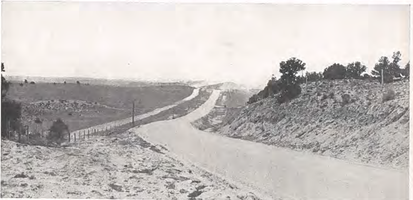
Showing new and old gravel surfaced highway east of Florence in Fremont County. A contract was recently awarded for the oil surfacing of this road. It was constructed with federal co-operation.
