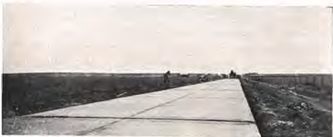
Showing finished concrete pavement before gravel shoulders have been laid.
