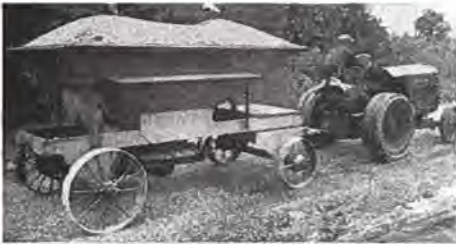
The Street Department of Philadelphia operates this chip spreader with a McCormick-Deering Industrial Tractor on new macadam road work
