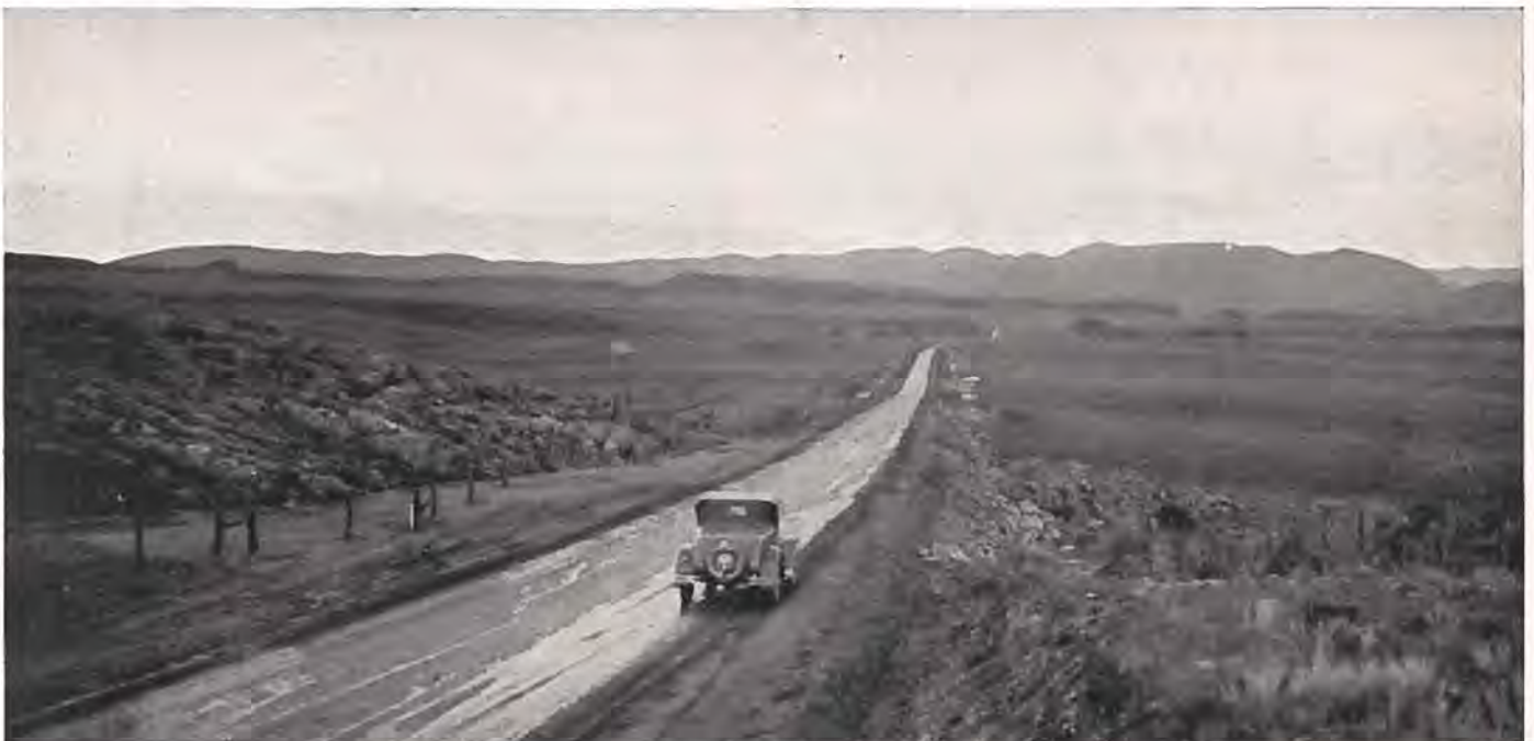
Showing section of new oil-processed highway northeast of Fort Collins recently opened for traffic.
