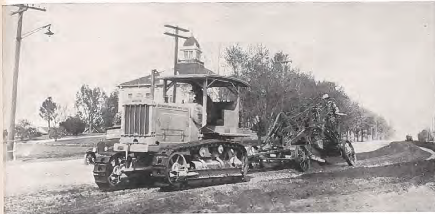
One of the State Highway Department's oil processing crews at work on four miles of oil processed roadway located between Englewood and Littleton. Arapahoe County courthouse in background. Photo by M. W. Bennett.
