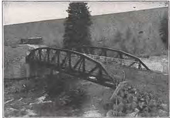
100 ft. Riveted Low Truss Span, Dillon, Colo.
