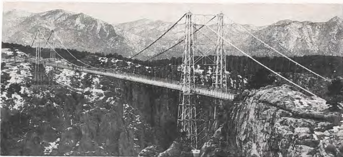
Newly constructed scenic highway bridge over the Royal Gorge near Canon City.
