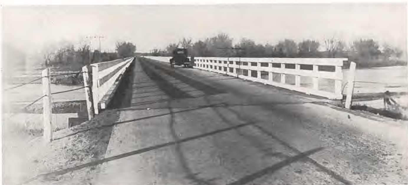
A 1,000 foot bridge across the Platte River near Moreno, on the Fort Morgan-Sterling paved highway, constructed by the State Highway Department.
