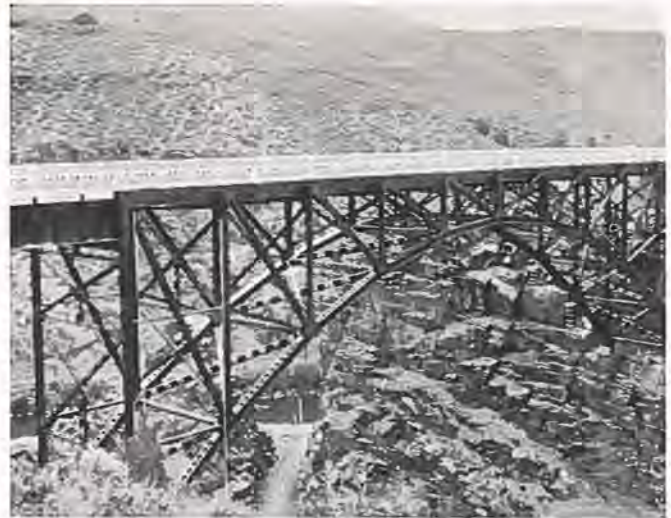
Sapinero arch bridge over the Lake Fork of the Gunnison River, one of the highest bridges in the West, constructed by the State Highway Department in co-operation with the U. S. Bureau of Roads. A big thrill to motorists.
