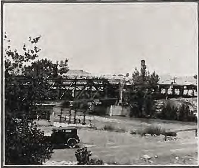
Showing newly constructed steel and concrete bridge over Arkansas River near the town of Portland.
