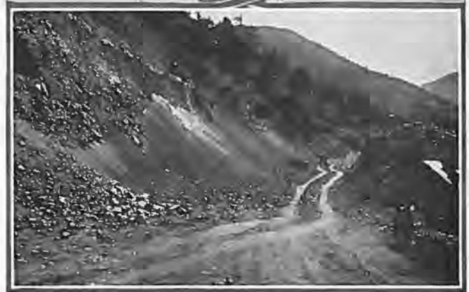
Upper—Reinforced Concrete Cribbing on Federal Aid Project 145. Lower—Showing Heavy Excavation Above Railroad Tracks
