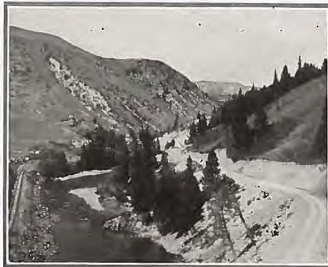
Byers Canon, located between Hot Sulphur Springs and Parshall. Completion of this costly piece of work eliminates the worst grade on the Victory Highway in Colorado.
