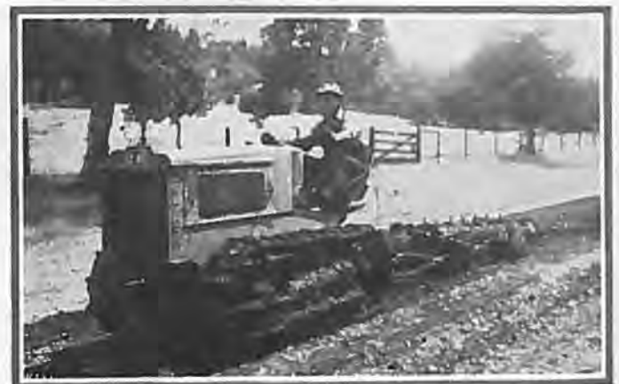
Harrowing oil into surface
