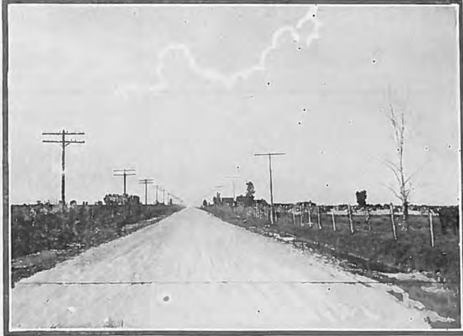
A Section of Gravel Surfaced Roadway in Eastern Colorado, Near Wray
