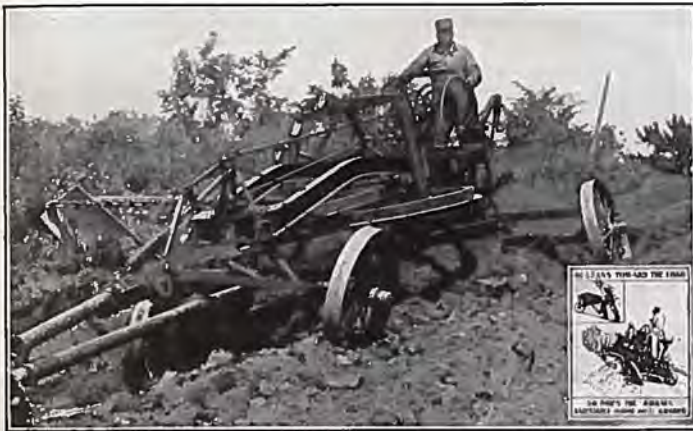
Adams 10-ft. grader finishing a ditch bank by making a heavy cut with the Back Sloper. Front wheels leaned to offset side pull of Back Sloper. Rear wheels leaned to hold machine against heavy cut.
