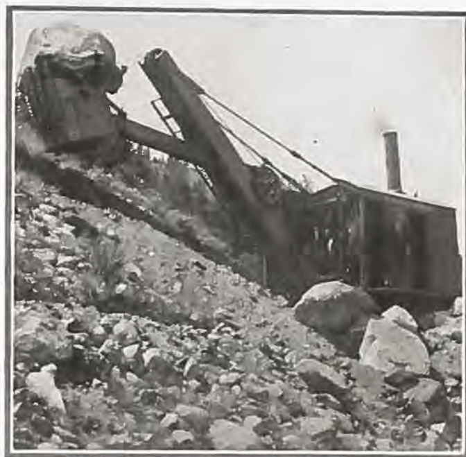
Showing steam shovel "eatin' up the earth"—a "he man" road building job—located in Chaffee county, north of Buena Vista.
