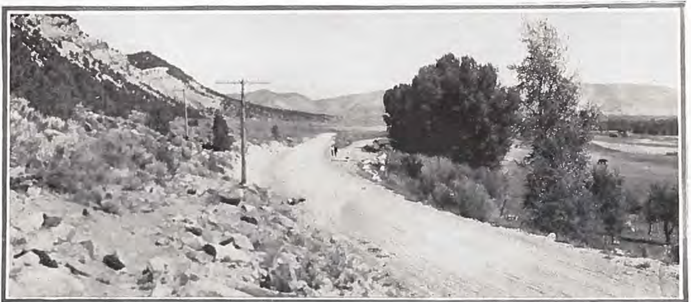
Completed Federal Aid Project located near Carbondale on State Road No. 82.
