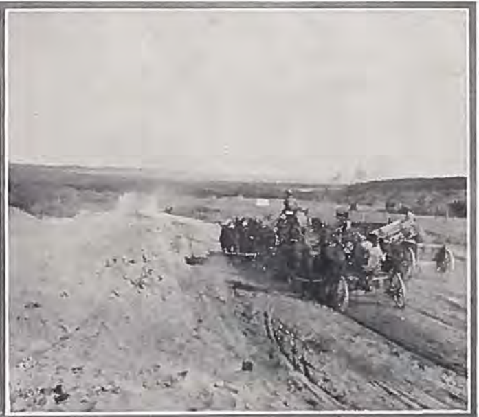
Two elevating grader outfits "moving dirt" on 10-mile project near Palmer Lake on Denver-Colorado Springs Highway.
