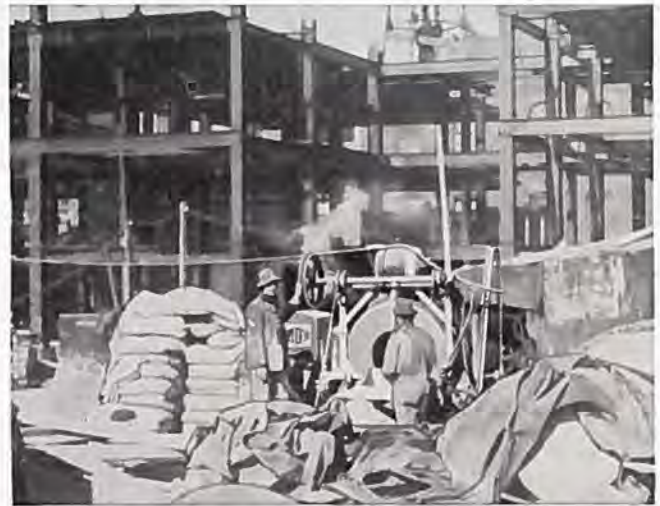
One of the Smith 7-S (One Bag) Mixers used in the construction of Tudor City by the Fred F. French Company, New York. This new housing development is in the heart of New York City between 40th and 43rd Sts., east of Second Ave. The French Co. demolished three square blocks of tenements to erect these safe, modern buildings.
