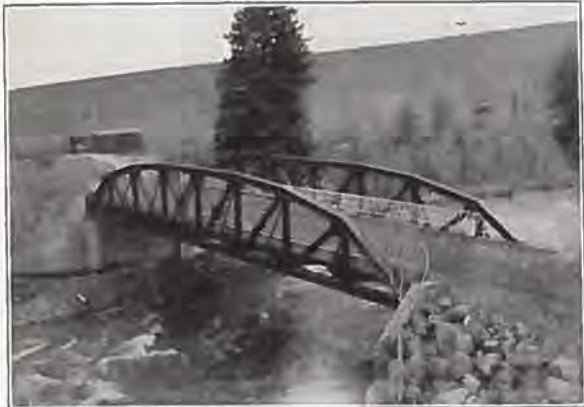
100 ft. Riveted Low Truss Span, Dillon, Colo.
