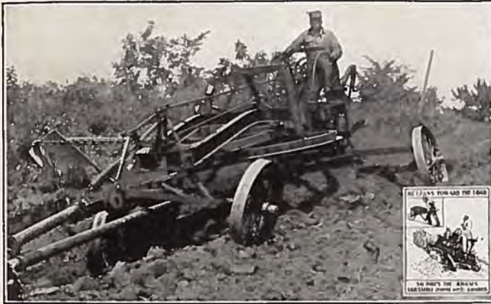
Adams 10-ft. grader finishing a ditch bank by making a heavy cut with the Back Sloper. Front wheels leaned to offset side pull of Back Sloper. Rear wheels leaned to hold machine against heavy cut.
