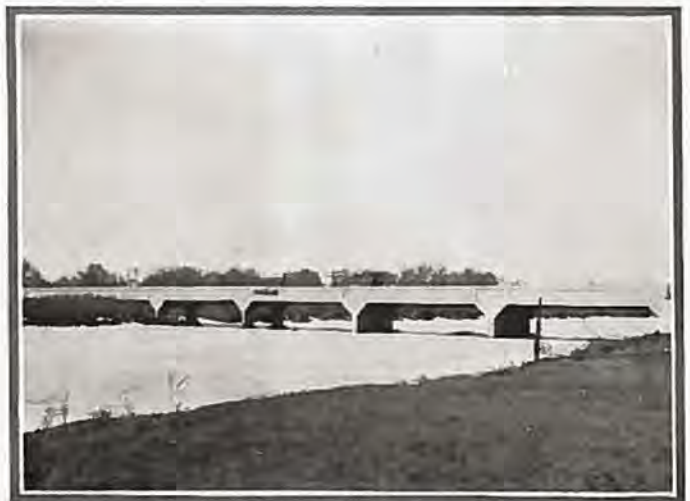
View of 6-span State Highway concrete bridge over Rio Grande Del Norte River near Alamosa.
