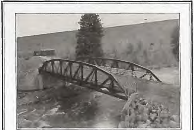
100 ft. Riveted Low Truss Span, Dillon, Colo.
