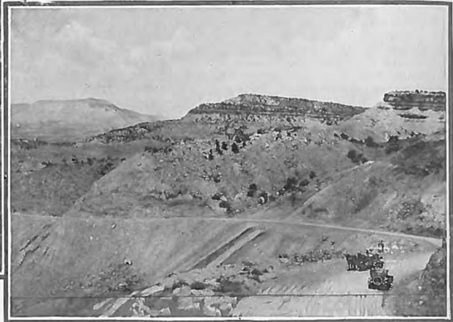
A Mountain of Oil Shale, with Heavy Side-hill Excavation, Near De Beque
