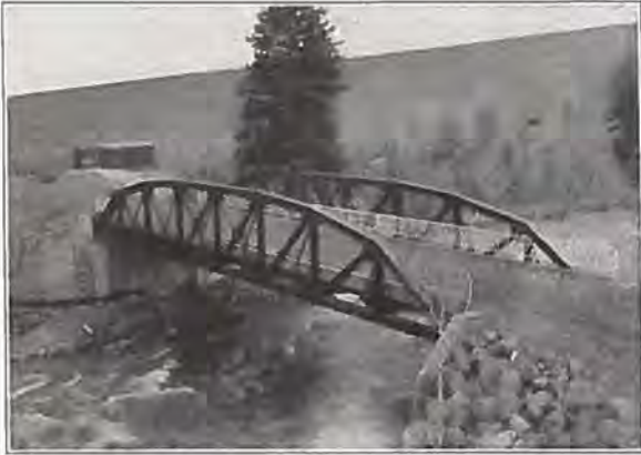
100 ft. Riveted Low Truss Span, Dillon, Colo.
