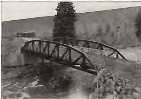
100 ft. Riveted Low Truss Span, Dillon, Colo.
