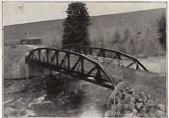
100 ft. Riveted Low Truss Span, Dillon, Colo.
