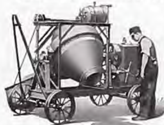
Smith 7-8 Tilting Mixer with power loader. One bag batch capacity up to 1-3-6 proportions. Easy control of discharge.
