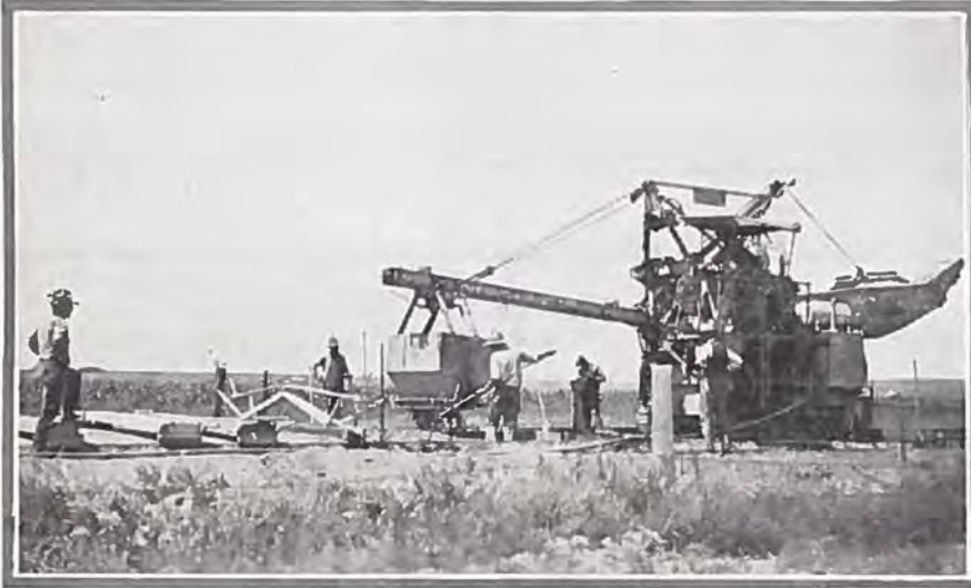
Two Views Showing Construction of Pavement North of Colorado Springs With Gold Ore.
