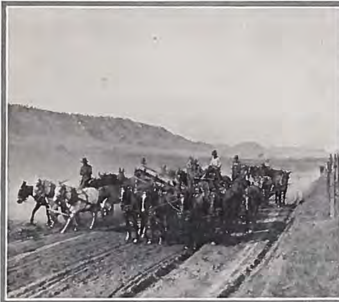
Two elevating grader outfits "moving dirt" on 10-mile project near Palmer Lake on Denver-Colorado Springs Highway.
