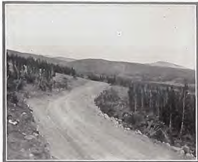
Typical side-hill section, looking north, showing broad, smooth gravel surface.
