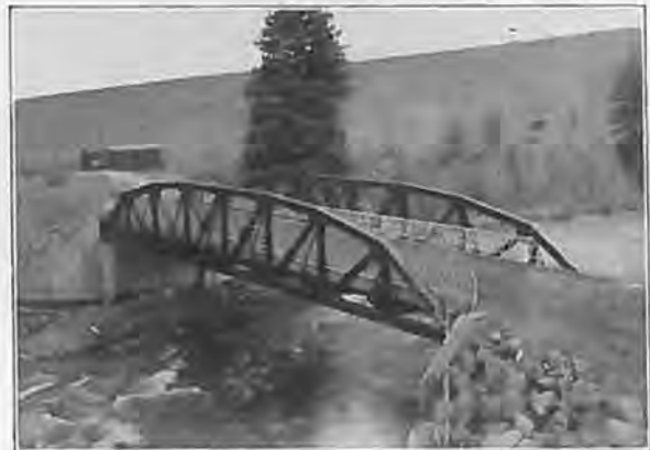
100 ft. Riveted Low Truss Span, Dillon, Colo.
