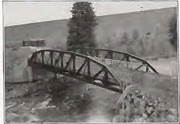
100 ft. Riveted Low Truss Span, Dillon, Colo.
