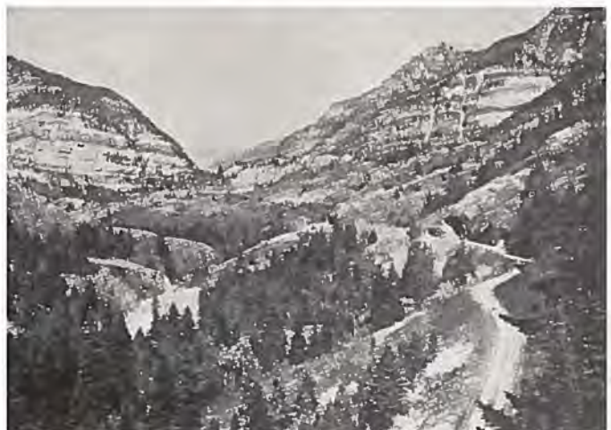
Section of Ouray-Silverton Highway, near the town of Ouray.
