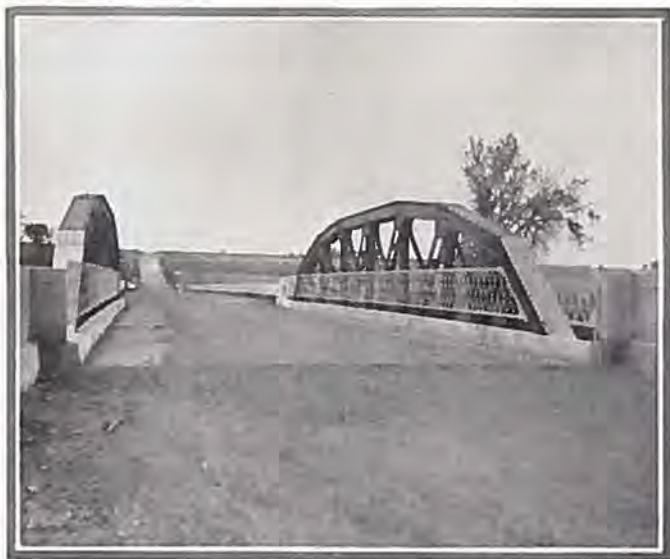
A section of the new Lafayette-Longmont road, showing 100-ft. steel bridge over Boulder Creek.
