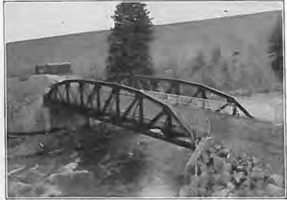
100 ft. Riveted Low Truss Span, Dillon, Colo.
