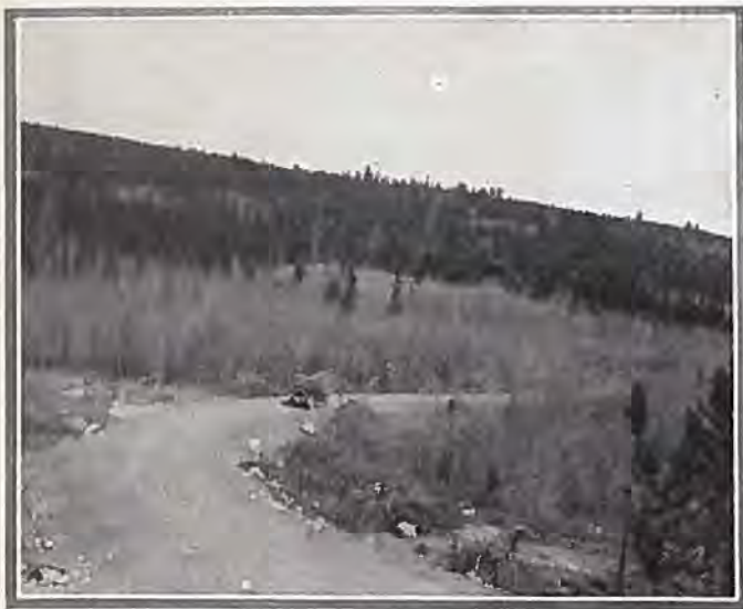
Where the Maxwell Highway was built through a swamp, near junction with old road.
