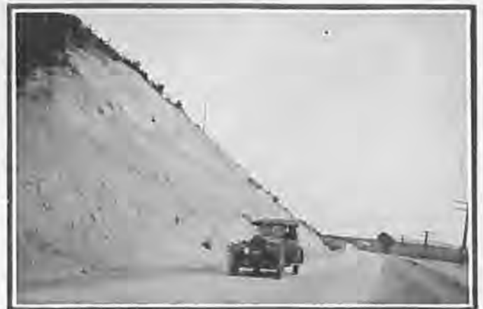
View of heavy side-hill cut on Denver-Colorado Springs road
