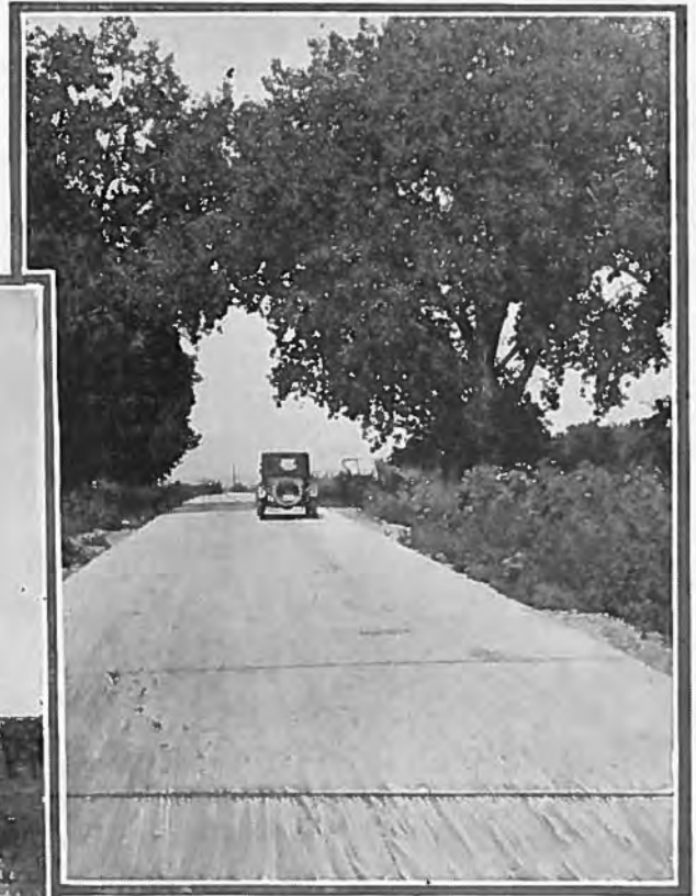
View of Concrete Pavement on U. S. Highway No. 285, Near Loveland
