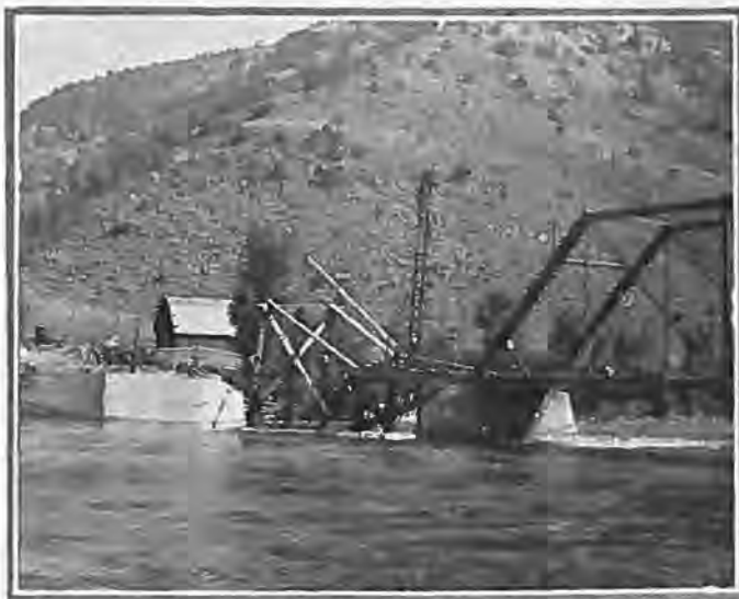
View of state maintenance crew making temporary repairs on bridge destroyed by June flood near State Bridge, in Eagle County.
