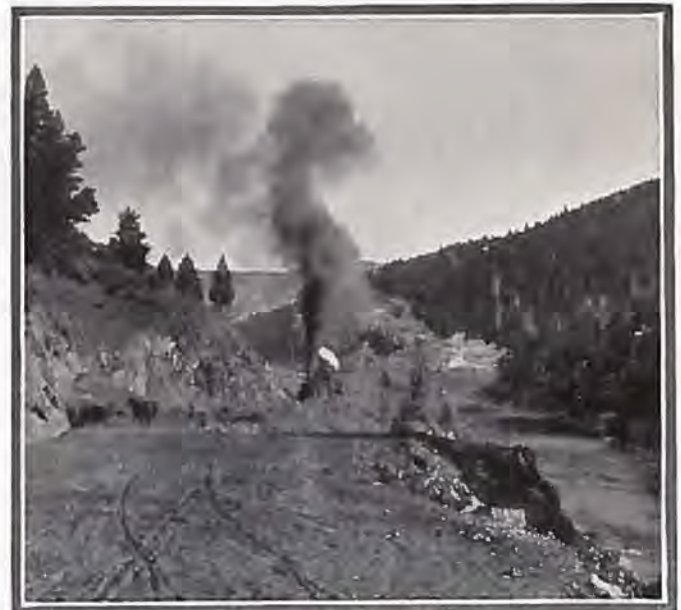
Steam Shovel Working on New Road at the West End of Byers Canon—Federal Aid Project
