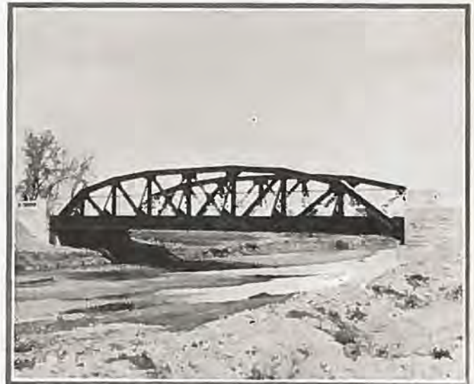
New steel and concrete bridge which spans Boulder Creek, on stretch of newly graded road, which is now in course of paving, located north of Lafayette.
