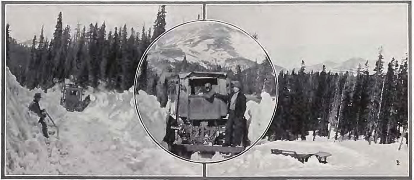
Showing how road over Hoosier Pass was cleared of snow with aid of heavy tractors and V-plows.
