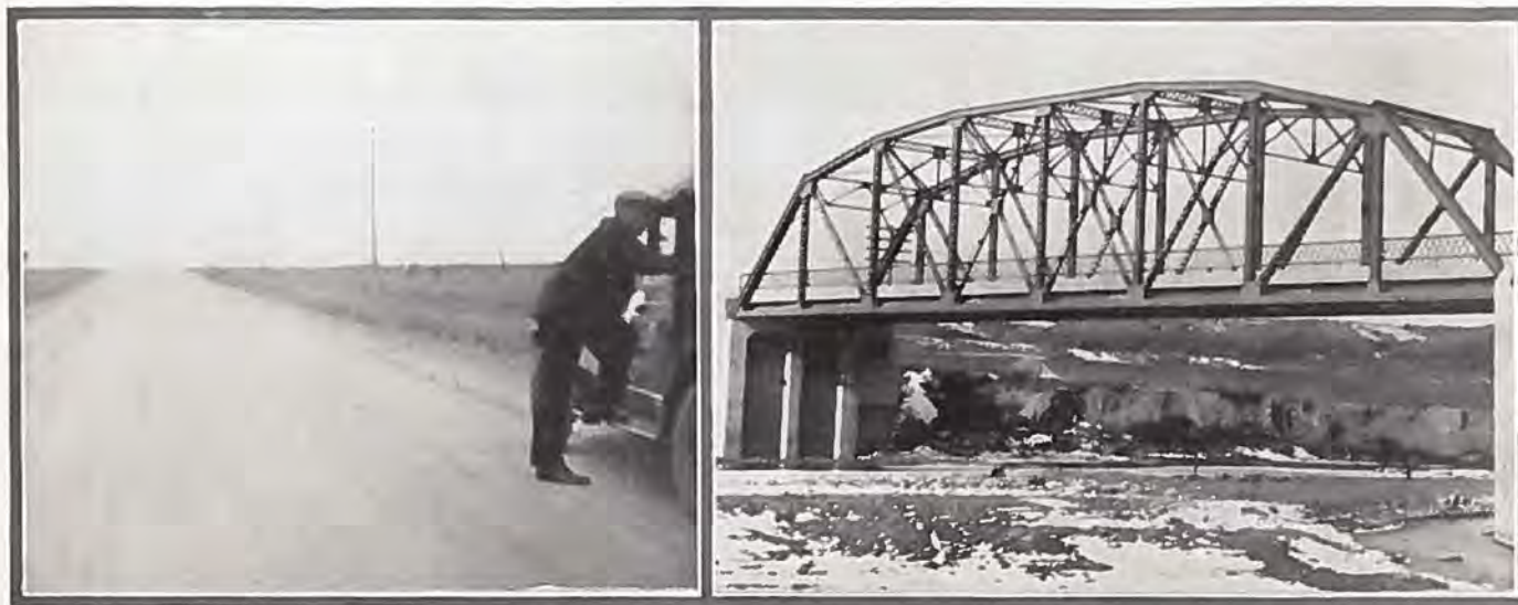
A Fine Stretch of Gravel Surfacing on Santa Fe Trail, Located East of Pueblo—on Right, New Steel and Concrete Bridge Over the St. Charles River, Constructed by the State Highway Department with Federal Aid Funds.
