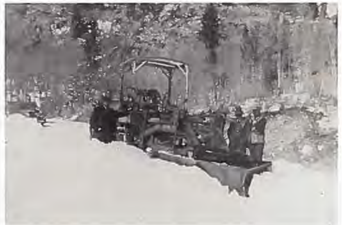
Clearing snow from the Berthoud Pass road near Empire in Clear Creek county—using one-man outfit.
