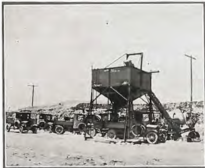
Fremont county's new portable gravel crushing plant—showing set-up between Florence and Canon City.
