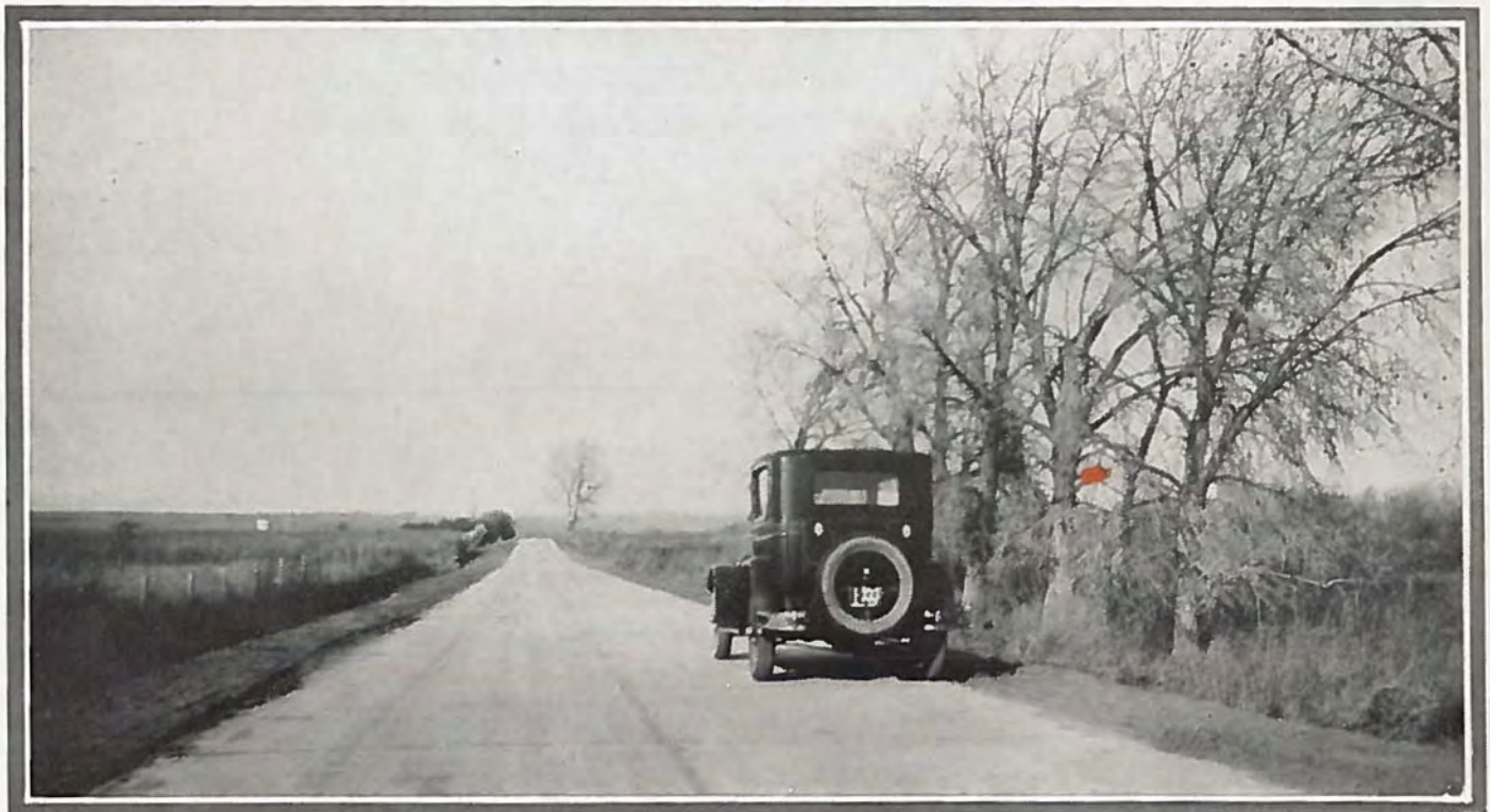
Scene along newly laid concrete pavement north of Lafayette in Boulder county
