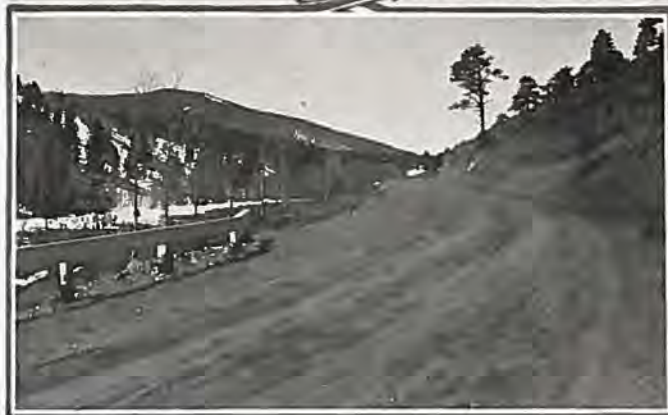
Upper—Shows Completed Road Through Fern Cliff Lower—Section of New Road Near Allens Park
