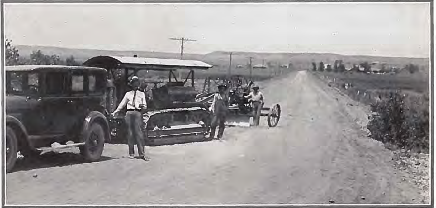
A graded earth section of state road in Crowley County, completed by county maintenance crew.
