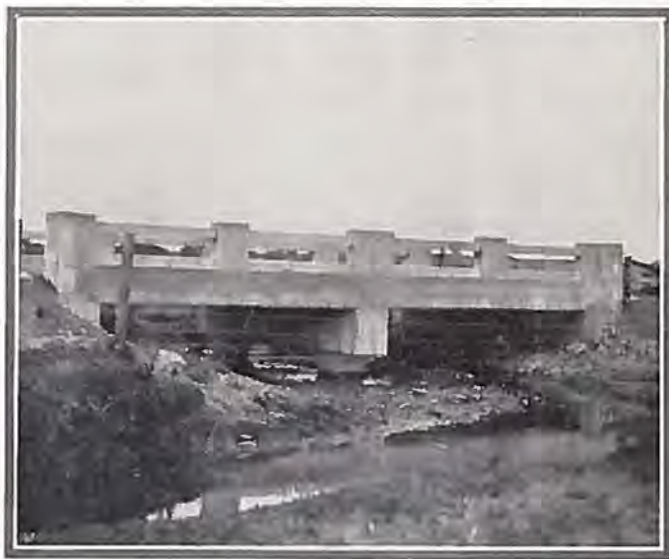
One of the concrete drainage structures on Lafayette-Longmont highway, "built to stay put."
