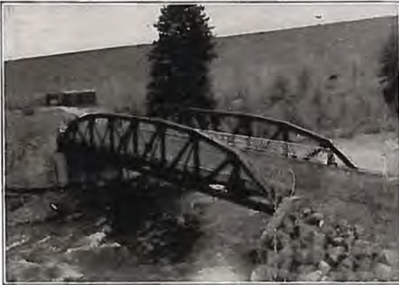
100 ft. Riveted Low Truss Span, Dillon, Colo.
