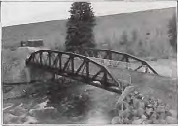
100 ft. Riveted Low Truss Span, Dillon, Colo.
