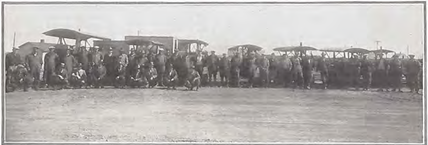
A part of Weld County's splendid maintenance organization with Caterpillar tractor equipment ready for annual spring inspection. These outfits are employed in District No. 1, under direction of Commissioner Dan Straight. Weld County has one of the largest maintenance organizations in the state.
