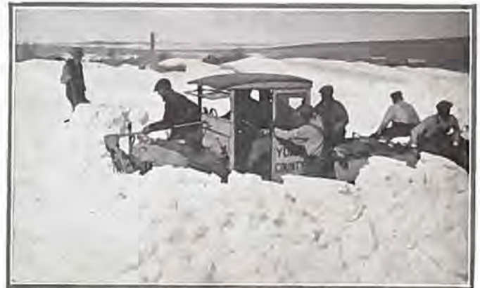
Diggin out of snow on State road near Wray.
