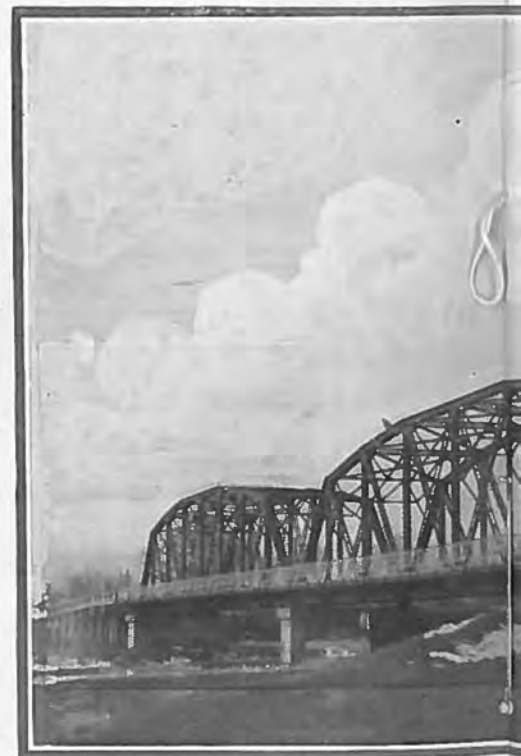
Steel and Concrete 400-Foot. Bridge Over
