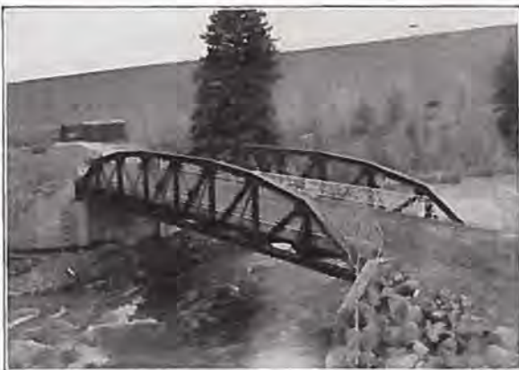
100 ft. Riveted Low Truss Span, Dillon, Colo.
