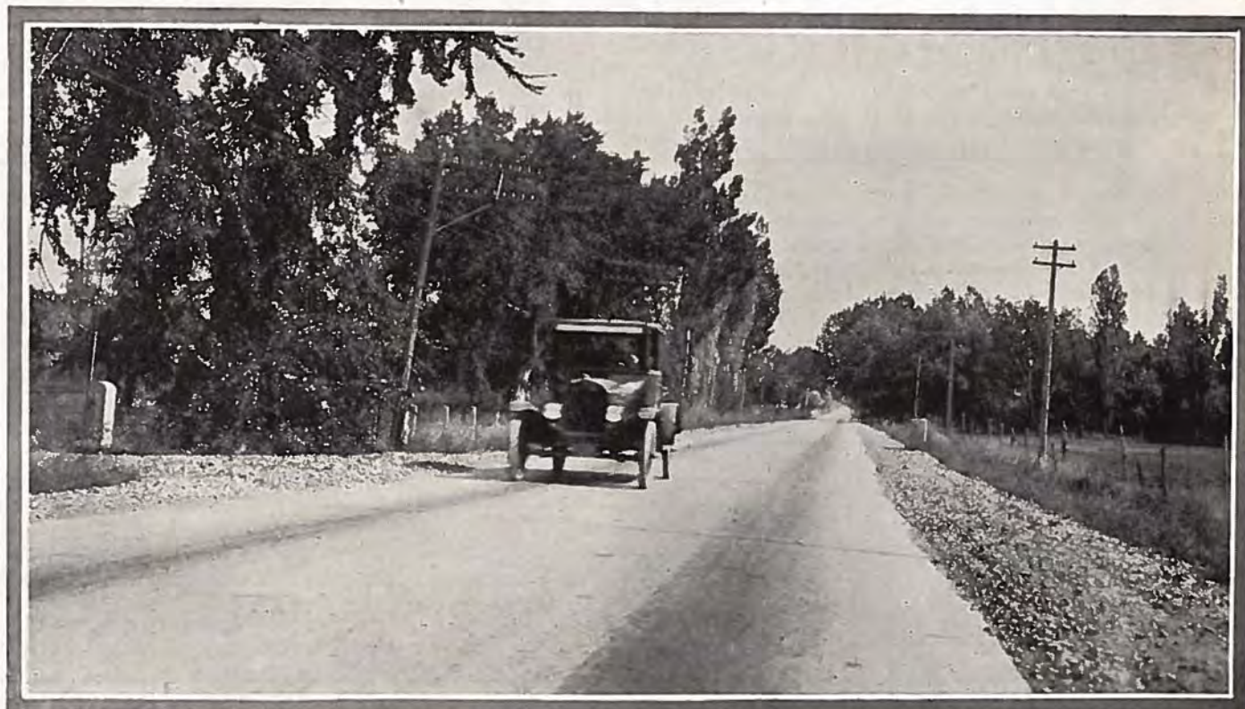
Looking east from Boulder, showing newly completed concrete pavement.
