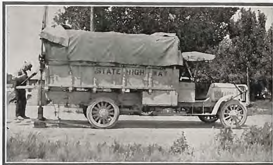
Core drilling machine used by Colorado State highway department in testing concrete pavement.
