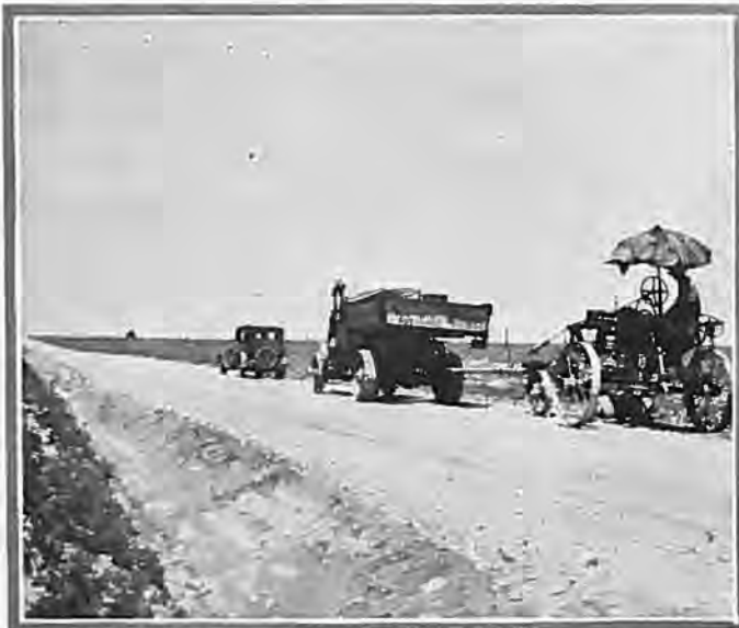
Showing Pueblo County truck-grader maintenance outfit at work on Pueblo-Canon City highway.
