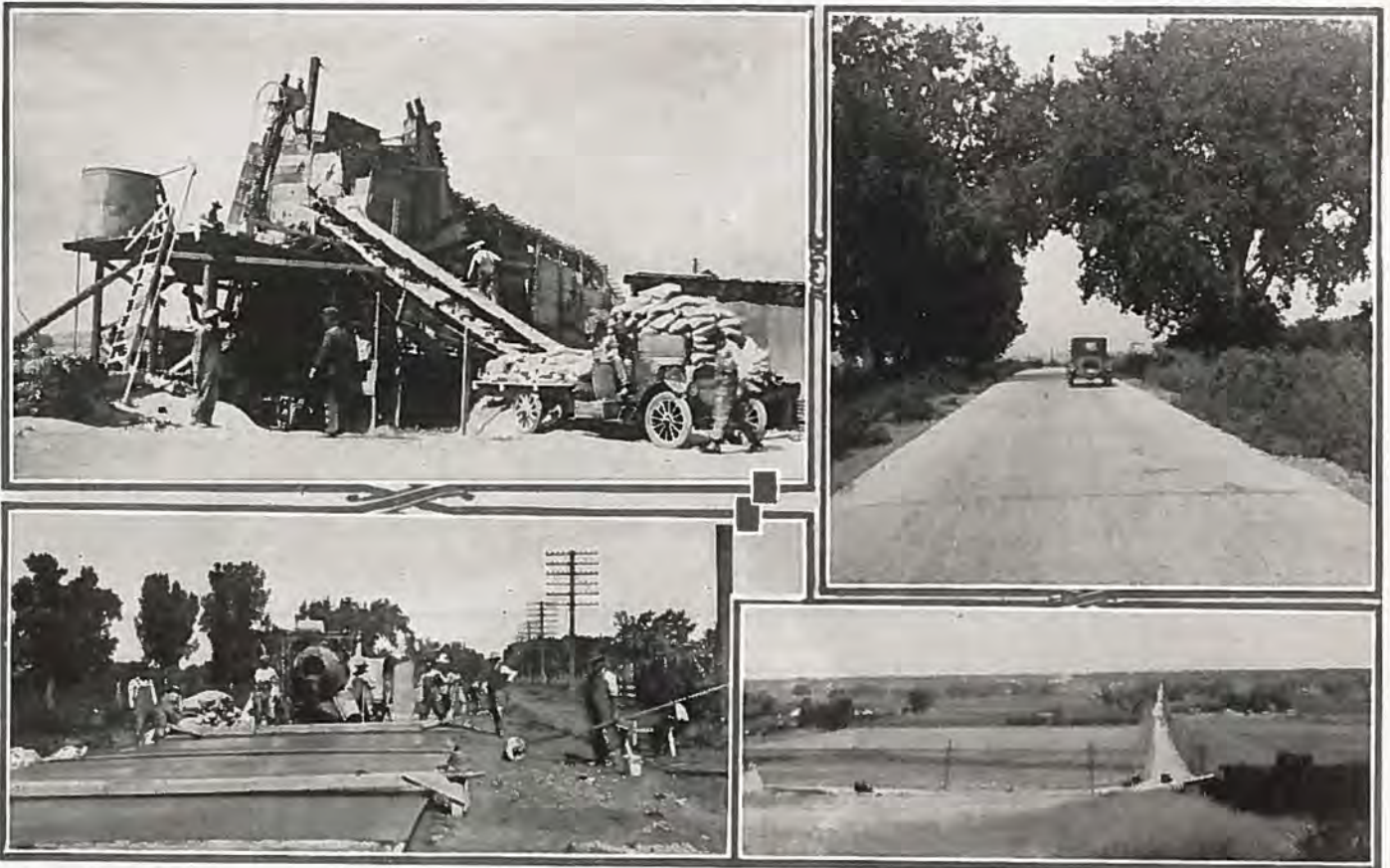
Showing paving operations on new concrete road connecting Loveland and Longmont on U. S. Highway No. 285. Upper left—Central mixing plant of J. H. Miller & Co., contractors. Upper right—View of complete pavement. Lower left—Mixer crew pouring concrete on subgrade. Lower right—View of finished pavement, with Loveland in the distance.
