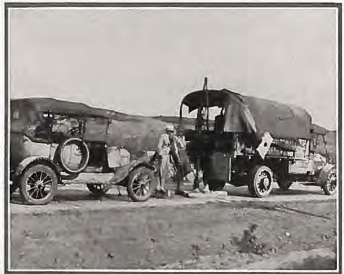
State Highway "core drilling machine" at work on pavement near Castle Rock. These cores are tested for strength of concrete.
