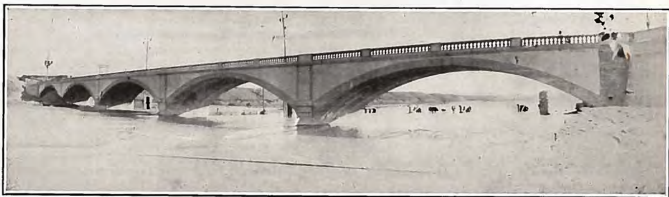
The Huerfano river concrete highway bridge—five 80-foot spans.
