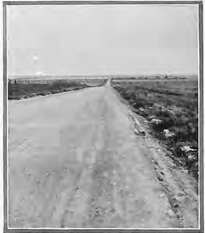
Stretch of gravel surfaced roadway on state highway system near Holyoke.
