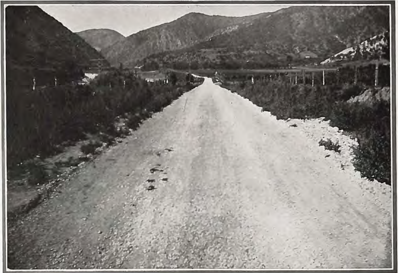
Portion of Completed Federal Aid Project No. 145 West of Glenwood Springs
