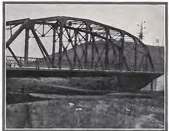
One of the Modern Steel and Concrete Bridges Recently Completed by the State Highway Department, Spanning the Arkansas River on the Santa Fe Trail.
