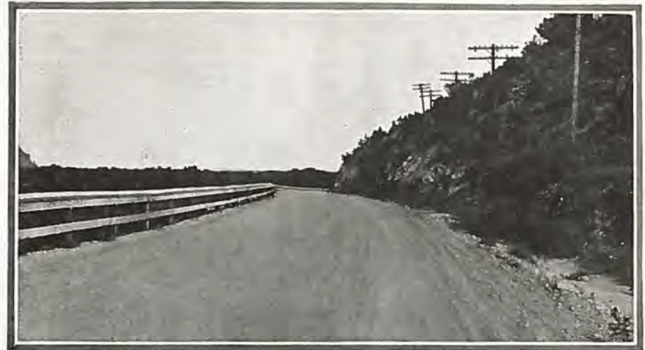
VIEW OF NEW HIGHWAY EAST OF CANON CITY—This beautiful new road was constructed by the State with Federal Aid funds. Note the smooth surface of the gravel and substantial guardrail.
