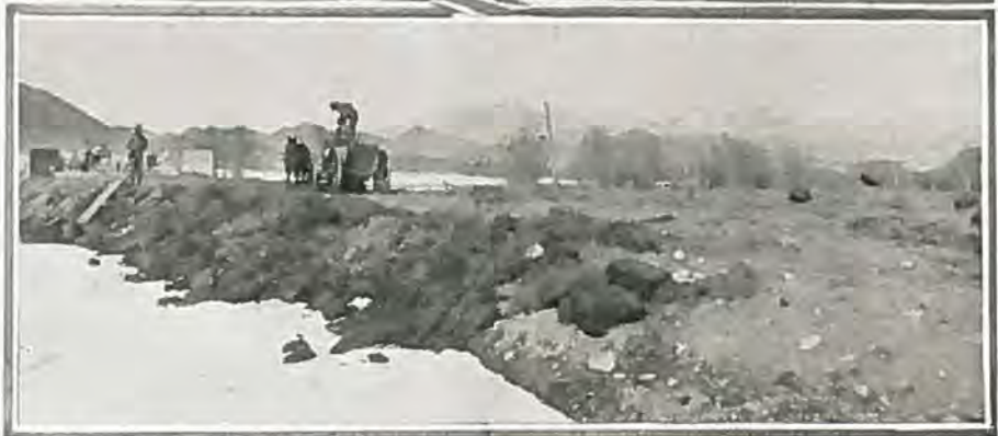
Federal Aid Project under Construction in Saguache County, Showing Heavy Fills and Method of Dirt Handling with Loader
