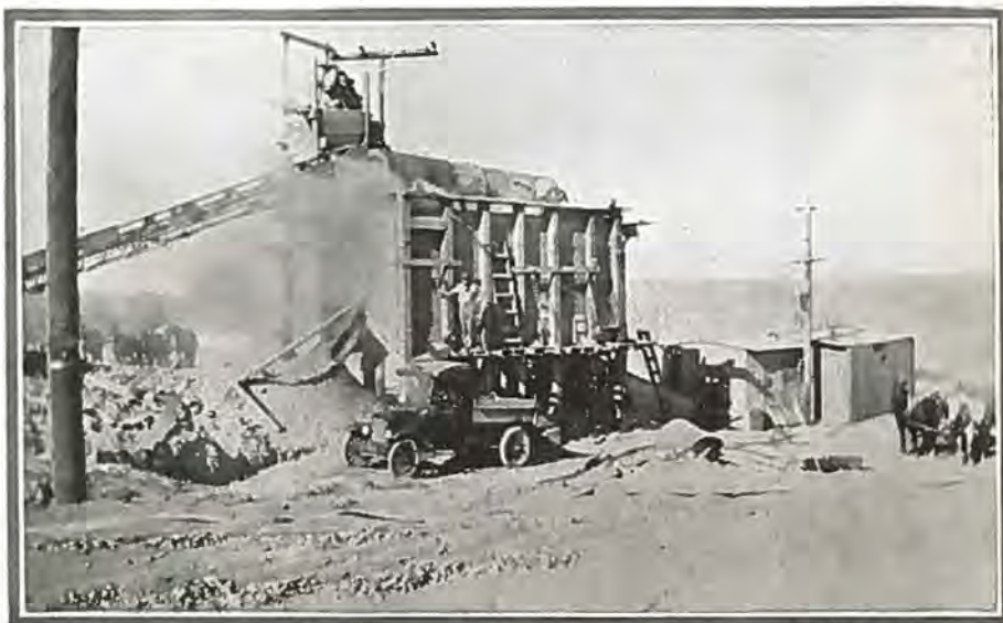
MODERN GRAVEL PLANT —Showing how screen gravel is handled in modern conveying and loading outfit on Federal Aid Job.—Photo by James D. Bell.
