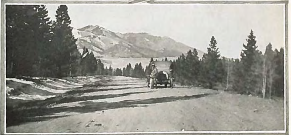
Views of State Road No. 10, showing newly improved stretch on west slope of LaVeta Pass, near the town of Fort Garland, in Costilla county.
