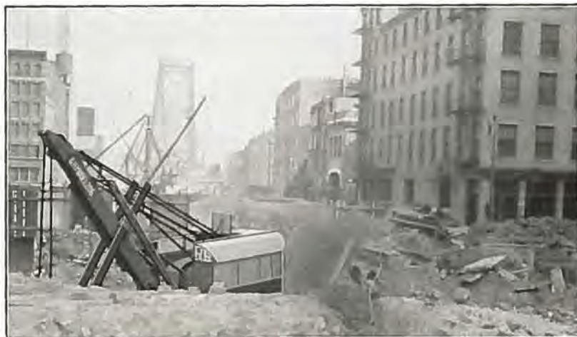
P & H \frac{3}{4} -yd. shovel excavating for Philadelphia approaches of the Delaware river suspension bridge.
