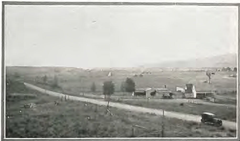
A fine stretch of gravel surfaced road near Hayden on the Victory Highway, constructed with Federal Aid funds.
