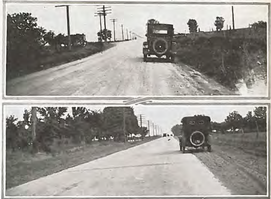
Upper—Showing smooth condition of road between Longmont and Lyons, on State road No. 66. Lower—Stretch of new completed concrete pavement south of Longmont; constructed with Federal Aid funds.
