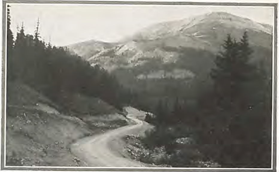
HOOSIER PASS NOW A PLEASURE —The above view shows a stretch of the improved roadway recently constructed by the State Highway Department with State funds. Photo by H. L. Jenness.
