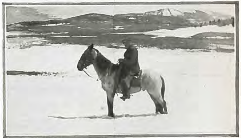
John F. Greene, Resident Engineer, poses "on the trail" of a new Highway above Indian Creek, in Costilla County
