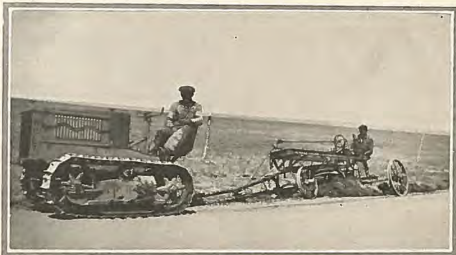
MODERN MAINTENANCE OUTFIT —This type of outfit has been adopted by one of the counties in eastern Colorado as standard equipment.
