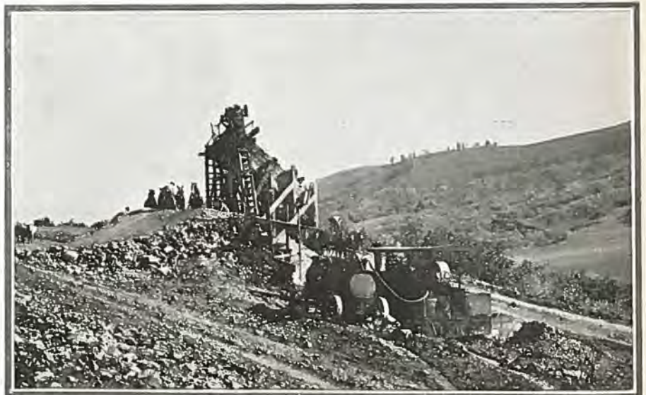
GRAVEL SCREENING PLANT—Working on Hesperus Federal Aid project under construction by Ed. Hansen, contractor.
