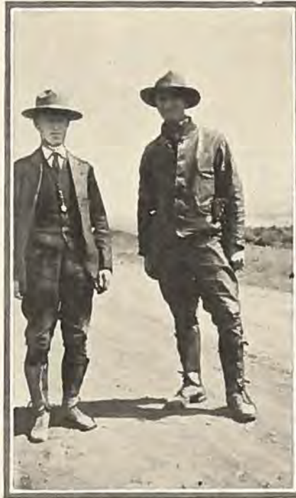
Division Engineer H. L. Jenness and Field Engineer W. A. Whitney on an inspection tour.
