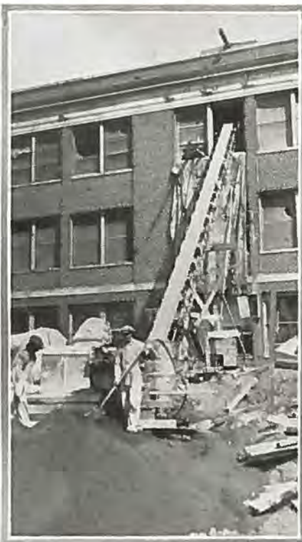
Belt conveyor handling plaster mortar to third story of Mitchell Junior high school in Denver.
