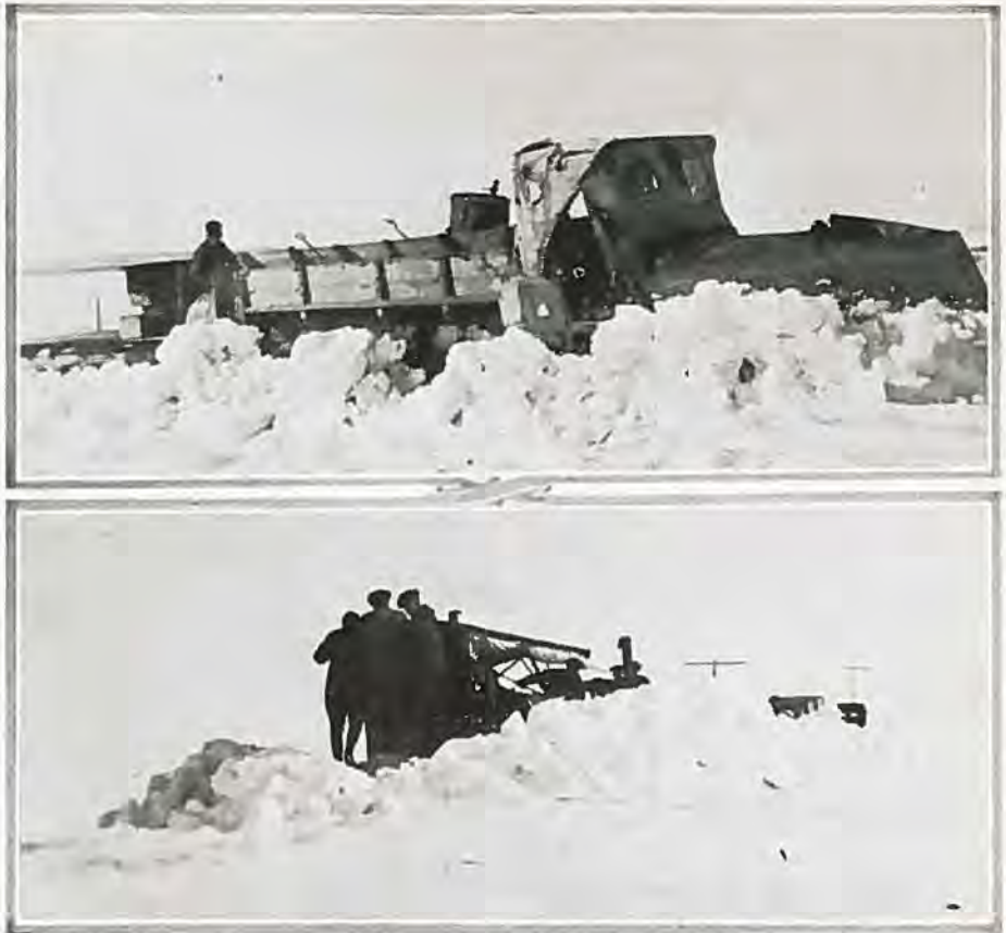
(Upper) Showing how Yuma county utilized a truck with V-plow to clear snow from road. (Lower) Two 10-ton tractors bucking snow in Kit Carson county.
