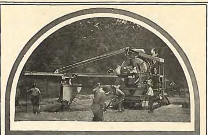
Smith 21-E on Construction Work
