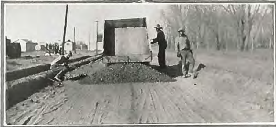
Yes, it's a road—in the making. A Federal Aid crushed rock surfacing project near Monte Vista, recently completed
