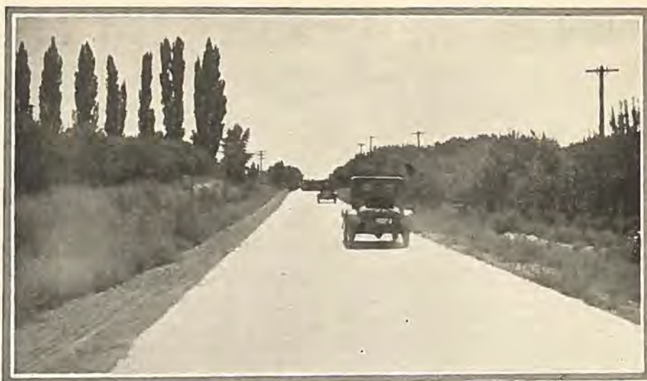
CONCRETE ROAD NEAR GRAND JUNCTION —Several hundred cars daily use this modern pavement at a big saving in operation costs.
