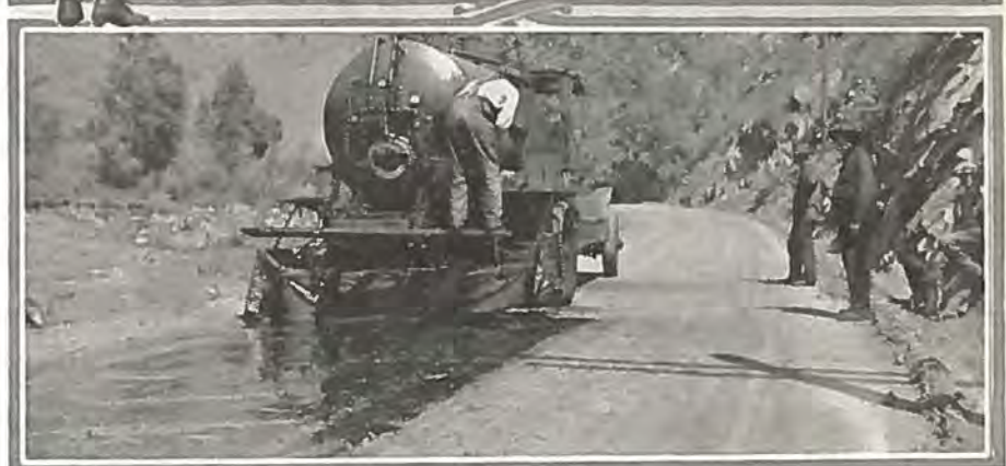
DENVER OILS BEAR CREEK CANON —As an experiment to eliminate the dust nuisance in Bear Creek canon, a part of the Denver Mountain Parks system, the City and County of Denver has oiled one and one-half miles of the roadway west of Starbuck. The work was supervised by F. J. Altwater, city highway commissioner. Mr. Altwater is the gentleman in the center picture wearing a straw hat. Standing at his right is W. T. Murnan, his chief assistant.
