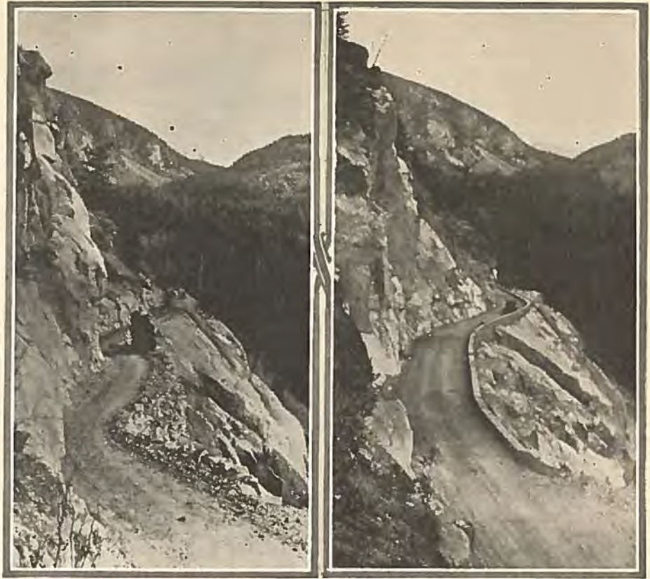
The old and new road on Weller Cliff. Picture on left was taken in 1916. The view on the right was taken in August, 1924, just after the masonry walls were finished. Photos by U. S. Bureau of Roads.
