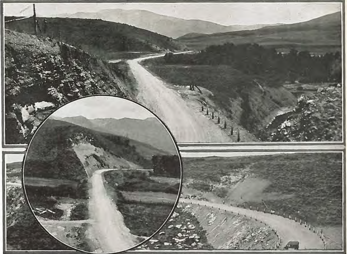
View of the Victory Highway in Colorado—newly completed Federal Aid project west of Steamboat Springs.
