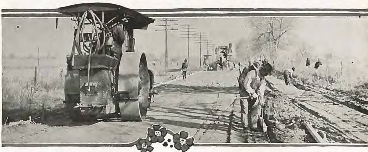
Showing modern methods employed in the construction of Colorado concrete highways—giant roller preparing subgrade in advance of mixer crew.
