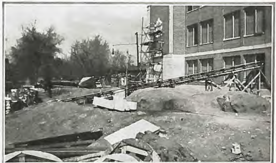
Showing unique conveyor installation for handling mixed mortar on Denver high school building, a modern labor saving device operated by only two men.
