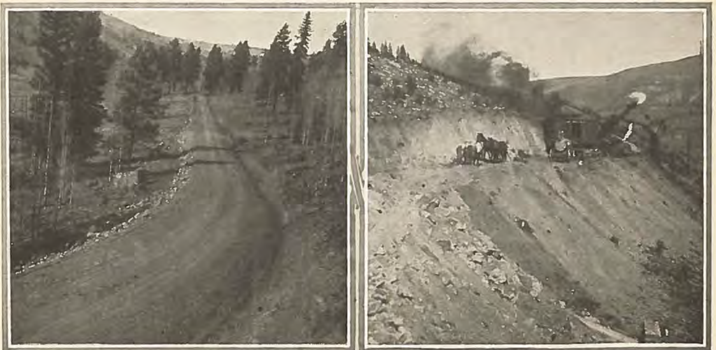
Left—A section of the Conejos canon project, which forms a part of the Cumbres Pass highway. Right—A steam shovel in pay dirt on La Manga Pass section. Photos by courtesy U. S. Bureau of Public Roads.
