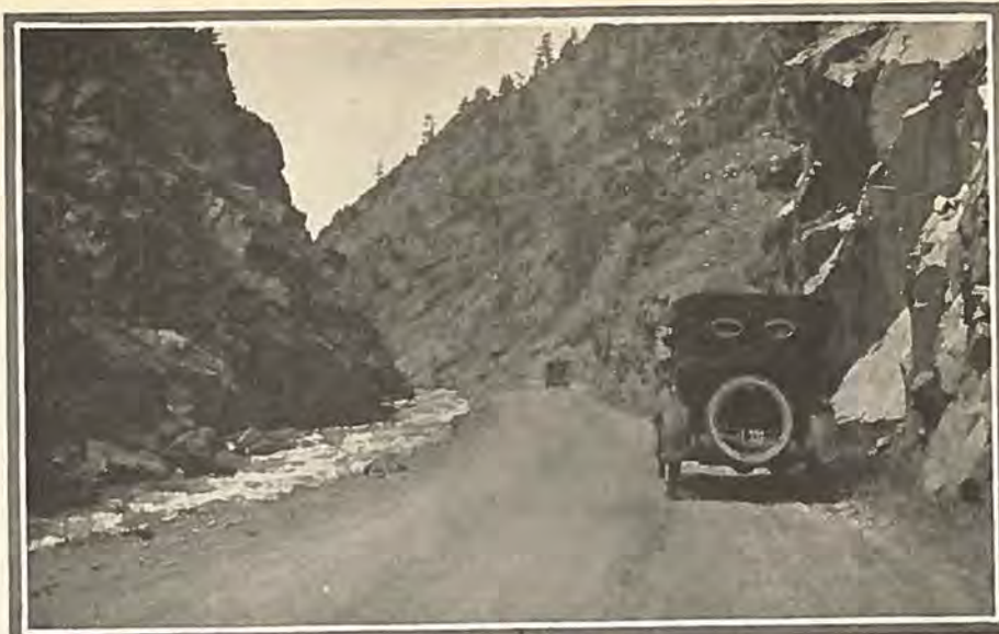
Showing splendid condition of roadway in Big Thompson canon, after completion of project by State highway forces in co-operation with Larimer county.
