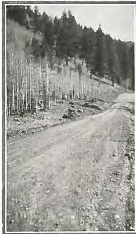
Finished Grade in Conejos Canon, State Road No. 10, to Cumbres Pass
