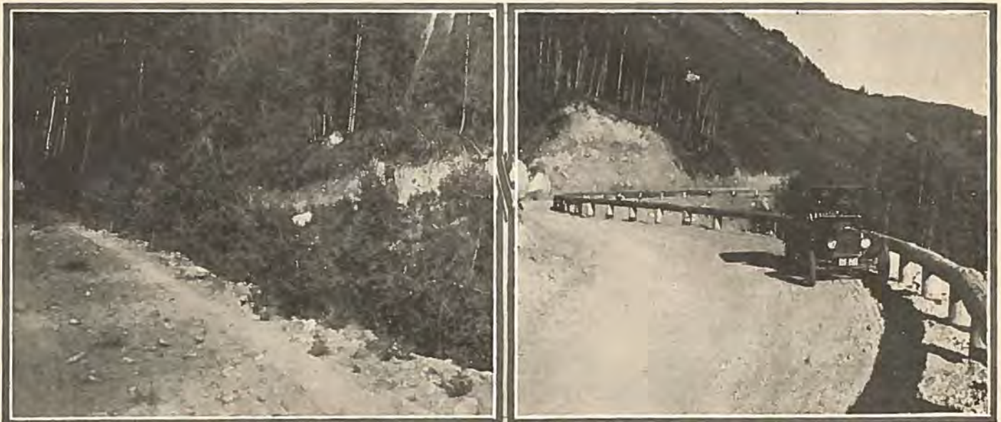
Before and After on the Independence Pass Road—"The Hair Pin" on old road—A large car could not make this turn without backing up several times. (Right) Same spot after completion of new road. Photos by U. S. Bureau of Roads.
