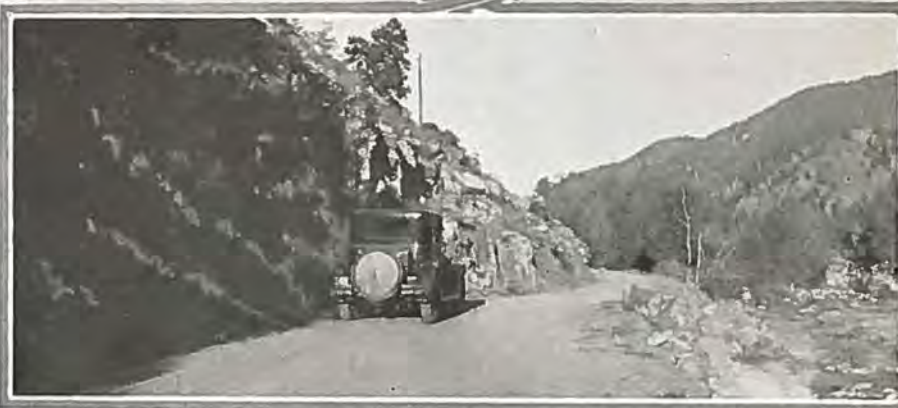
SCENES IN POUDBRE CANON—Middle view shows the far-famed Poudre tunnel located at the "Little Narrows." The canon at this point is only thirty feet wide. The tunnel bore is thru solid granite.
