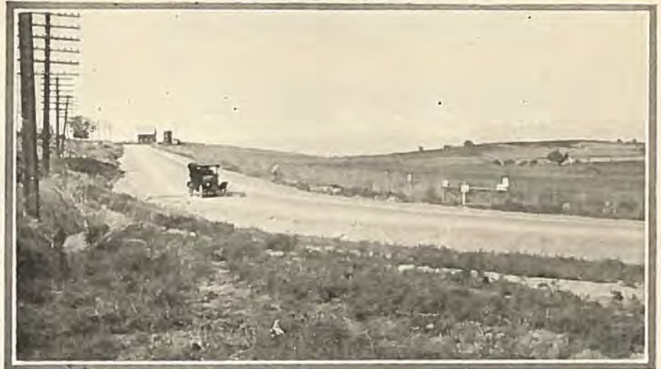
CAR OWNERS SAVE MONEY ON PAVEMENT—View showing a stretch of concrete road located south of Loveland in Larimer county on State Road No. 1.
