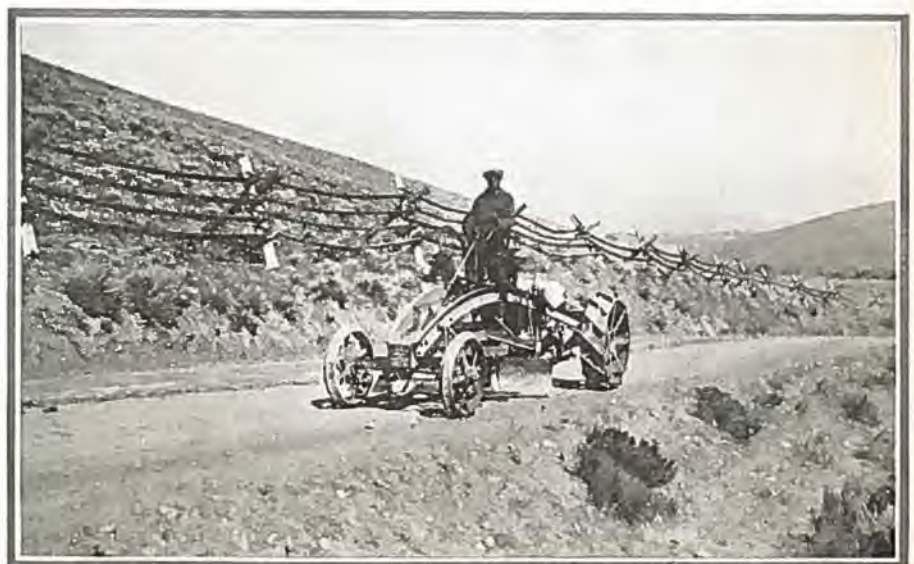
ONE-MAN MAINTAINER IN GRAND COUNTY—Type of maintenance machine operated on Victory Highway near Granby and Grand Lake.
