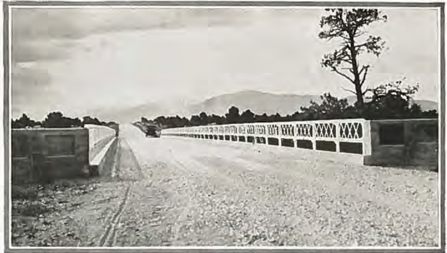
NEW BRIDGE NEAR SALIDA—This modern steel and concrete structure was completed with Federal Aid early in 1925. It forms a part of a fifteen-mile stretch of gravel surfaced highway.—Photo by Staff Photographer.
