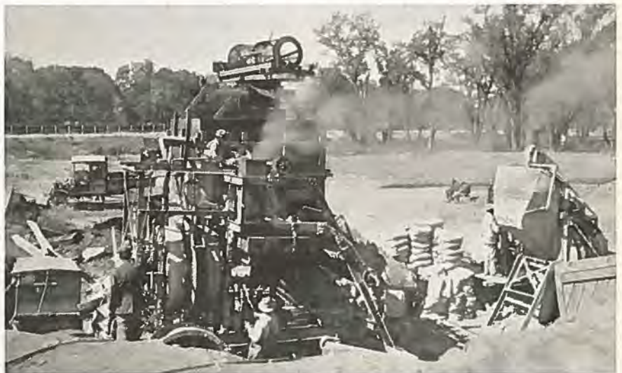
A unique "Two Mixer" set up, used by a contractor in conjunction with a fleet of small speedy trucks in laying one of Colorado's concrete pavements in record time.
