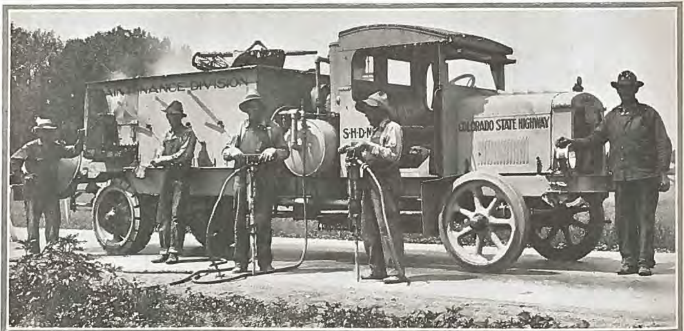
NEW CONCRETE MAINTENANCE MACHINE OPERATED BY STATE —This outfit is moved from one section of the state to another, making repairs on concrete pavements and bridges. It is equipped with concrete mixers, paint brushes and jack-hammers.
