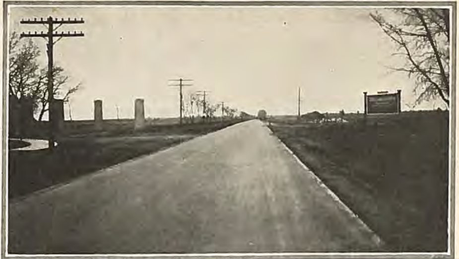
COLORADO'S FIRST STRIP OF ASPHALT HIGHWAY—This piece of asphalt pavement is located in front of the Fitzsimons Hospital east of the town of Aurora in Adams county.
