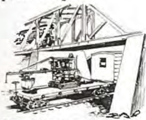
There is no superstructure to dismantle when shipping a Smith Paver. It clears all railroad trestles.
