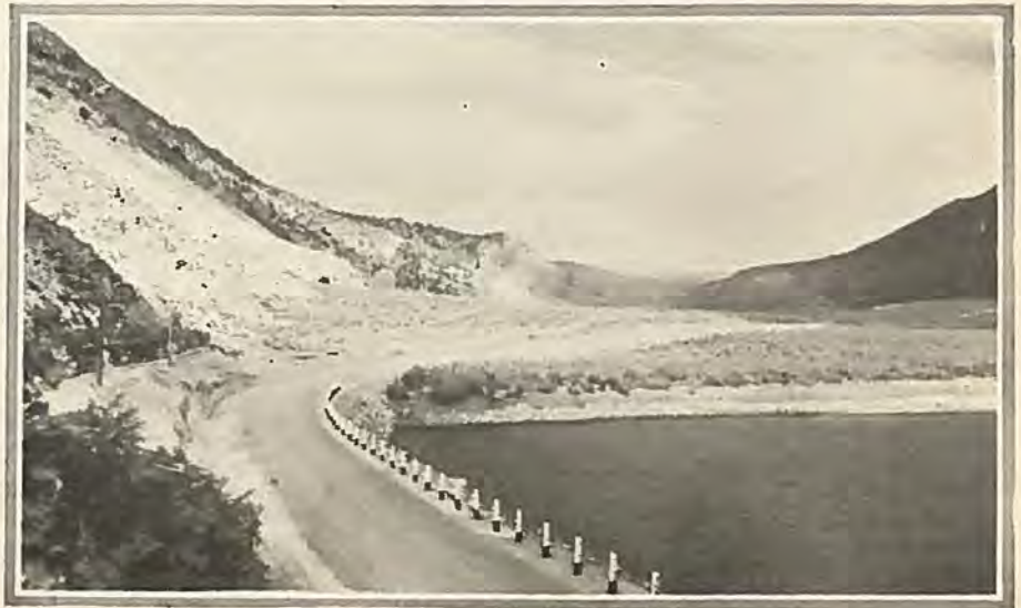
VIEW OF GRAVEL ROAD NEAR GYPSUM—This is a gravel surfacing project just completed by the State Highway Department under a Federal Aid agreement.
