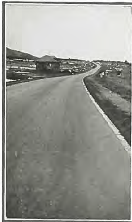
ASPHALT PAVEMENT NORTH OF TRINIDAD —Six miles of this pavement was completed in 1925, constructed according to U. S. standards.—Photo by James D. Bell.
