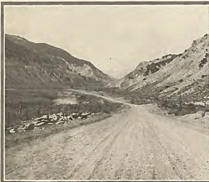
New and Old Road Between Dotsero and Gypsum—(Left) A section of the new Gypsum-Dotsero highway, showing fine gravel surfacing. (Right) Part of the abandoned trail through sagebrush, once the roughest road between Leadville and Grand Junction. Photos by Worth C. Knowles.
