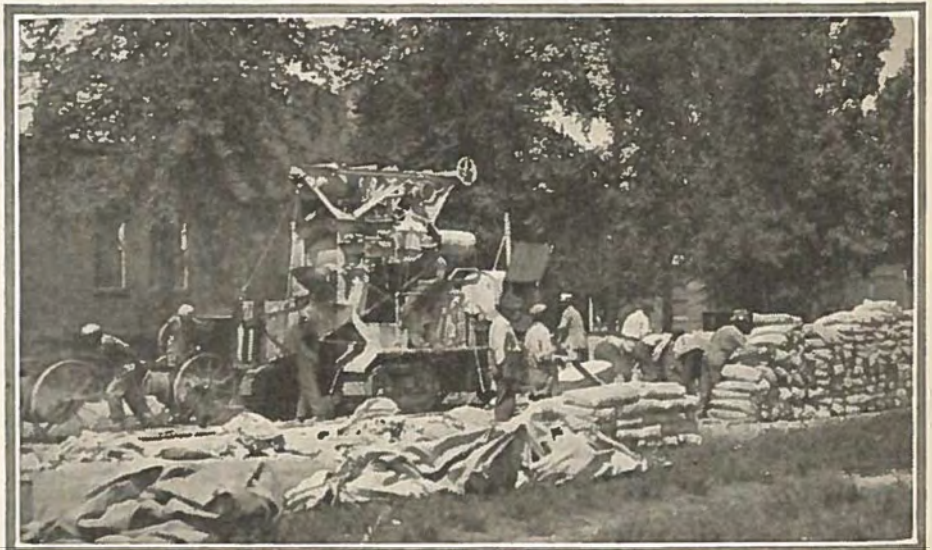
MIXER CREW BREAKS RECORD —Showing Rex paver owned by W. F. Pigg & Son, contractors, in action on alley paving job in Denver.
