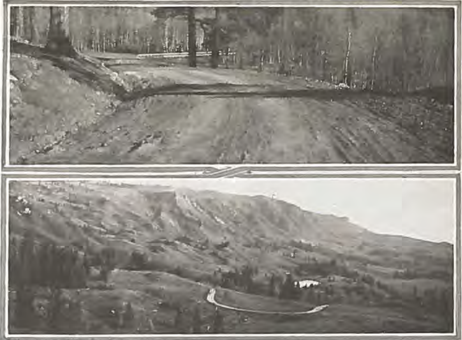
Upper—A wide, smooth curve approaching guard railed fill, on Cumbres Pass. Lower—View on west side of the Cumbres Pass, looking toward New Mexico after new road was completed. Photos by courtesy U. S. Bureau of Public Roads.
