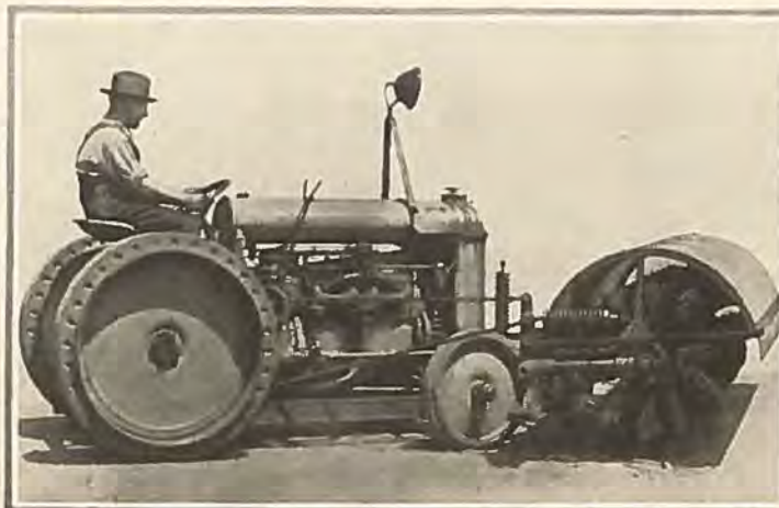
Type of Fordson sweeper designed by F. J. Altwater, Highway Commissioner, being used by the City of Denver.
