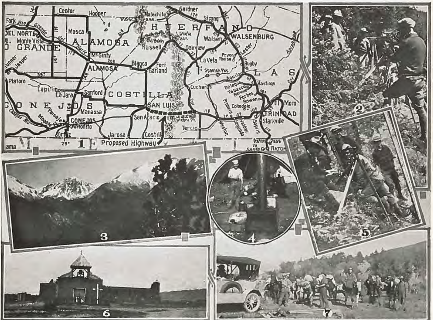
(1) Dotted line on map shows proposed new road over San Francisco pass. (2) Setting up transit under difficulties. (3) Showing peaks of Culebra range. (4) The most popular man in camp. (5) Engineering party above Purgatoire creek. (6) Mission in San Pablo built in 1854. (7) Moving camp from San Francisco creek.
