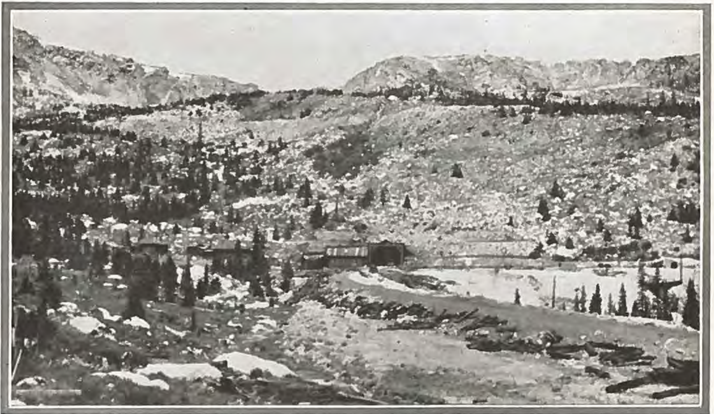
VIEW OF EAST PORTAL OF THE BUSK-IVANHOE TUNNEL —This old railroad tunnel, two miles in length, is now being rehabilitated by the State Highway Department for automobile use. The roadbed was presented to the state by A. E. Carleton, Colorado Springs millionaire.
