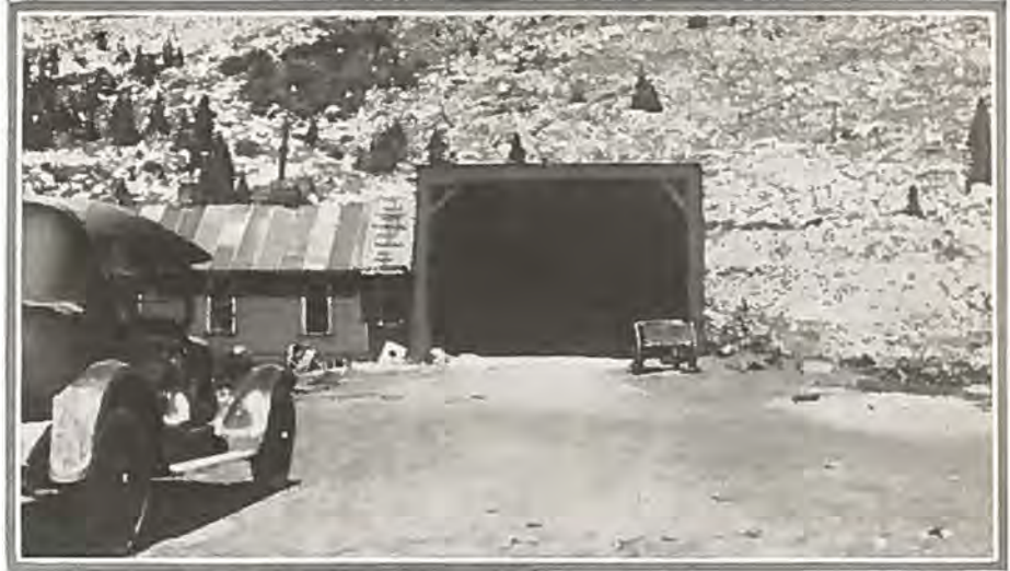
CLOSE-UP OF BUSK-IVANHOE TUNNEL —Showing snow shed at east portal, with roadway in splendid condition. A breeze blows thru the tunnel constantly, eliminating possibility of bad air. It is one of the longest highway tunnels in the world.
