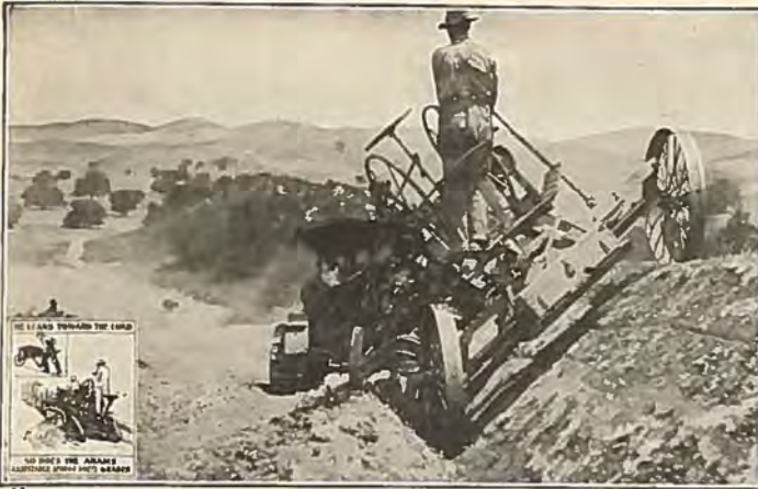
12 ft. Adams Grader at work cutting a high back-slope by riding up on the banks. No grader without "Leaning Wheels" could do this work.
