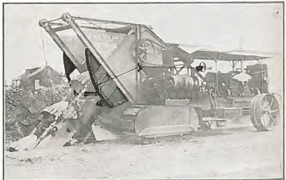
Buckeye traction ditcher, showing new stabilizer.
