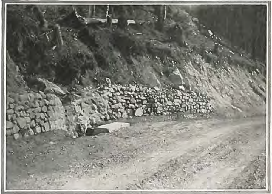
Modern drainage structure constructed on Colorado mountain highway
