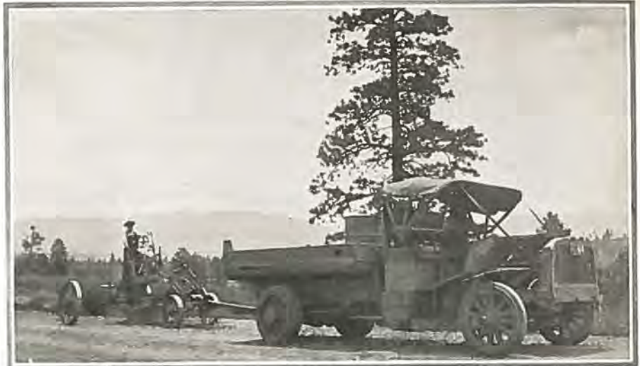
Maintenance outfit of La Plata county taking "wrinkles" out of State Highway west of Durango.
