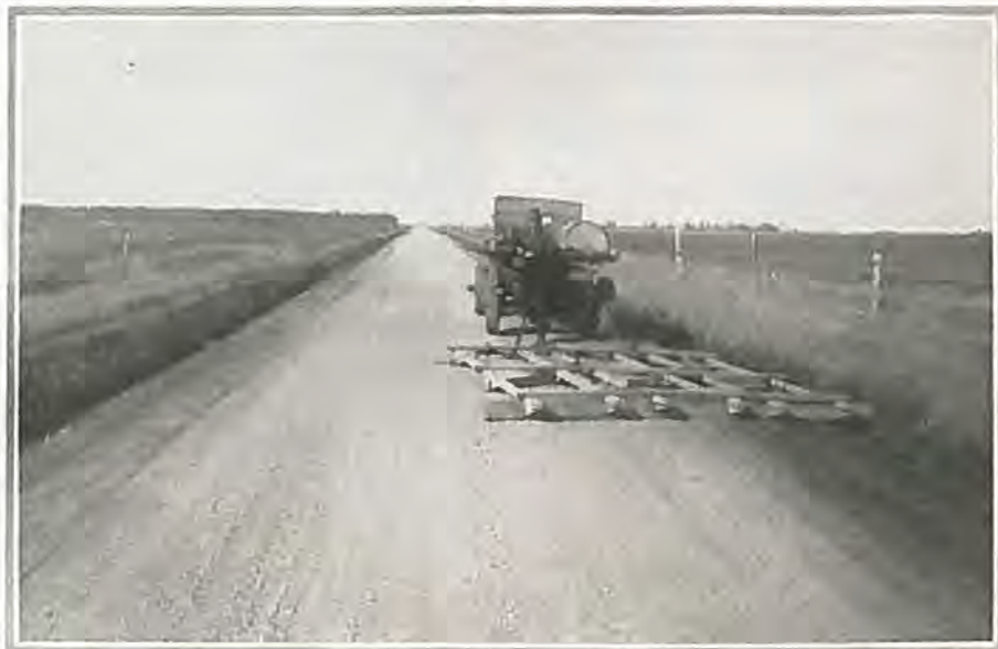
Maintenance outfit in, Yuma county showing specially constructed road drag.
