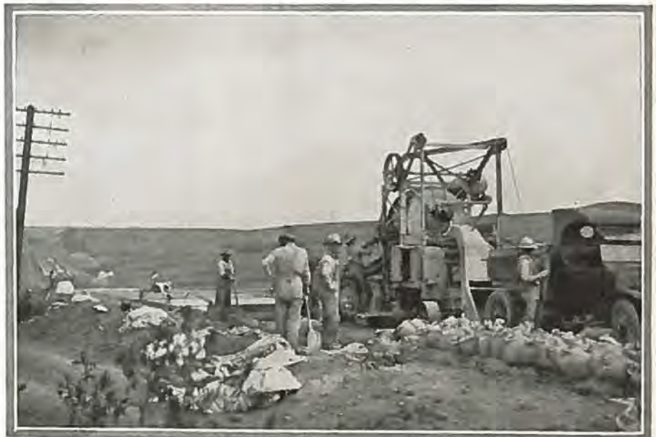
Koehring 21E Paver at work on Broomfield concrete pavement.
