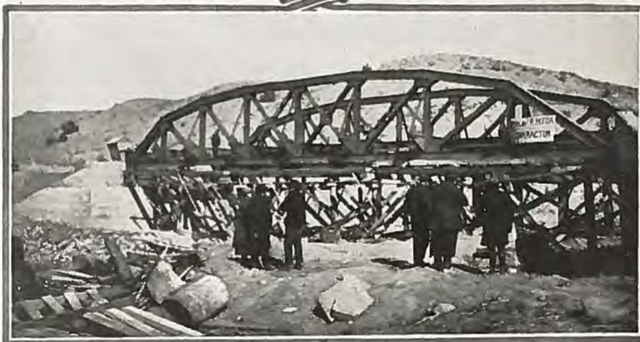
Top—Showing bridge assembled on roadway. Lower—After being rolled into place over Beaver Creek, near Florence.
