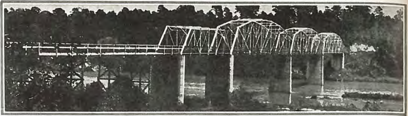
Bridge reconstructed by North Carolina Maintenance Forces.
