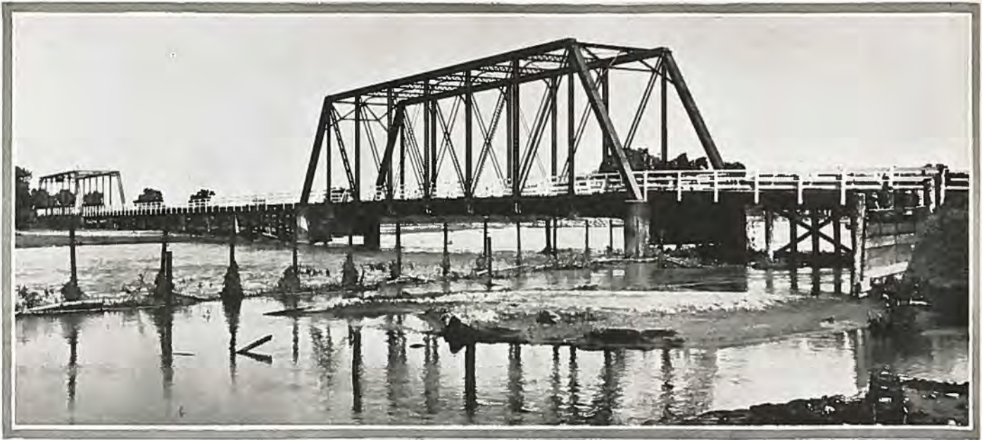
Reconstructed steel bridge over Arkansas River east of Pueblo, erected with county funds.
