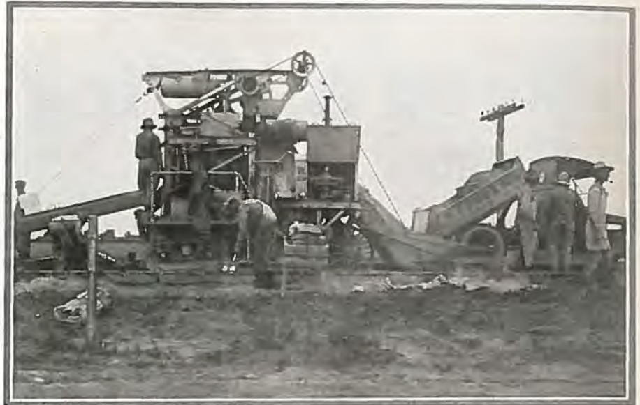
Concrete mixer outfit which broke paving record on Fort Morgan-Brush highway project.
