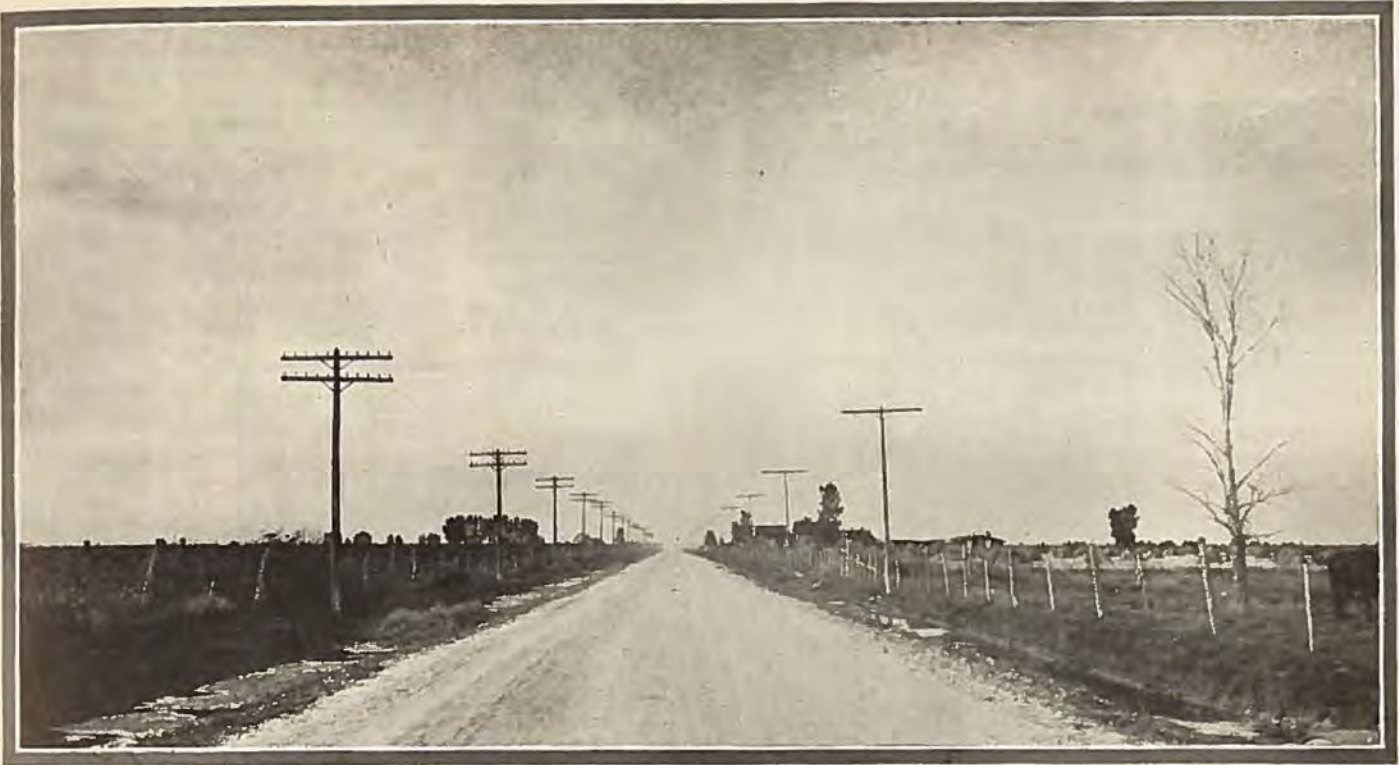
A fine example of modern road construction is the Gunbarrel road. Scene is looking north from Monte Vista, showing gravel surfacing after completion of Federal Aid Project. Photo by Bureau of Public Roads.
