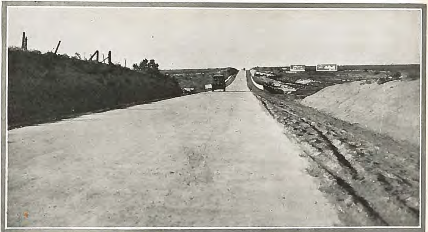
Showing a stretch of the new constructed concrete pavement south of Wollhurst.
