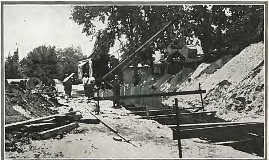
The above is a picture of the first dragline sold by the Koehring Co. It is a No. 2, caterpillar type, and is being used on a large sewer project in Denver, laying 66-in. concrete pipe.
