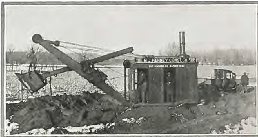
Steam shovel excavating approach to under-pass railroad crossing, near Walkurst.
