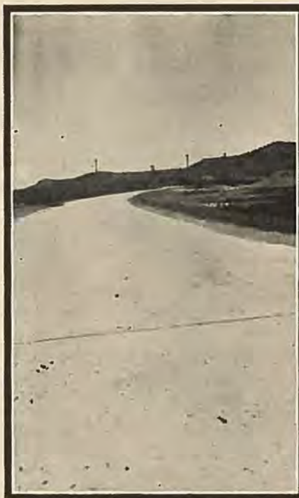
This view of the Denver-Colorado Springs concrete highway exemplifies the "spiral curve."
