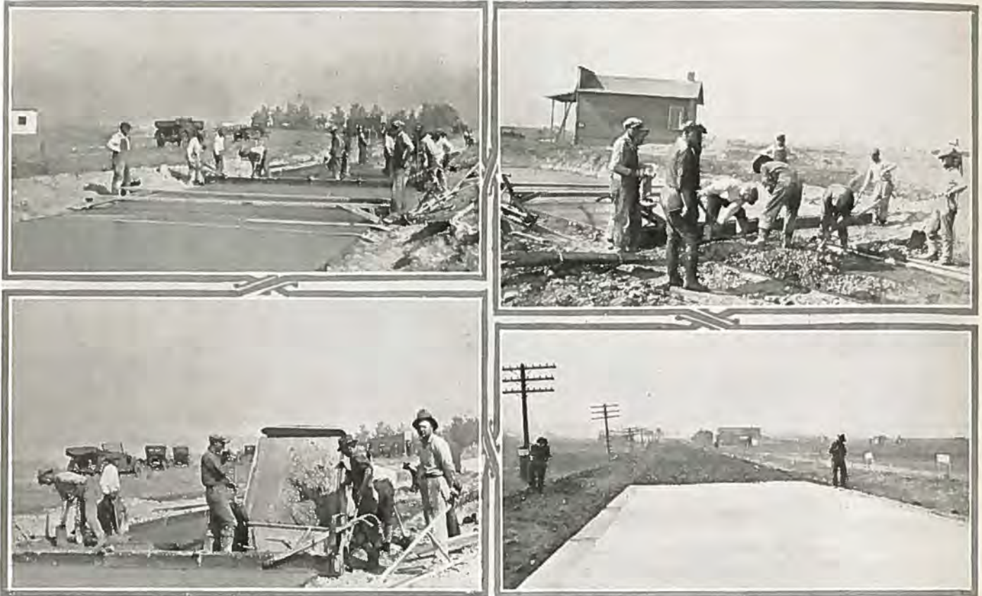
Showing method of handling concrete on Denver-Morrison project, completing pavement between these two points for heavy traffic.
