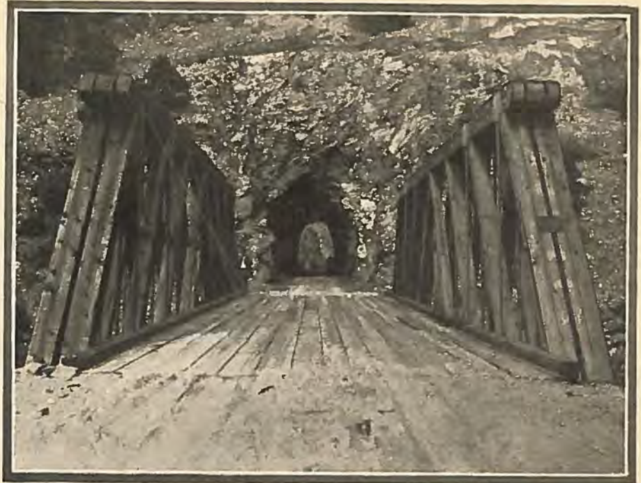
Phantom Canon, showing how old railroad bridge and tunnel have been converted into a modern scenic highway, forming a link in one of the most beautiful and interesting circle tours in Colorado. Photo courtesy of Colorado Springs Chamber of Commerce.
