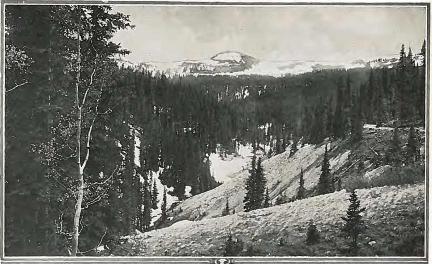
Scene on Wolf Creek Pass, elevation 11,000 feet, showing section of new highway constructed by State Highway Department forces.
