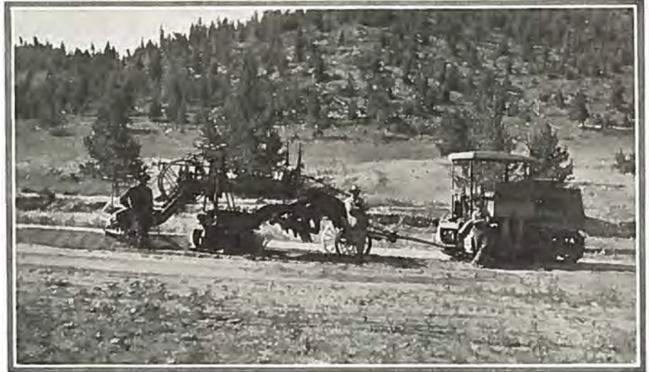
Scarifier-grader and tractor at work on Trout Creek Pass in Chaffee county.
