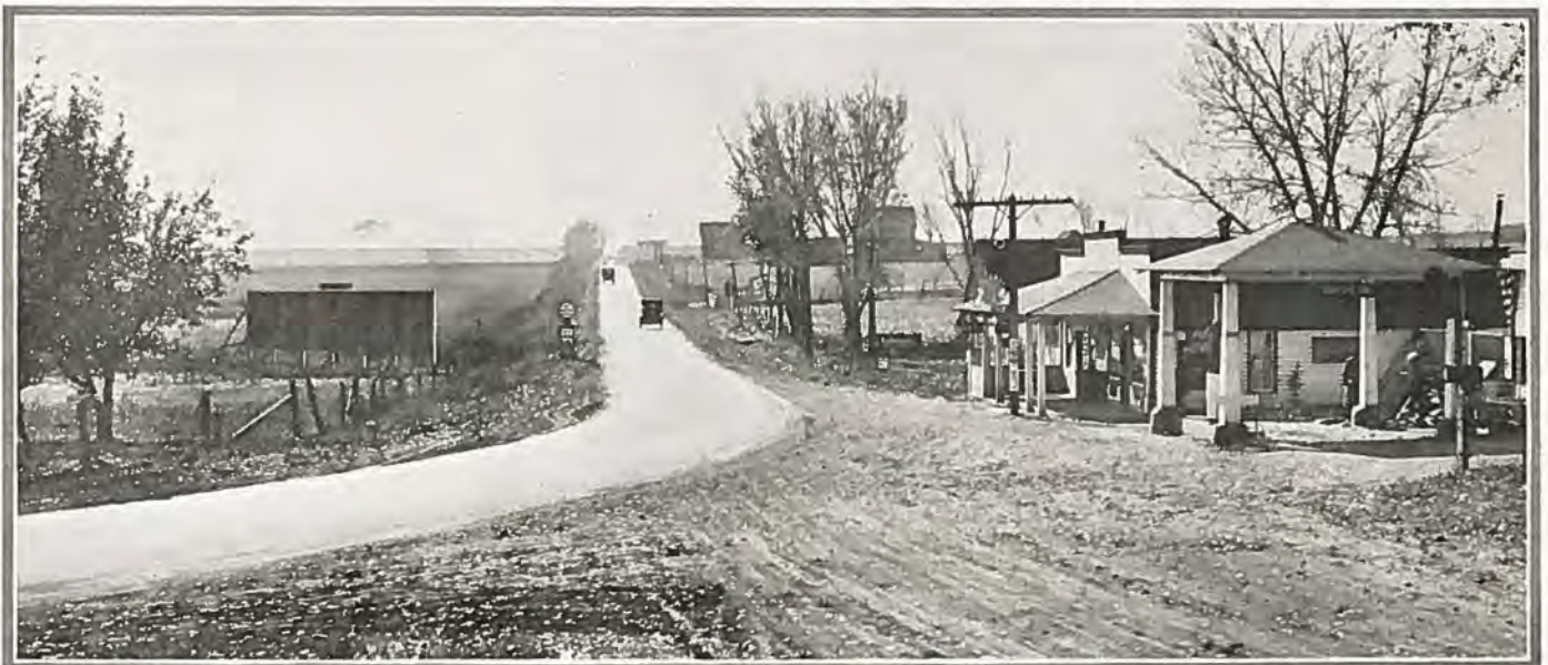
A stretch of the new concrete highway between Denver and Morrison, connecting with the Denver Mountain Parks, recently opened to traffic.
