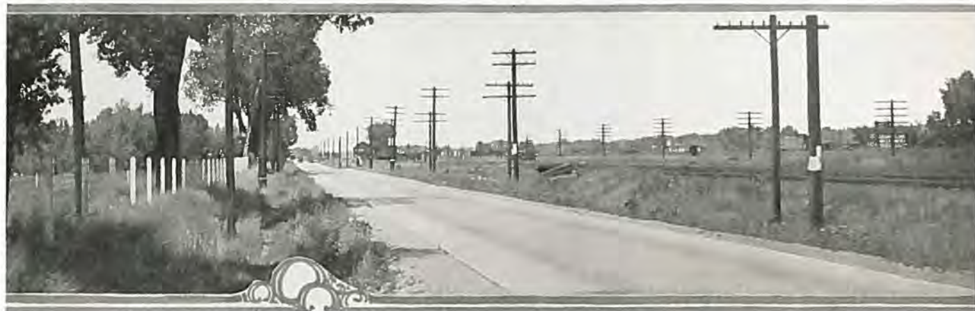
A stretch of pavement on one of Colorado's heavily travelled trunk line highways—located near Littleton. A daily average of 3,000 passenger cars and trucks pass over this road.
