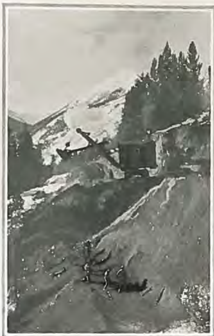
Steam shovel eating away earth from mountain side to make room for one of America's finest mountain boulevards.
