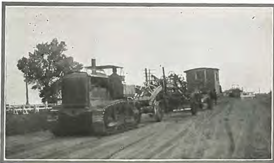
One of Weld County's modern road building outfits, designed for heavy construction work.
