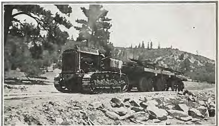
Hauling steel for the new Piedra state highway bridge near Bayfield.
