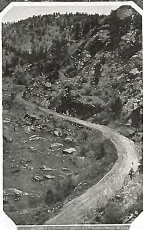
Top—Scene near Hell Gate on newly constructed Midland Trail. Center—Showing completed highway through Eleven Mile Canon.
