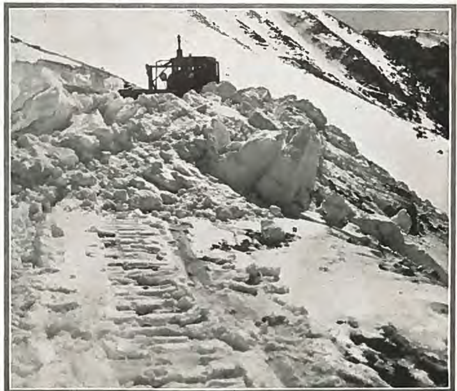
Showing Best Tractor and Blade outfit clearing snow from Pikes Peak highway.
