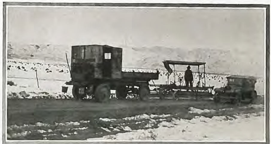
One of the maintenance patrols employed to keep the "wrinkles" out of the detour between Wolhurst and Gann, on State Highway No. 1, during construction of the concrete roadway between these two points.
