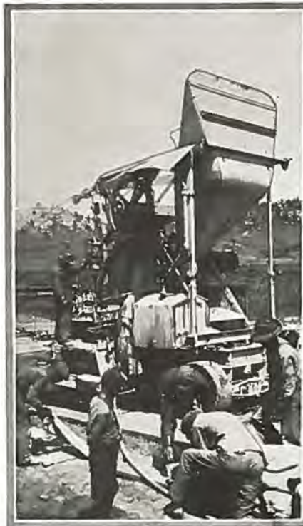
Concrete paver at work on Federal Aid project north of Colorado Springs, on State Road No. 1.
