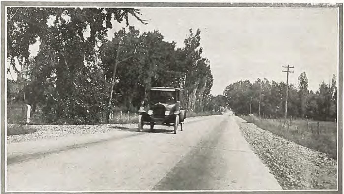
Looking east from Boulder showing new "shoulders" made of crushed volcanic rock.
