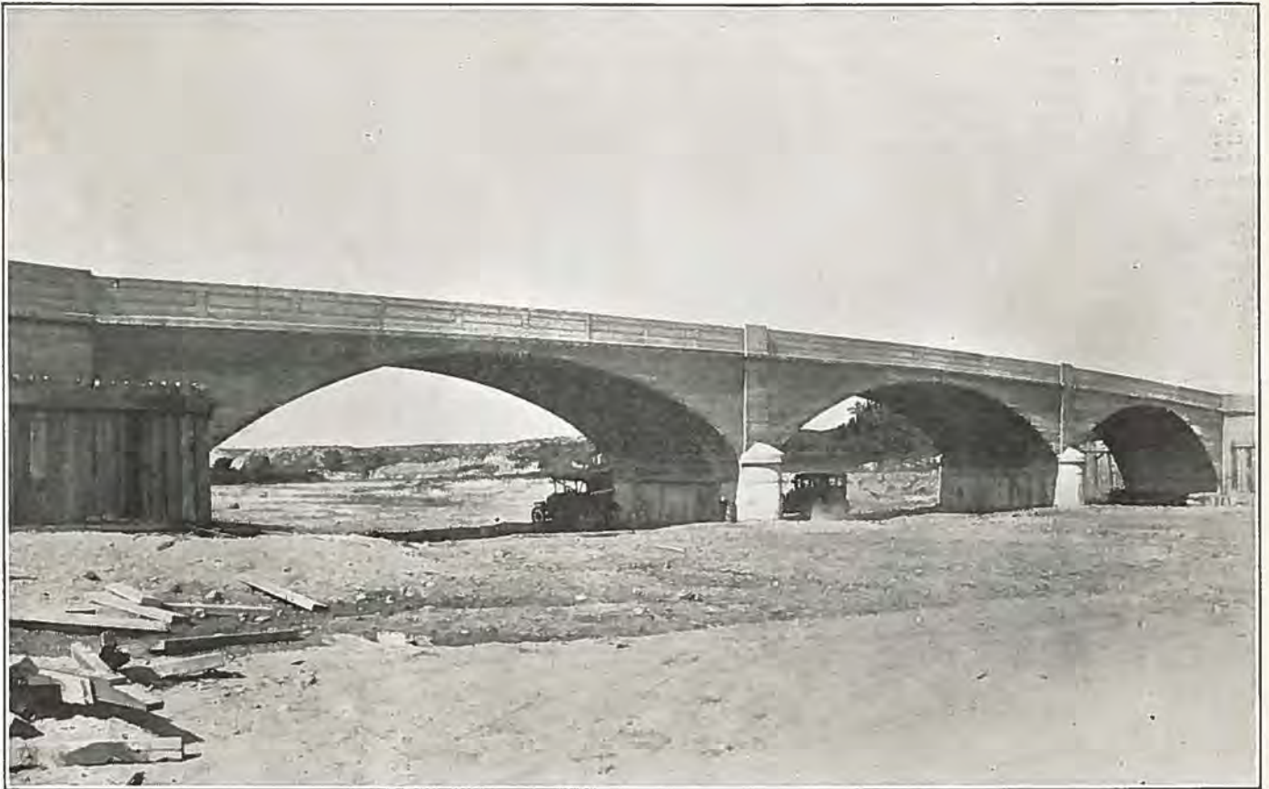
New 300-ft. Concrete Bridge Over St. Charles River in Pueblo County Recently Completed.
