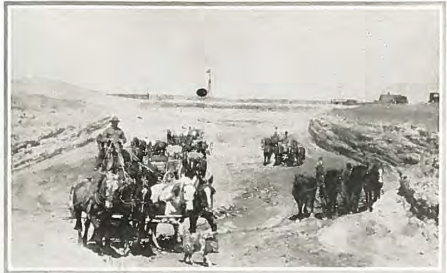
One of Yuma County's numerous gravel pits, showing farmers hauling material on "yard-mile" plan.
