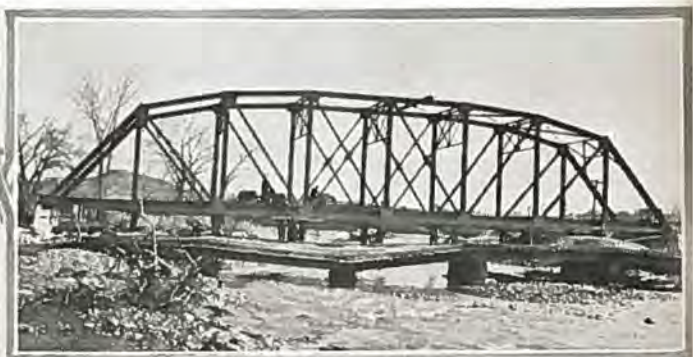
New steel highway bridge under construction on State Road No. 72, near Arvada in Jefferson county.
