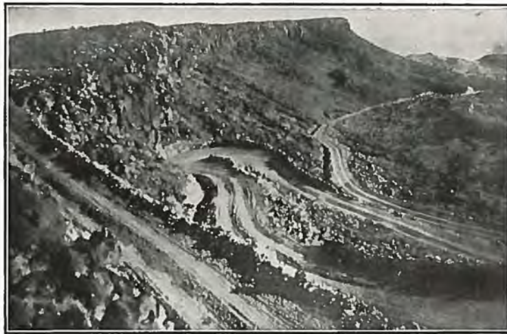
NEW MEXICO STATE HIGHWAY NO. 1
