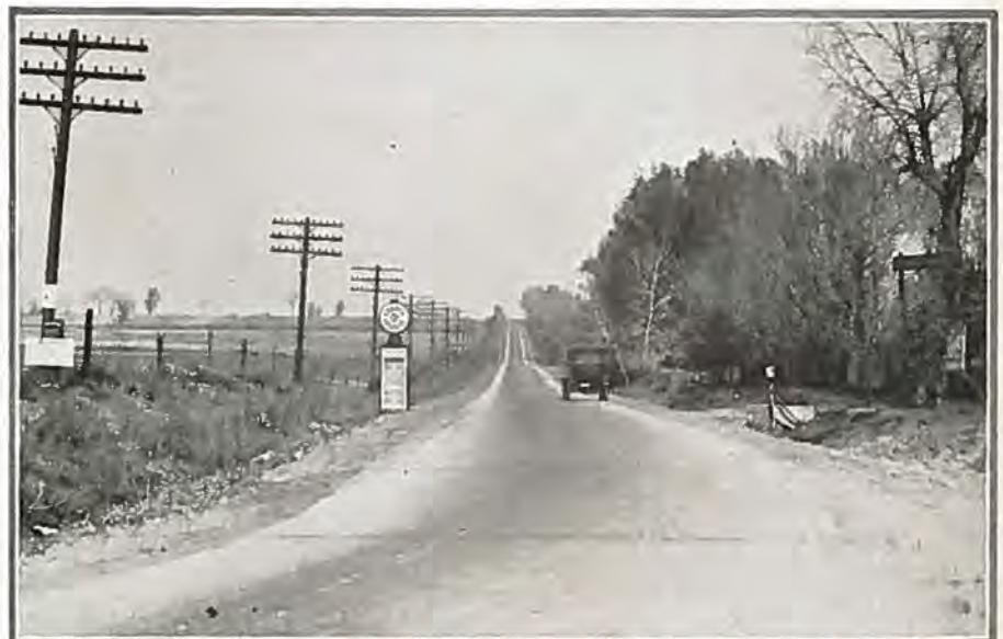
A stretch of new concrete highway located east of Morrison, now connected with Denver with continuous pavement.
