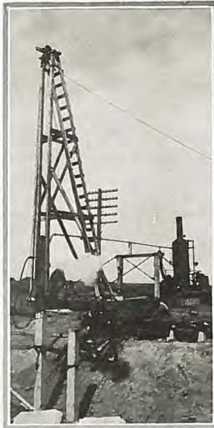
Driving piles for concrete bridge near Lafayette in State Highway No. 1.
