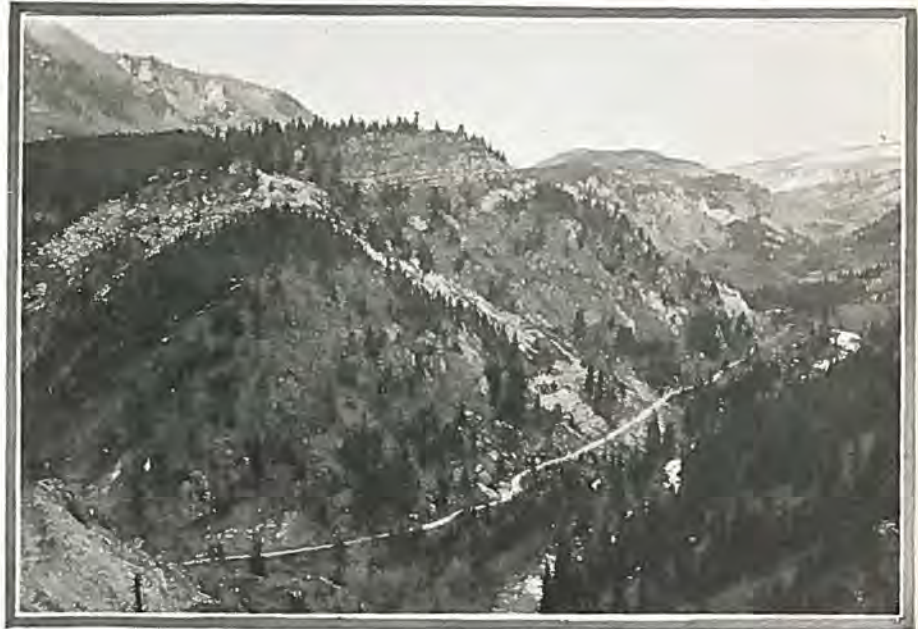
View of State Road No. 4 from Red Cliff looking toward Tennessee Pass.
