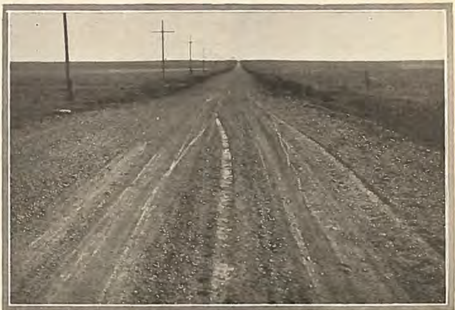
Modern gravel surfaced all-year highway located in Eastern Colorado, constructed with State and County bond funds. Roads such as this attract thousands of tourists to Colorado each summer, adding tremendously to the wealth of the state.
