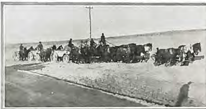
Elevating grader outfit moving dirt on State Road No. 1, south of Lafayette, preparatory to laying pavement.
