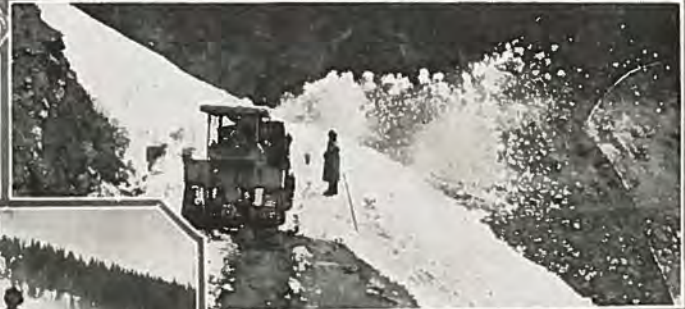
Upper left—Side view of rotary plow and tractor outfit. Upper right—Front view of rotary wheel. Lower left—Clearing way thru snow slide. Lower right—Making 8 ft. cut thru slide on danger curve. Insert—"Sleepy Bill," the human measuring stick, takes snow reading.
