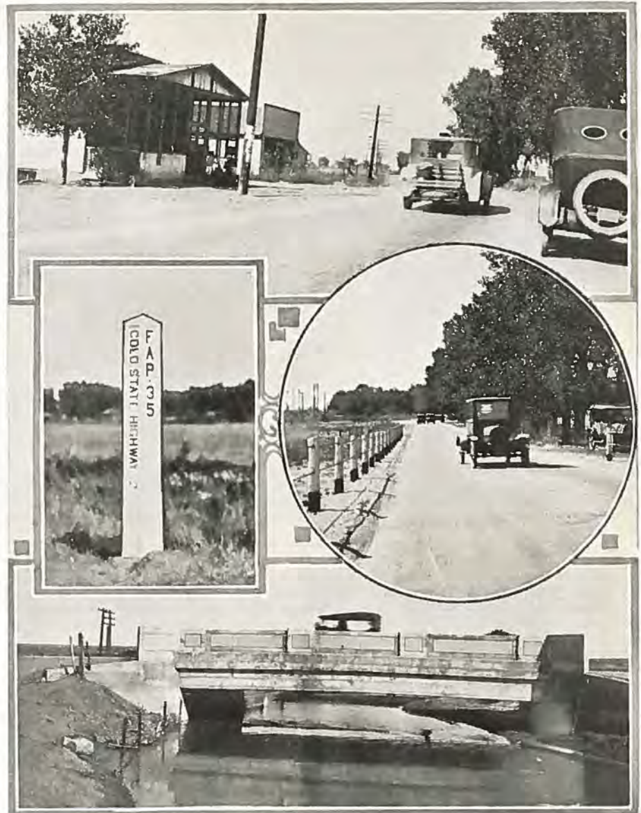
Upper—A Motorway bus passing thru Ione. Center, left—New concrete guide post. Center, right—Looking west toward Riverside Cemetery, Denver. Lower—Concrete bridge over irrigation canal near Platteville.
