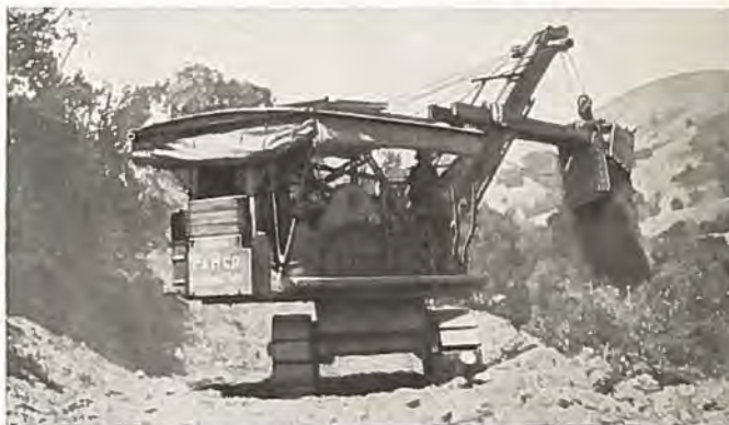
P & H 206 Gasoline Shovel owned by Arvid Olson, Denver.
