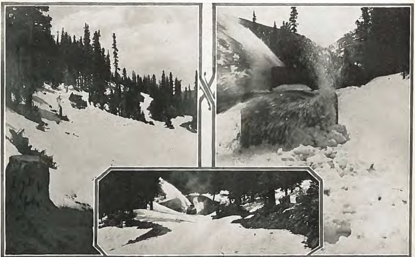
Left—View of Berthoud Pass highway, with plow bucking 6 ft. of snow. Right—Showing front of rotary wheel throwing snow 250 ft. down slope. Insert—Plow emerging from 20 ft. drift, with temperature two above zero.
