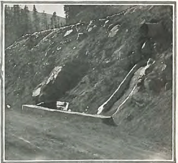
One of the numerous drainage structures consisting of catch basins and corrugated culverts laid below frost line. —Photos by courtesy of Bureau of Public Roads.
