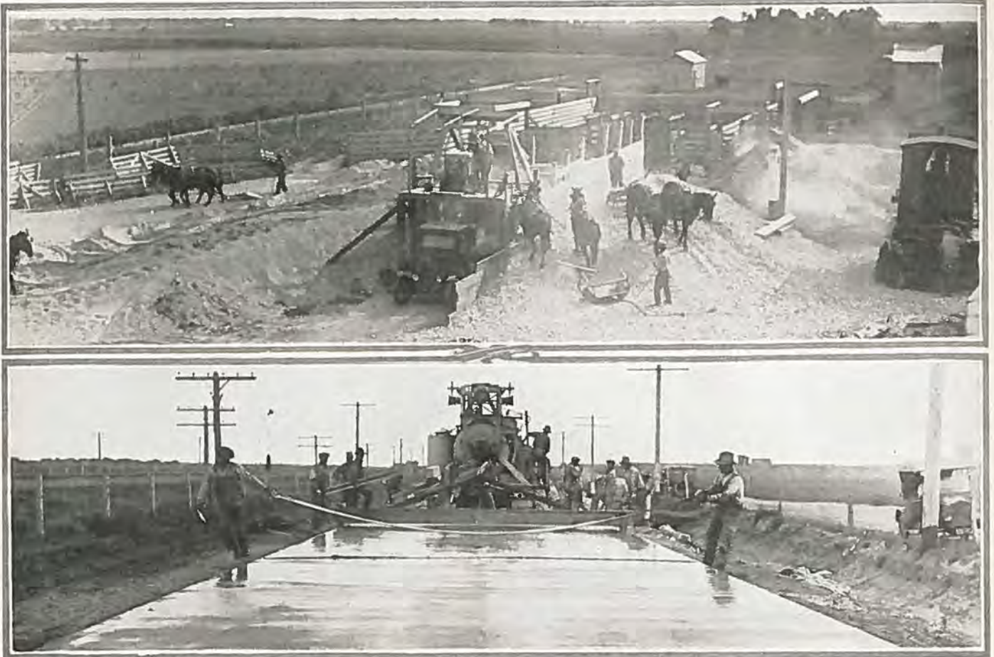
Showing screening plant mixing materials for concrete highway near Brush. (Lower picture)—Shows workmen finishing top of pavement.
