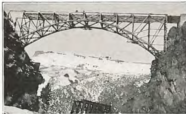
Sapinero Bridge Fabricated and Erected by
