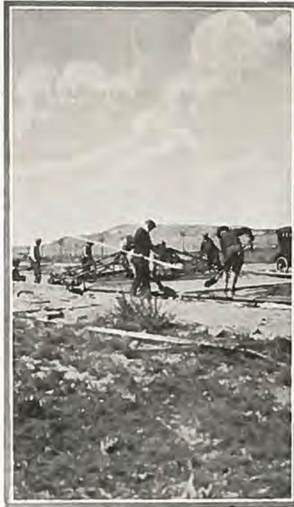
Showing operation of concrete finishing machine which insures smooth riding surface of highway pavements.
