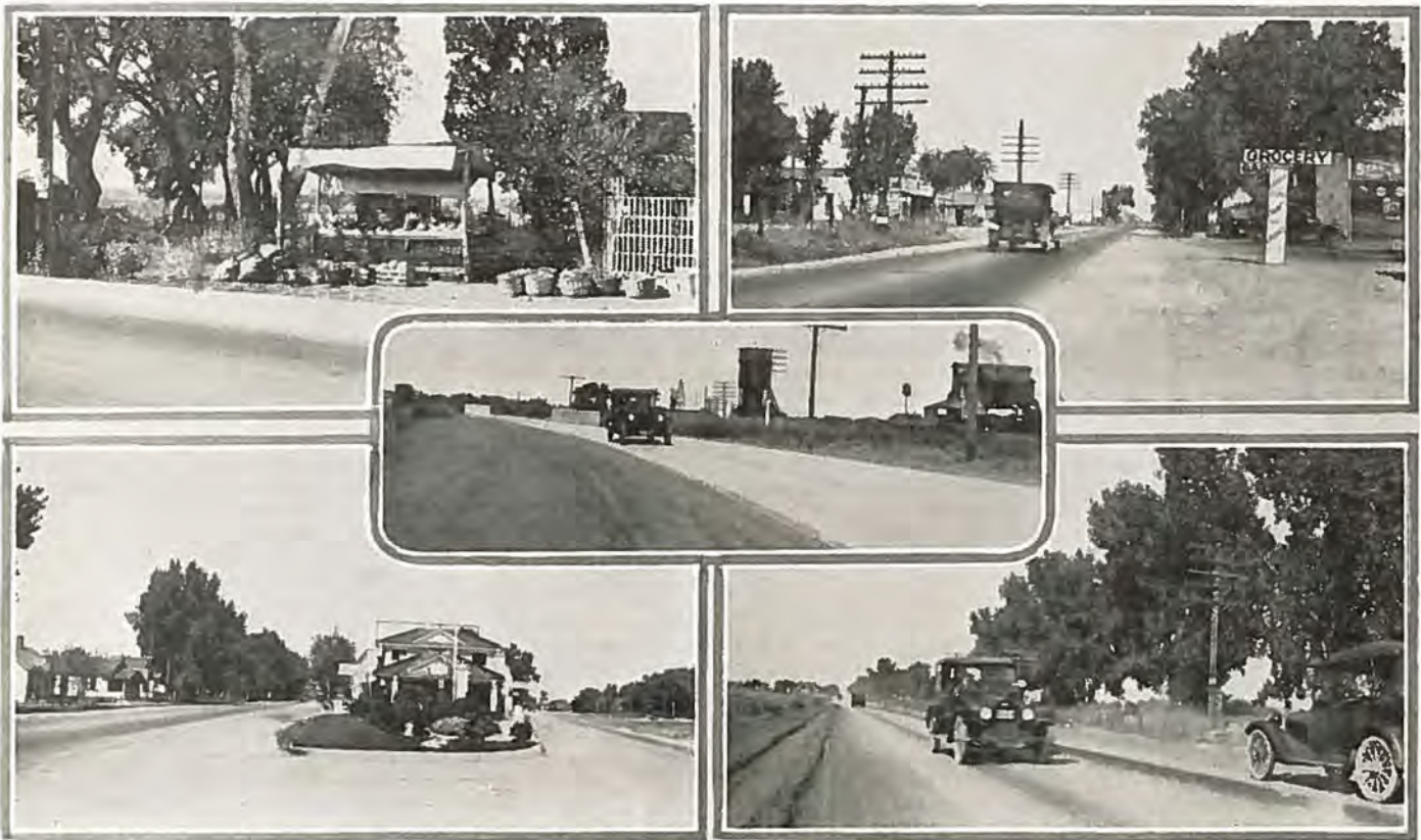
Scenes along the Denver-Greeley concrete highway. Upper left—Truck farmer's stand near Henderson. Upper right—Town of Henderson. Center—Scene near LaSalle. Lower left—Scene in Brighton. Lower right—City limits of Greeley.
