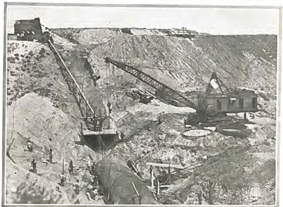
Showing Equipment Layout on U. S. Reclamation Service Siphon Project near Riverton, Wyo.
