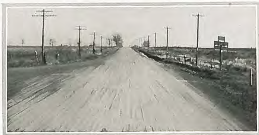
Last word in Maintenance—stretch of road between Ordway and Olney Springs on gravel surfaced Kansas-Colorado Boulevard
