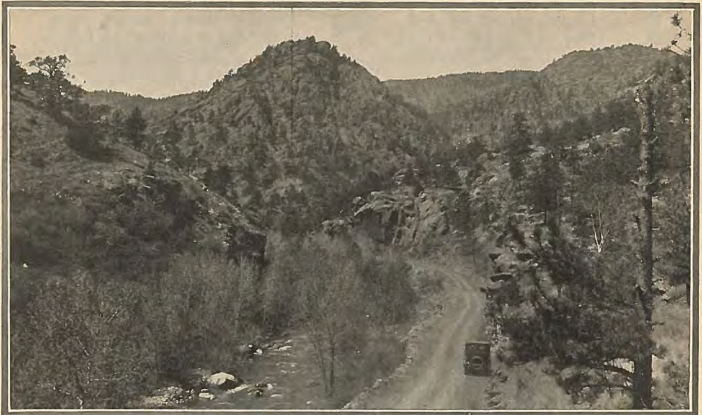
Boulder county is justly proud of its road in the South St. Vrain Canon, which has been practically completed to Allens Park. The above picture is a glimpse of the road four miles above Lyons. Photo by H. E. Link, Longmont.
