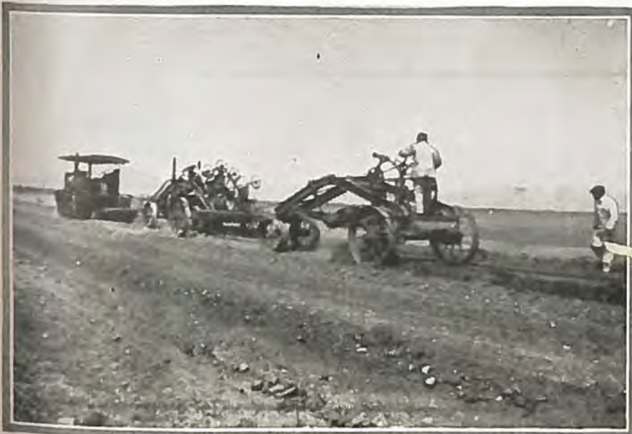
Tractor-grader outfit used on road construction in Alamosa county.
