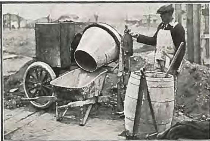
Stewart B-3 Trailer on the job
