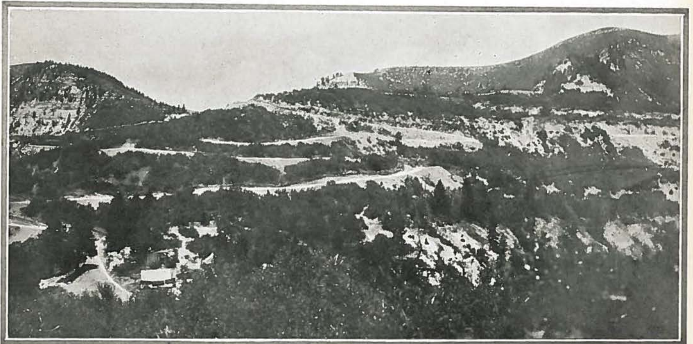
South side of Douglas Pass, showing switch-backs, on new highway being constructed by State Highway Department into the Uintah Basin, one of the largest undeveloped sections of the United States.
