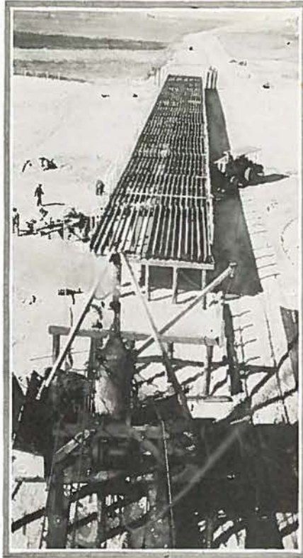
Picture taken from top of pile driver, looking west
