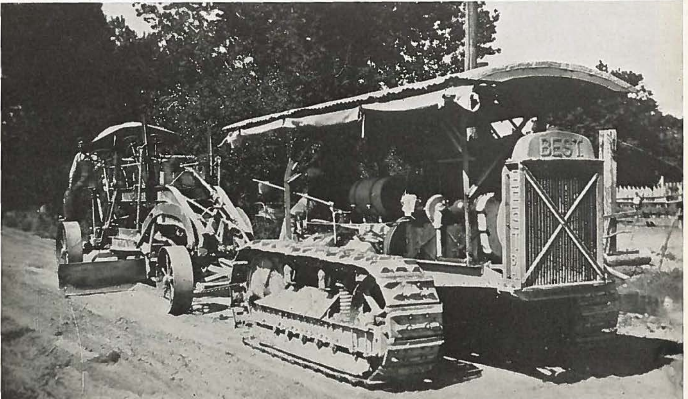
Large type Best tractor and grader working a Pueblo county road. This equipment turns out a mile of graded road each day.
