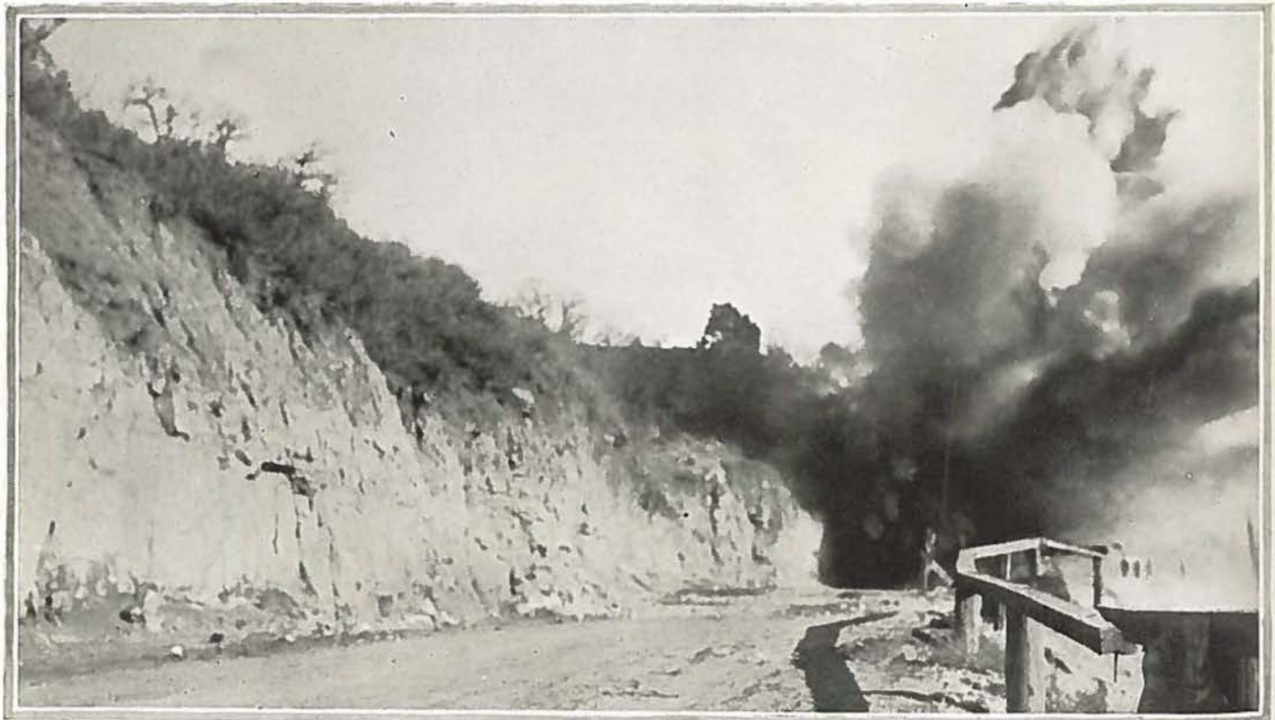
Modern road-making—showing the effect of the explosion of a ton of T. N. T. used by the El Paso County road crew, under Supt. H. A. Cudger, in blasting out a narrow portion of the North and South Highway near Pike View, four miles north of Colorado Springs. Photo by courtesy Pike's Peak News Bureau.
