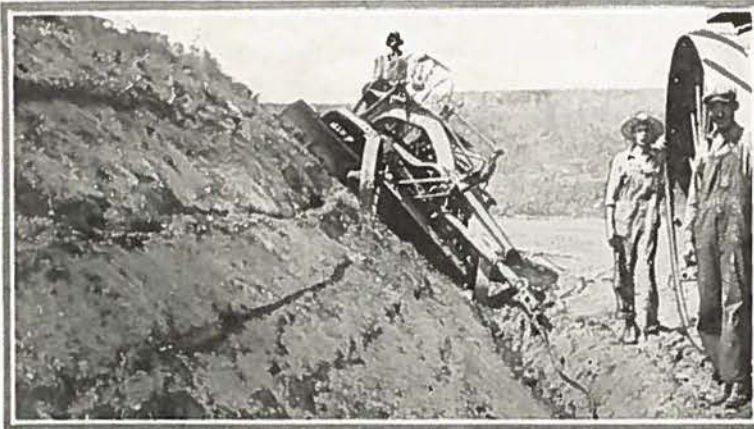
Cutting back a steep bank with 12 ft. Adams Grader riding upon the bank. Illustrates extreme work made possible by Leaning Wheels. Name of contractor on request.
