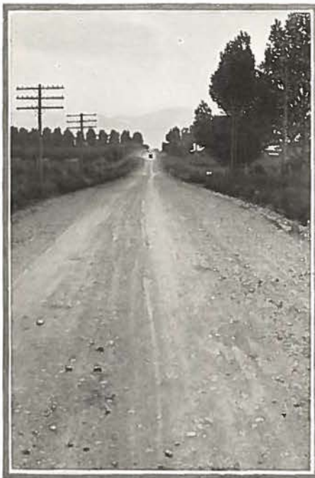
Gravel surfacing on this road by Colorado farmers
