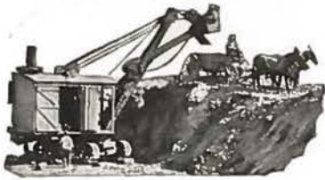
High Lift for Excavation Work
