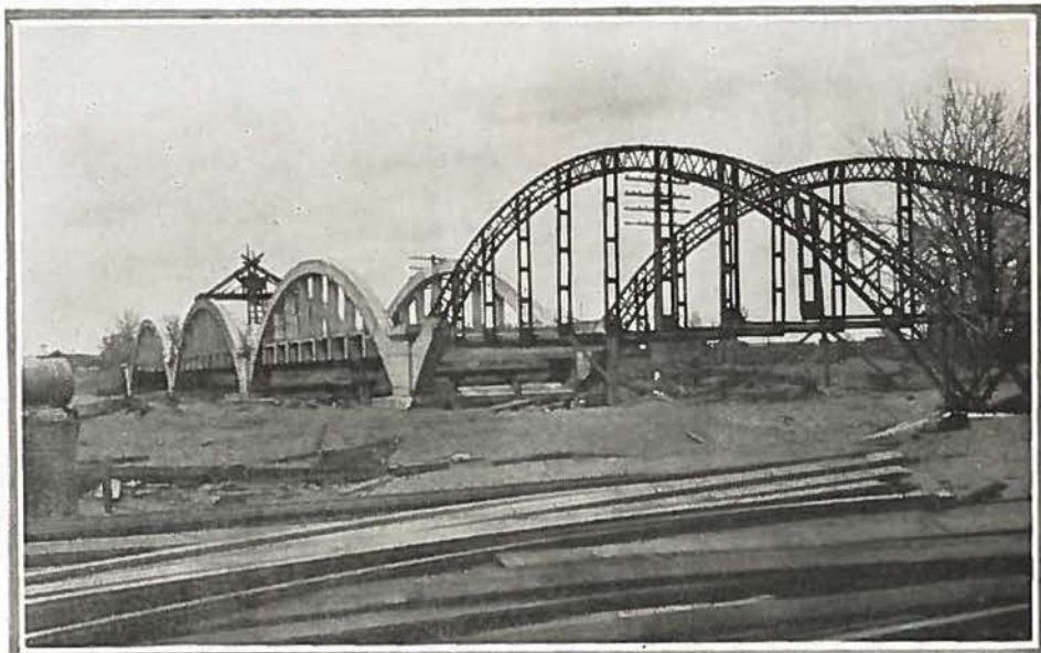
General view of partially completed bridge
