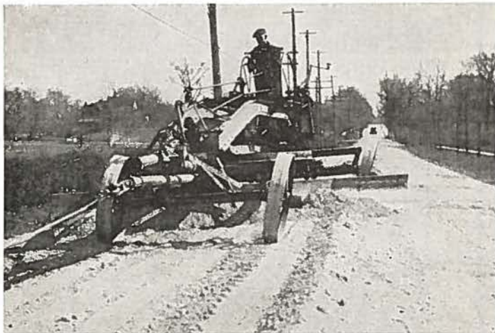
Twelve ft. machine with Blade Extensions which lengthen the blade to 18 ft. One round trip covers the road, doing the job smoothly and thoroughly.
