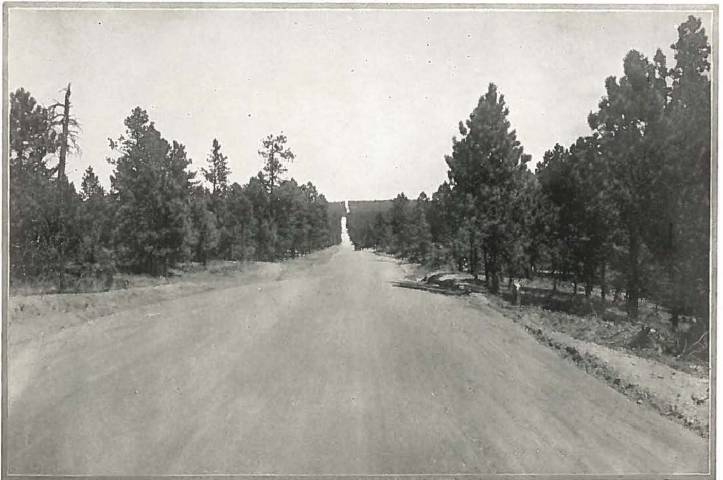
View of new road constructed through the Black Forest northeast of Colorado Springs, forming a new connecting link with Denver
