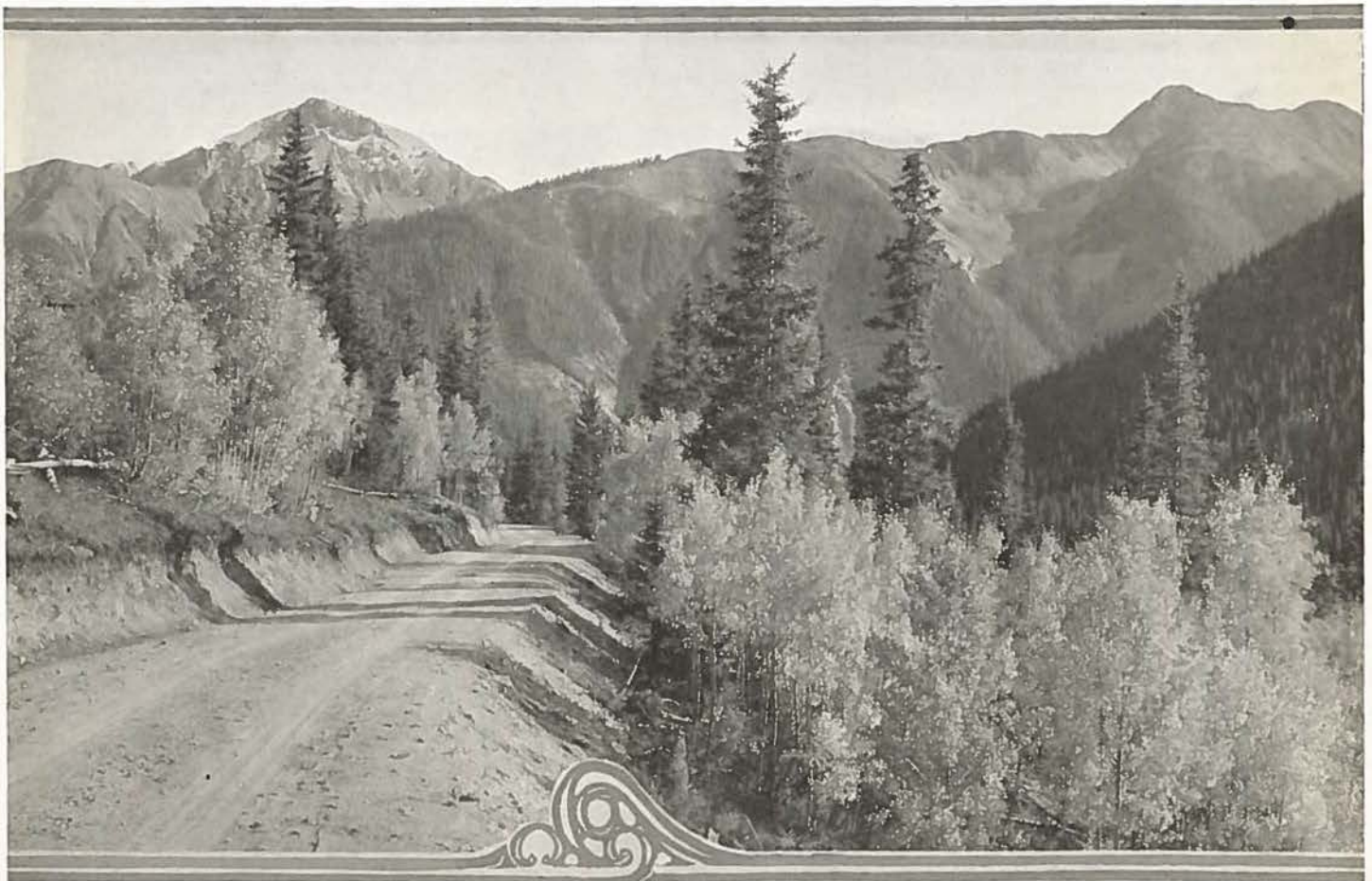
Scene on the southern slope of Red Mountain Pass, showing type of roads being constructed by the State in co-operation with the U. S. Forest Service.
