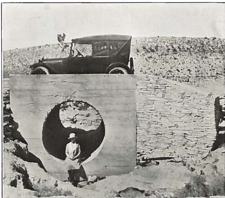
Six Foot Culvert on State Highway in Pueblo County Installed 1911
