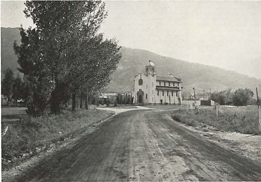
“Pauline Chapel” Adjacent to the Home of Spencer Penrose at Colorado Springs, Showing Road Made Mudless and Dustless With
