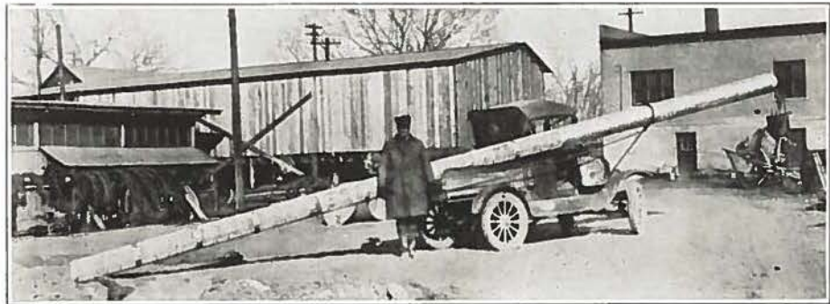
Well-Casing 11 in. diam. by 34 feet
