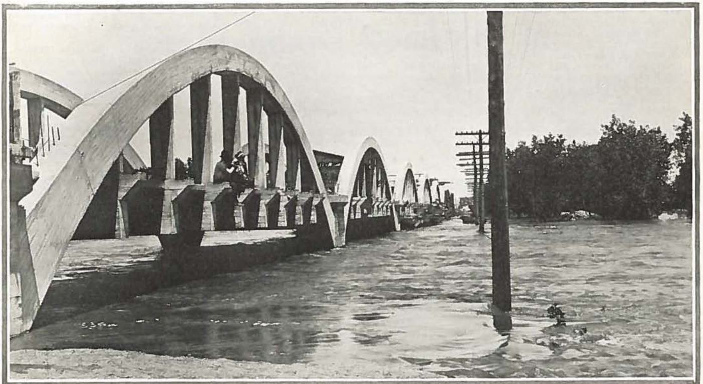
Fort Morgan bridge during recent flood in Platte river showing 5-foot clearance above water.
