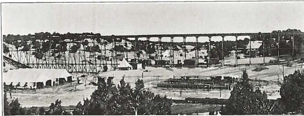
Flume No. 108 5 ft., 9 in. diameter
