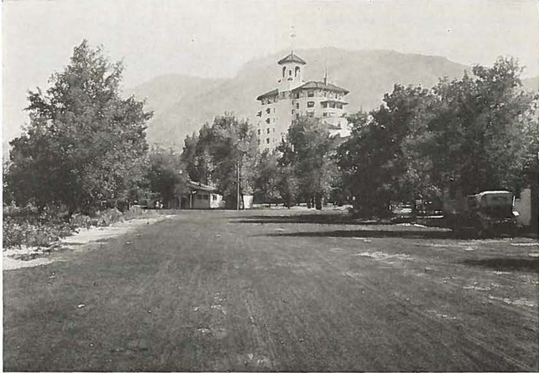
Oiled Road in vicinity of Broadmoor Hotel at Colorado Springs Made Mudless and Dustless with
