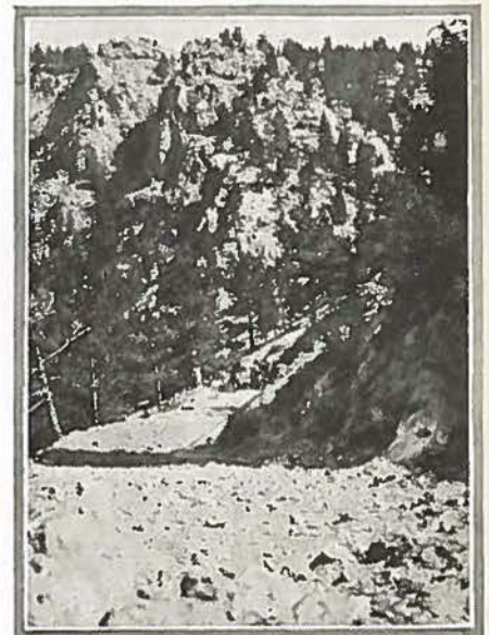
Heavy rock work on Bennett Creek Road
