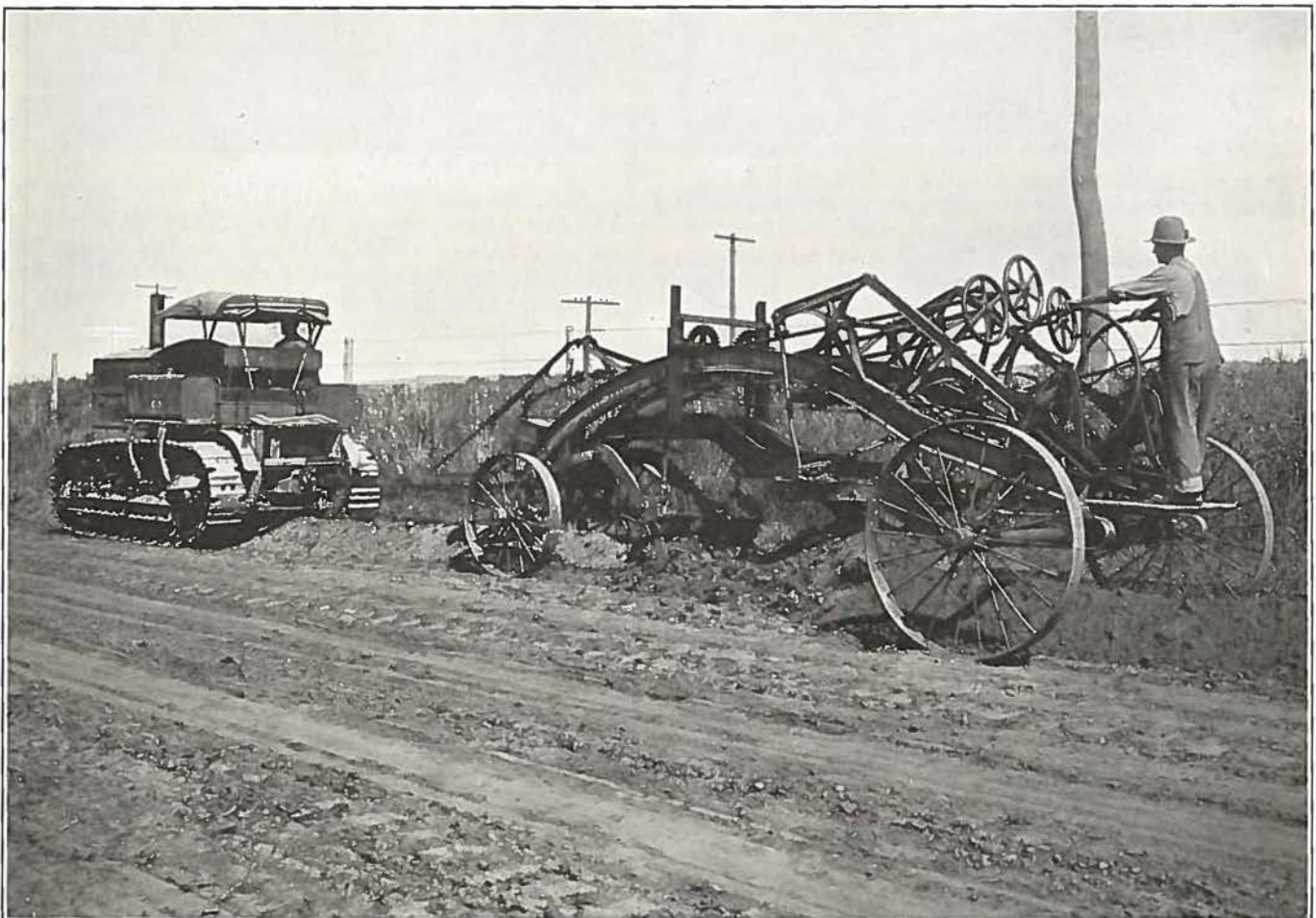
A maintenance outfit in action on one of Colorado's main roads.
