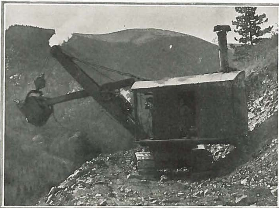
Roosting on the corner of "eternity", chewing away a new 25-foot roadway at the foot of Berthoud Pass, one of Colorado's famous mountain boulevards. State Highway forces are now engaged in constructing an extension of this road between Empire and Lawson. Photo by U. S. Bureau of Public Roads.
