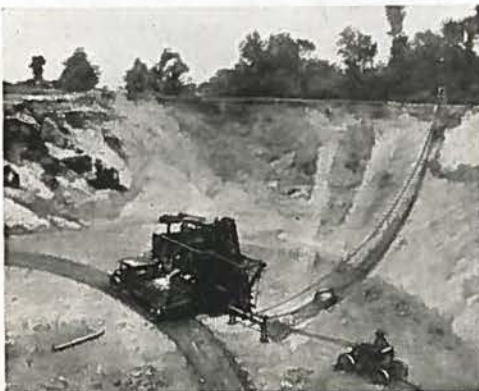
Excavating Gravel for a Highway job with a ½ yard Sauerman Portable Power Scraper.
