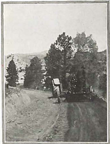
A grader in action on road in Colorado National Forest
