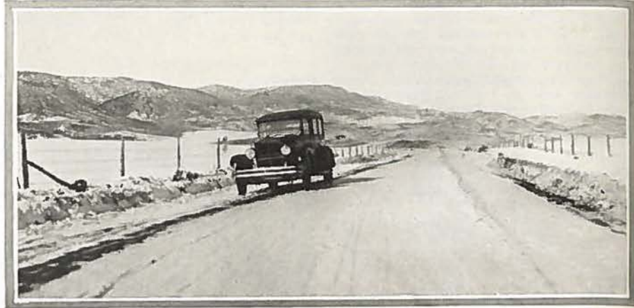
Scene on Rifle-Meeker Highway—Showing Result of Maintenance Work.
