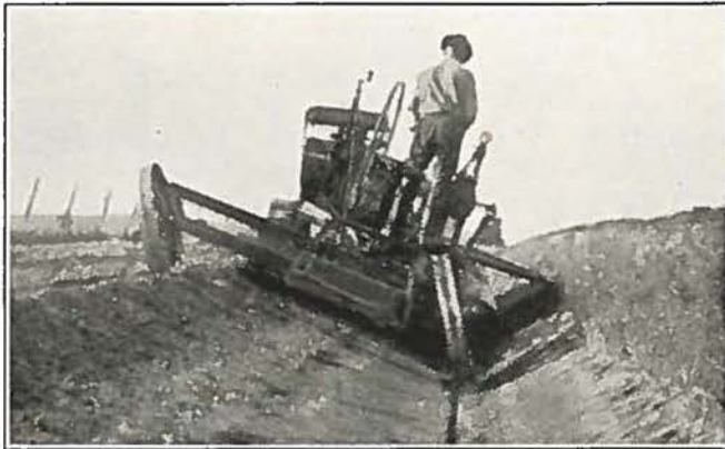
Perfect back-sloped and flat bottom ditch cut with Adams Back-Sloper Attachments
