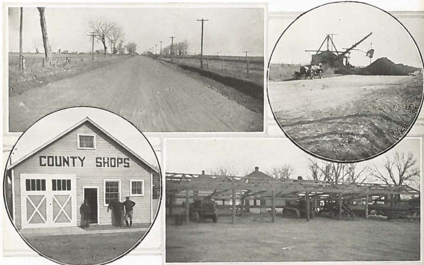
Top circle—Grading state highway with dirt excavated from Ordway drainage ditch; when completed will be 30 ft. wide and will cost state and county about 2\frac{1}{4} cents per yard. Top left—Portion of Kansas-Colorado boulevard between Sugar City and Ordway recently completed with gravel surfacing. Bottom circle—Front of Crowley county highway shops in Ordway. Bottom right—Machinery shed ready for roof and siding.
