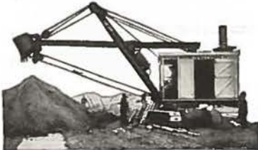
Steam Hoe for Trench Work
