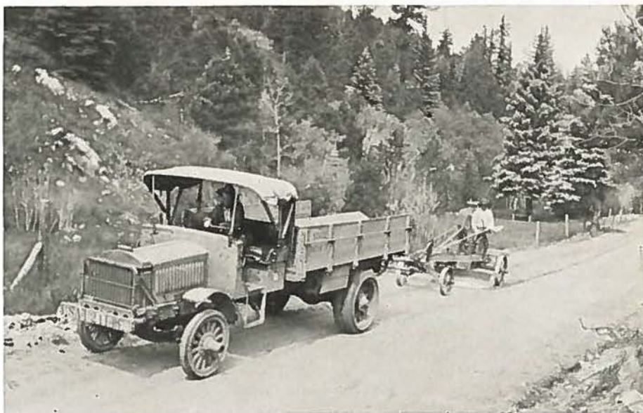
Jefferson County Maintenance Crew Working on State Highway Through Turkey Creek Canon.
