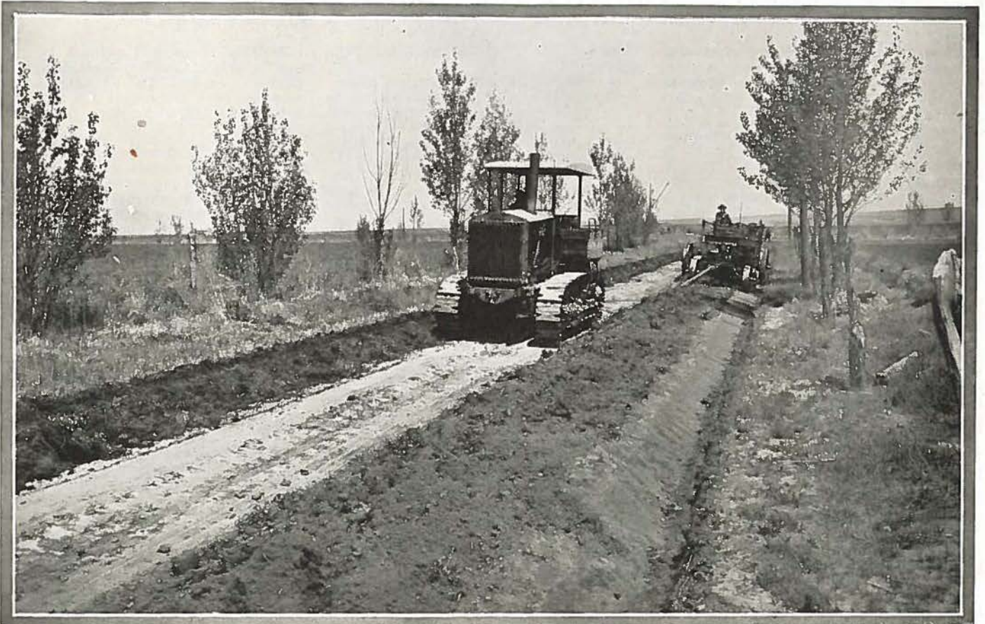
Showing how El Paso county is economically building roads with a ten-ton Holt tractor furnished by the U. S. Government from surplus war stocks, supplemented with a modern large type Stockland grader. With this combination outfit one mile of modern roadway can be constructed in a day.
