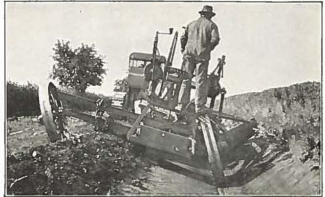
Perfect back-sloped, flat-bottom ditch cut by Adams Grader with backsloper attachment.
