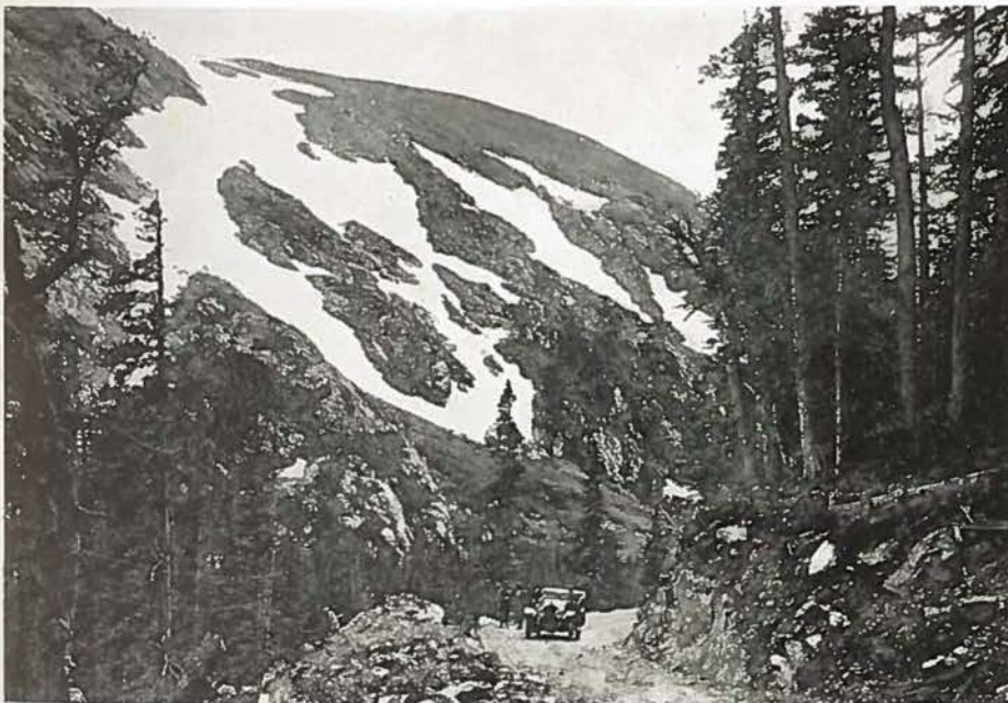
Fall River road in the Rocky Mountain National Park, constructed by the Colorado State Highway Department.
