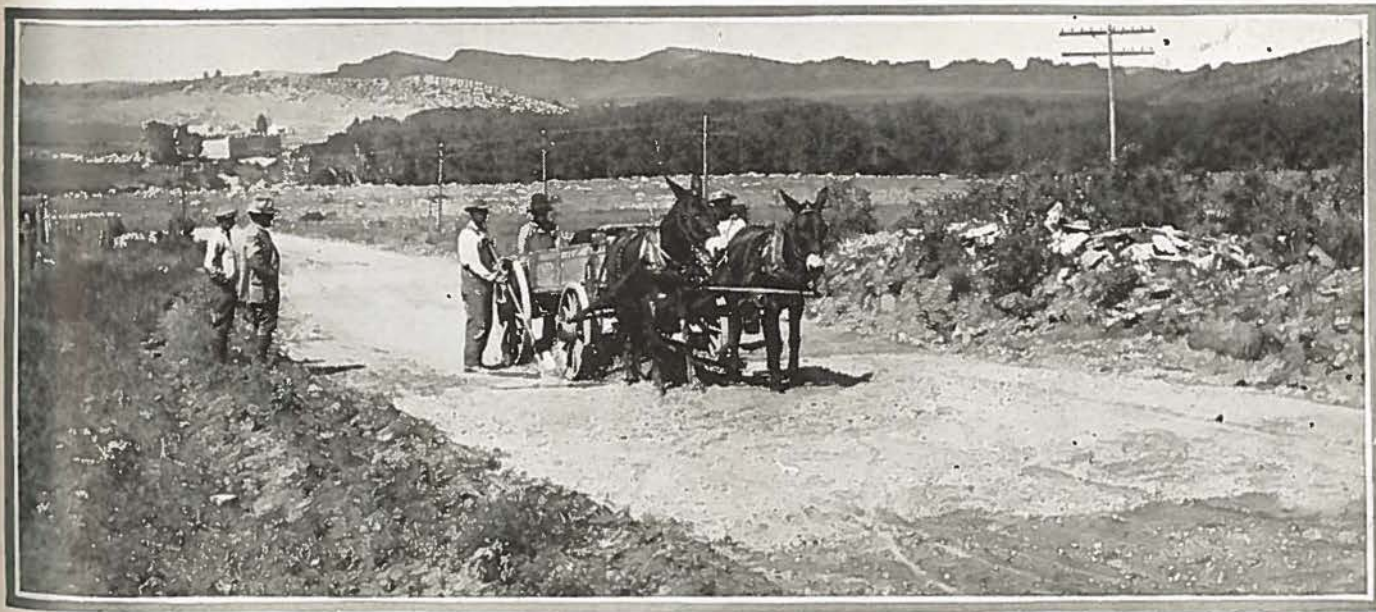
Farmer team unloading gravel on Northern Colorado road.
