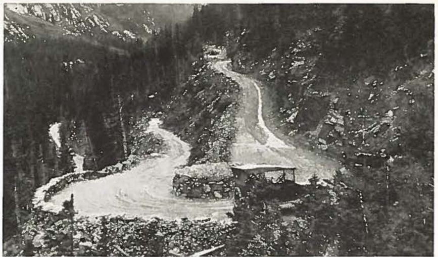
Scene on Fall River Road near Grand Lake, showing water being drained from surface of road by means of open top culverts.
