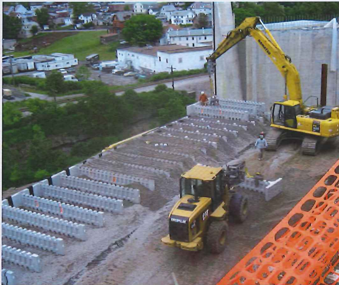
T-WALL® units being lowered into place
