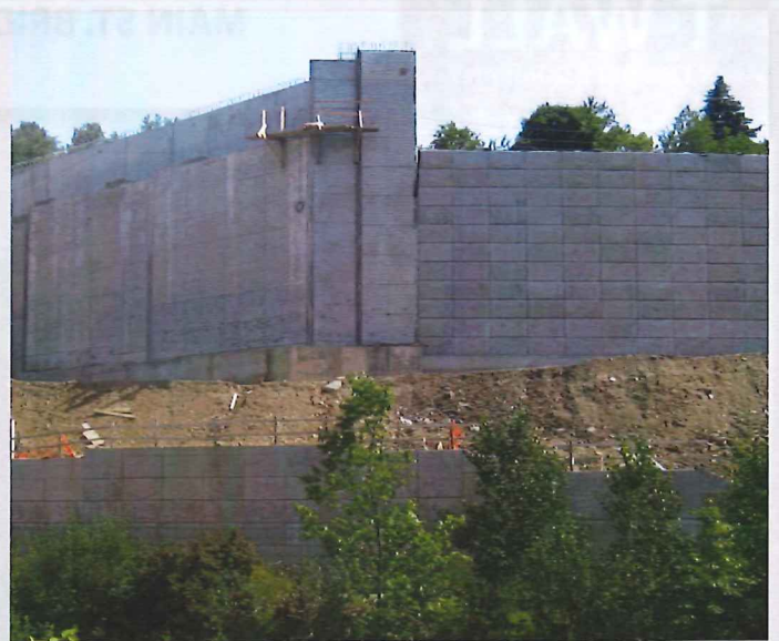
Crash wall and partially completed bridge approach
