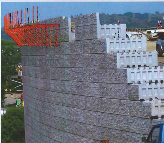
Partially completed bridge approach
