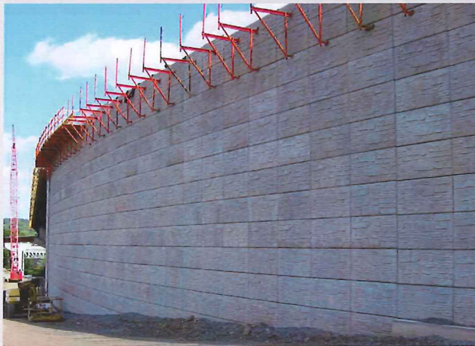
Partially completed bridge approach
