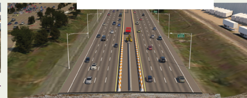
This MOT concept first reconstructs the median barrier to allow for early relocation of the ITS backbone outside of the roadway, as well as installing new permanent lighting in the median to replace the existing lighting that lines much of the 4.5-mile corridor.
