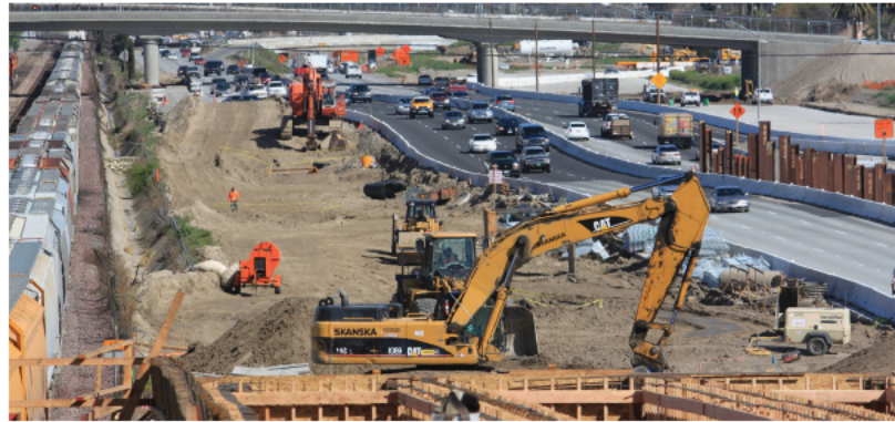
Figure 5.07 | Positive protection: Provided between long-term construction activities and vehicles traveling Central 70.
