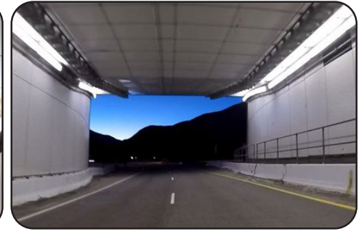
Image 12. West Facing View and Lighting of the Johnson Memorial Tunnel
