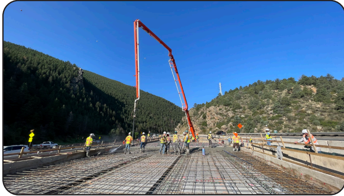
Image 33. Deck Pour of the Temporary Floyd Hill Bridge
