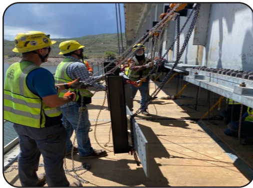
Image 5. Repair Plate Installation
