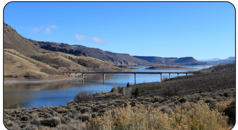
Image 9. Blue Mesa Bridges and Reservoir
