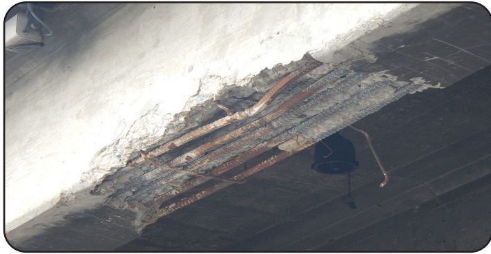
Image 36. Impact Damage on US 50 ML over I-25 ML (K-18-J)
