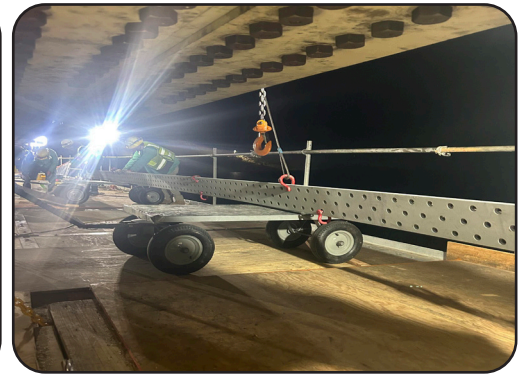
Image 7. Crack Arrest Plate Positioning
