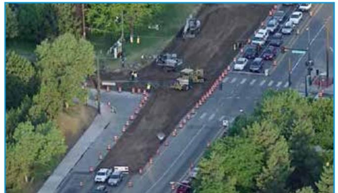
Taken just before the morning rush hour, this photo of Colorado Boulevard and Hampden Avenue resurfacing highlights the large work areas that are possible with an aggressive phasing approach (17 days). CDOT received positive feedback for the quick work at this congested city intersection.
