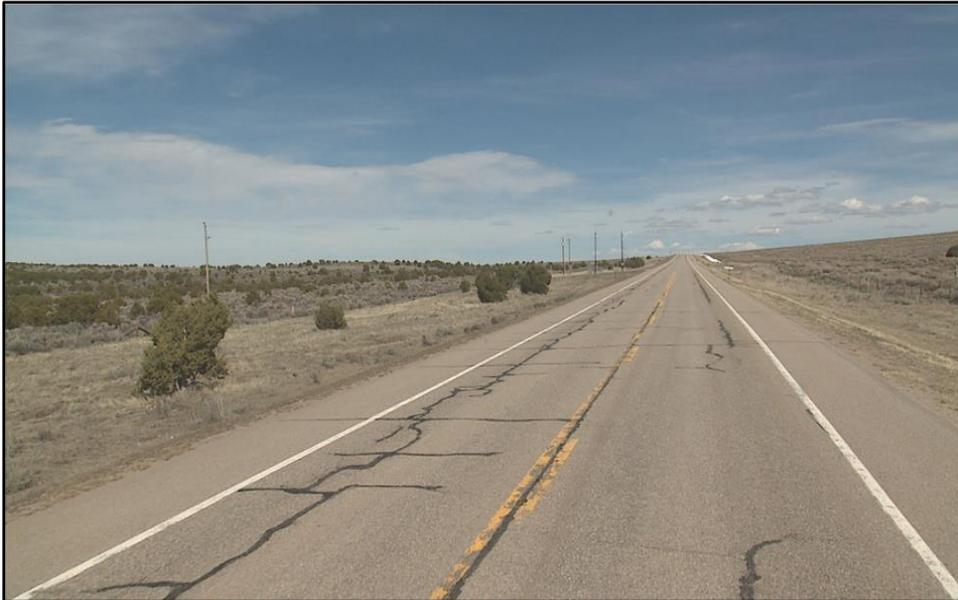
*State Highway 40 east of Elk Springs. This pavement was rehabilitated in 1999. It is a Moderate Drivability Life road, which is exceeding its design expectations. Preservation techniques, such as crack sealing and chip sealing, keep this pavement from deteriorating.*
