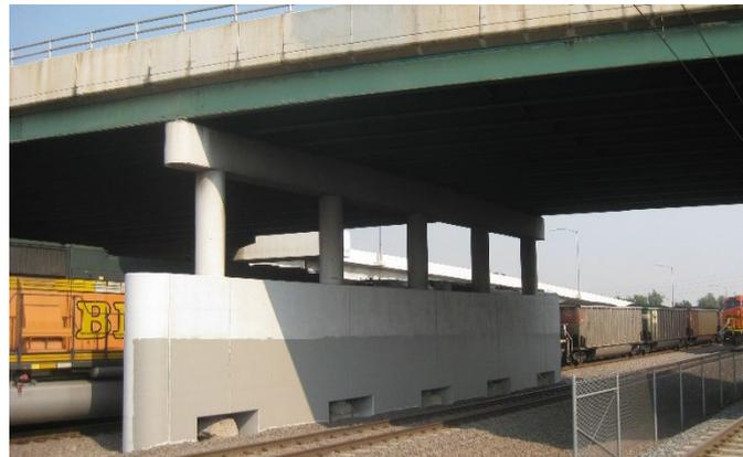
**For Highway Underpass Structures**, horizontal clearances vary depending on the railroad, curvature of track, future tracks, access roads, and other issues that need to be investigated with the railroads before beginning design. Design must also meet PUC minimum requirements.
