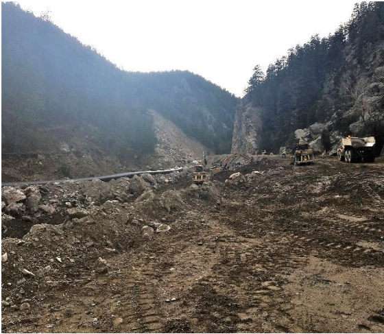
Photo 17.3 Construction of a matrix riprap revetment along the Big Thompson River on US 34, Larimer County, Colorado, near MP 72.
