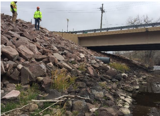
Photo 17.1 Rock riprap treatment along US 287 on the bank of the Cache la Poudre River in Larimer County, Colorado.
