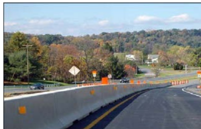
JJ Hooks Concrete Barrier
