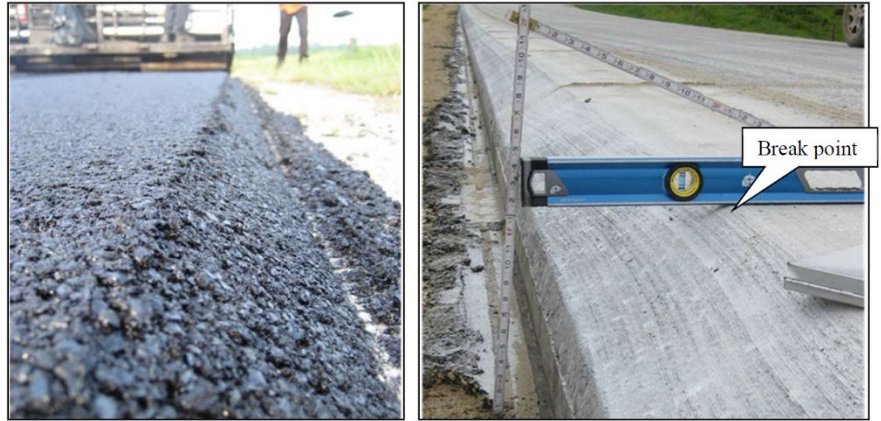
Figure 1. Safety Edge placed on AC and PCC
