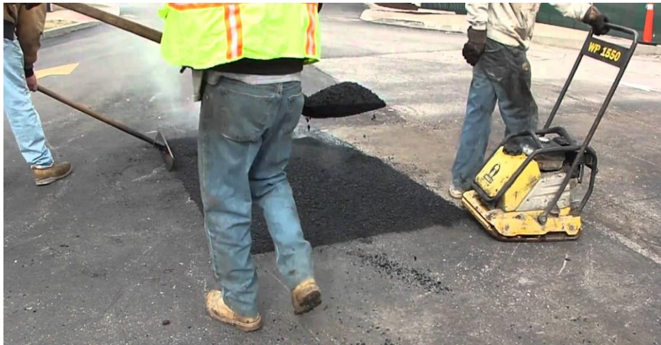
Figure 8.50 Photo of Manual Skin Patching
