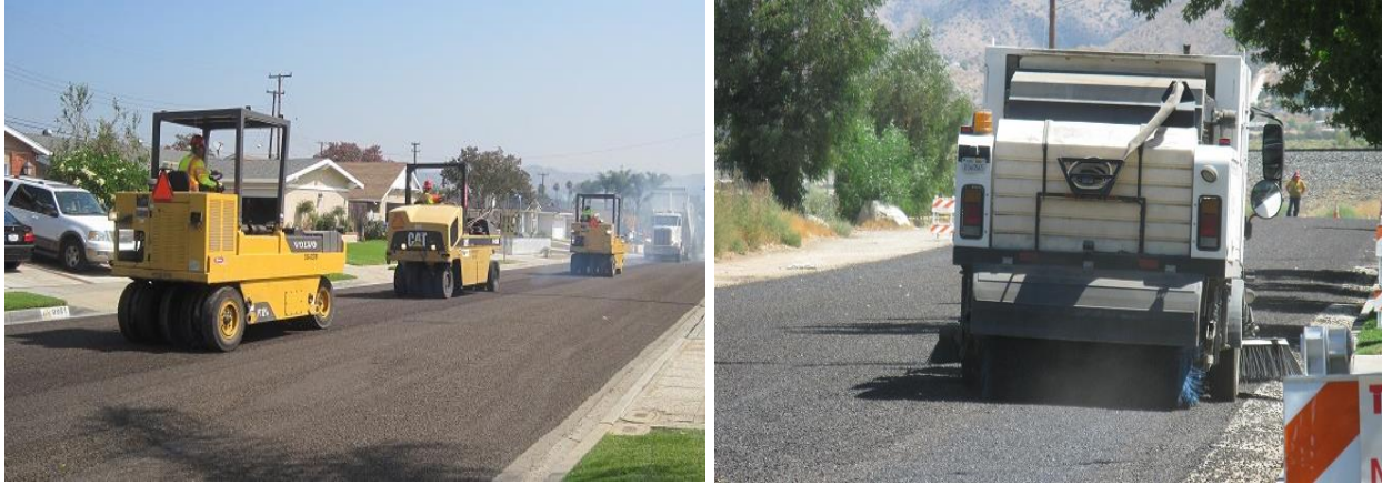
Figure 8.37 Photos Showing the Rolling and Sweeping After Chip Placement
