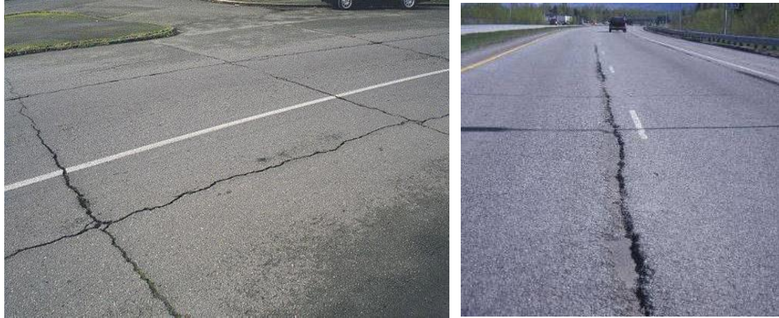
Figure 8.4 Photos of Longitudinal and Transverse Cracking
