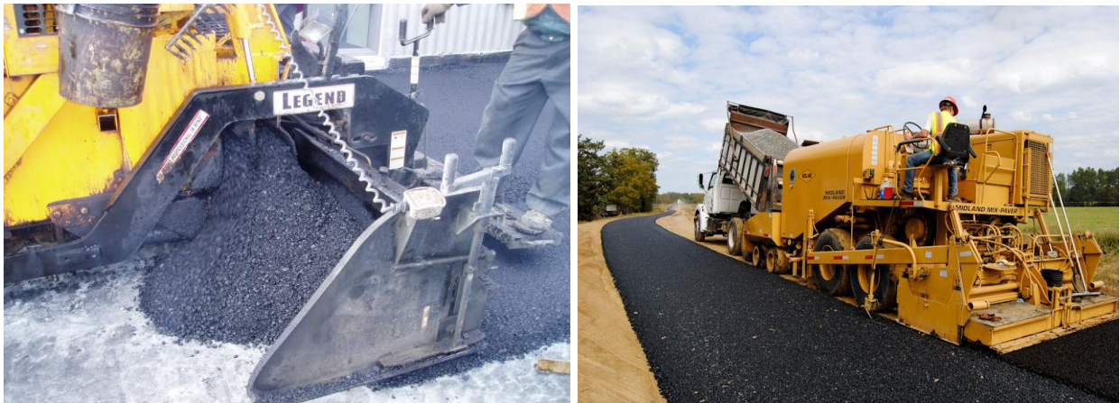
Figure 8.44 Photos of Cold Mix Paving
