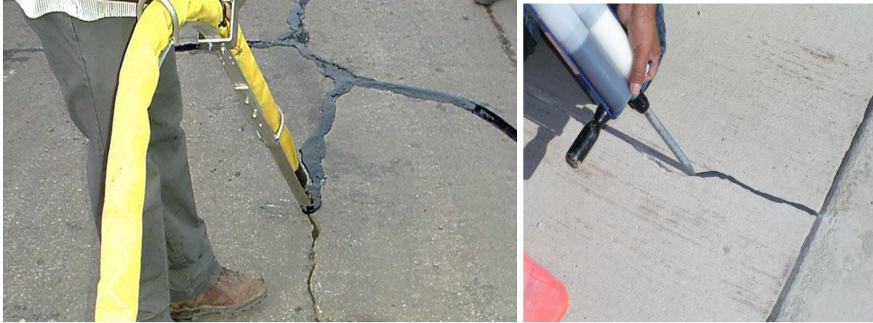
Figure 10.5 Photos of Crack Sealing
