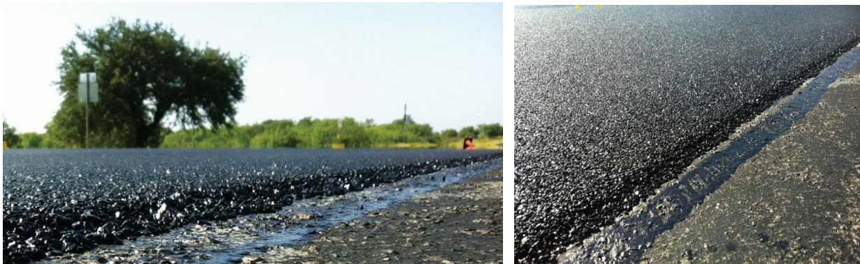
Figure 8.25 Photo of a Conventional HMA Overlay
