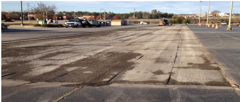
Figure 8.7 Photo of Milling of Old Asphalt
