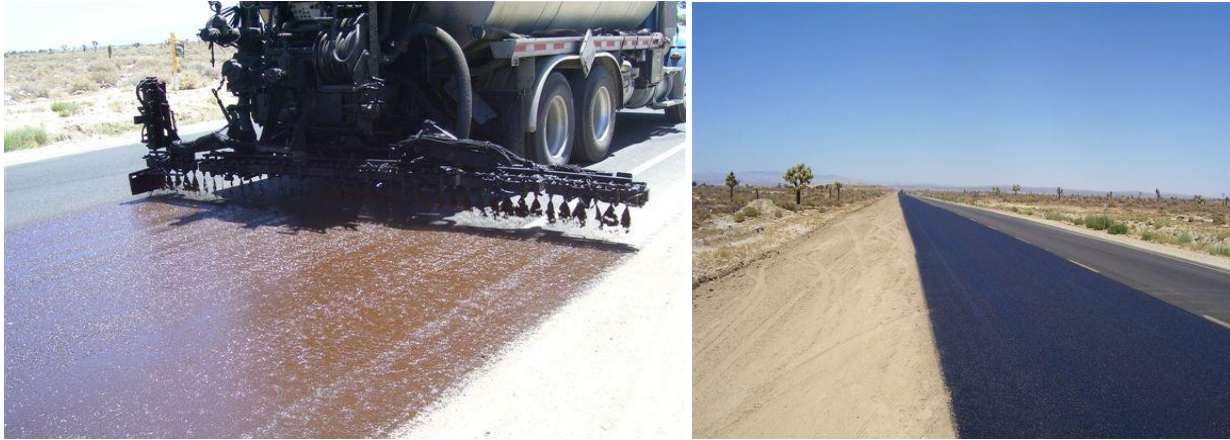
Figure 8.45 Photos Showing the Placing of a Fog Coat and the Final Result
