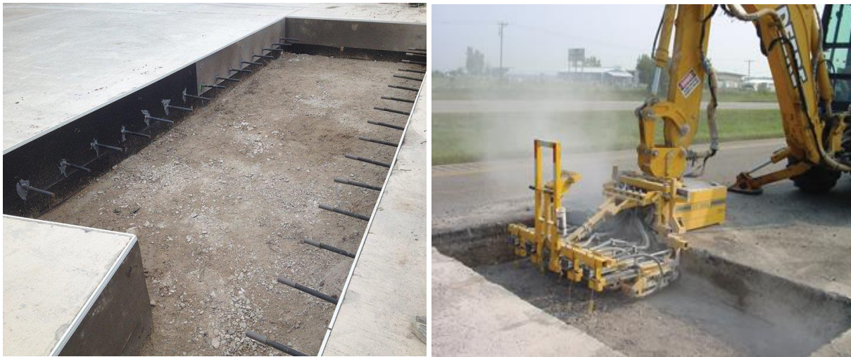
Figure 10.8 Photos of Full Depth Concrete Repair
