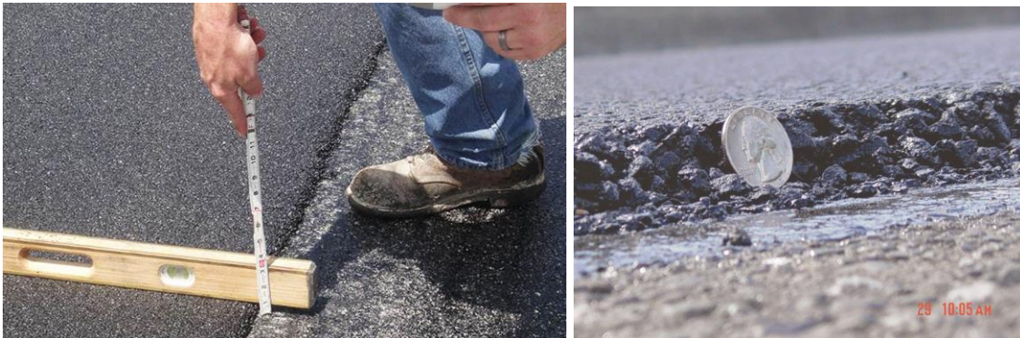
Figure 8.48 Photos of Ultra-Thin Asphalt Overlays
