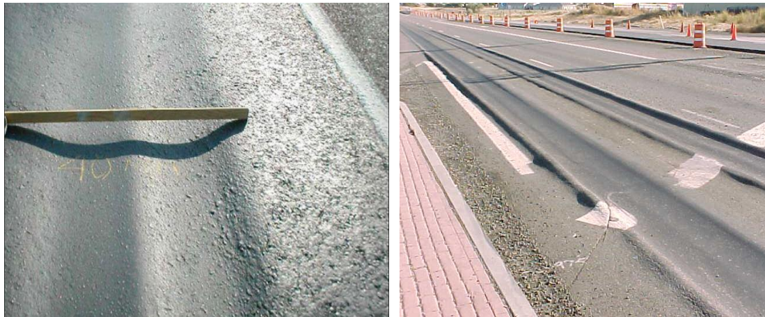
Figure 8.5 Photos of Rutting
