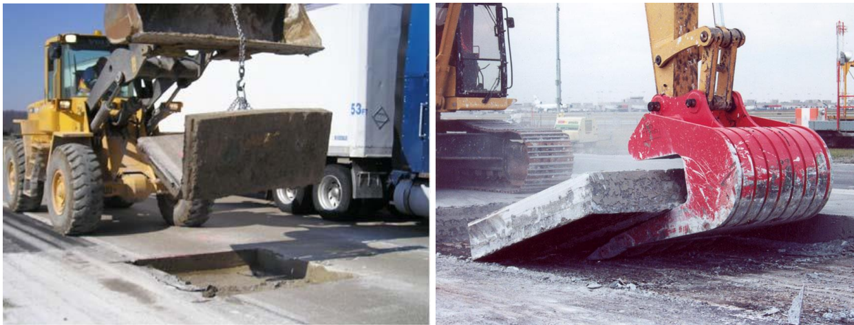
Figure 10.9 Photos of Concrete Slab Removal
