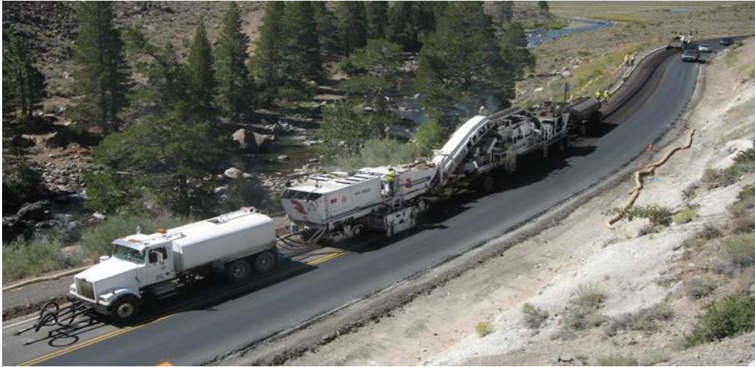
Figure 8.47 Photo Showing A Cold In-Place Recycling Operation
