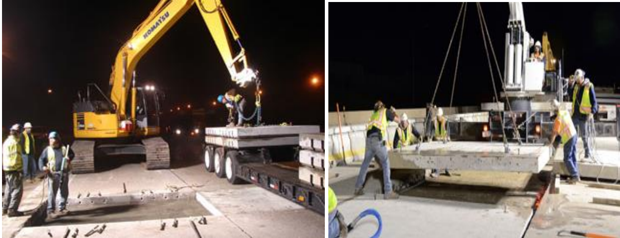
Figure 10.13 Photos of Precast Concrete Panel Repair
