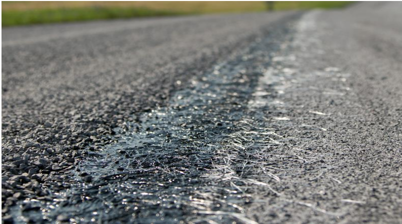
Figure 8.49 Photo Showing a Stress Absorbing Membrane
