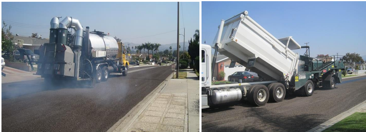
Figure 8.36 Photos Showing the Emulsion Spraying and Placing Chips
