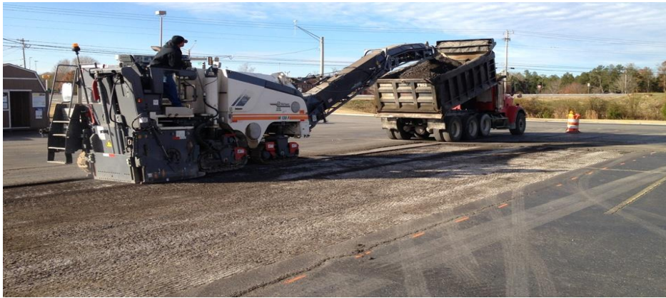
Figure 8.7 Photo of Milling of Old Asphalt
