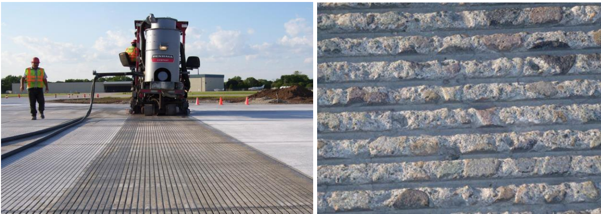
Figure 10.2 Photos of Diamond Grinding and Grooving
