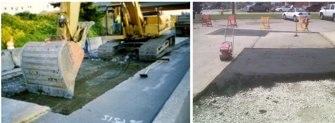
Figure 8.46 Photos Showing Various Stages of Full Depth Replacement Patching
