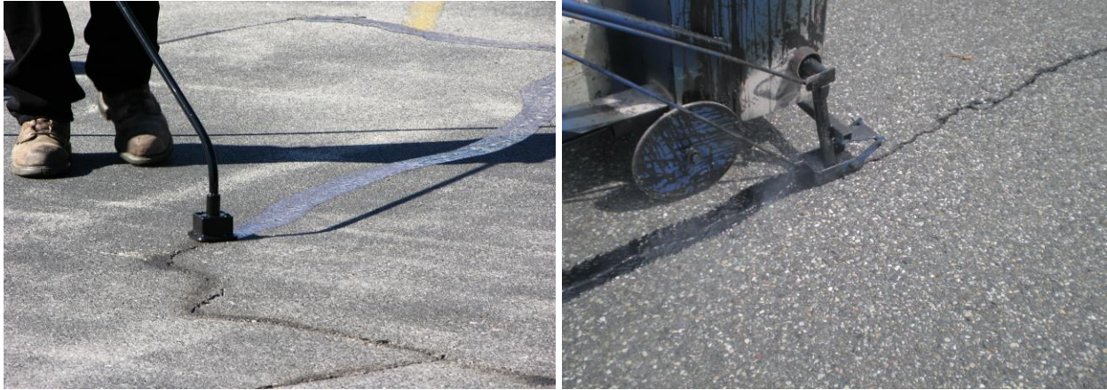
Figure 8.43 Photos Showing Crack Sealing
