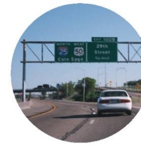
Freeway: Ground Level
