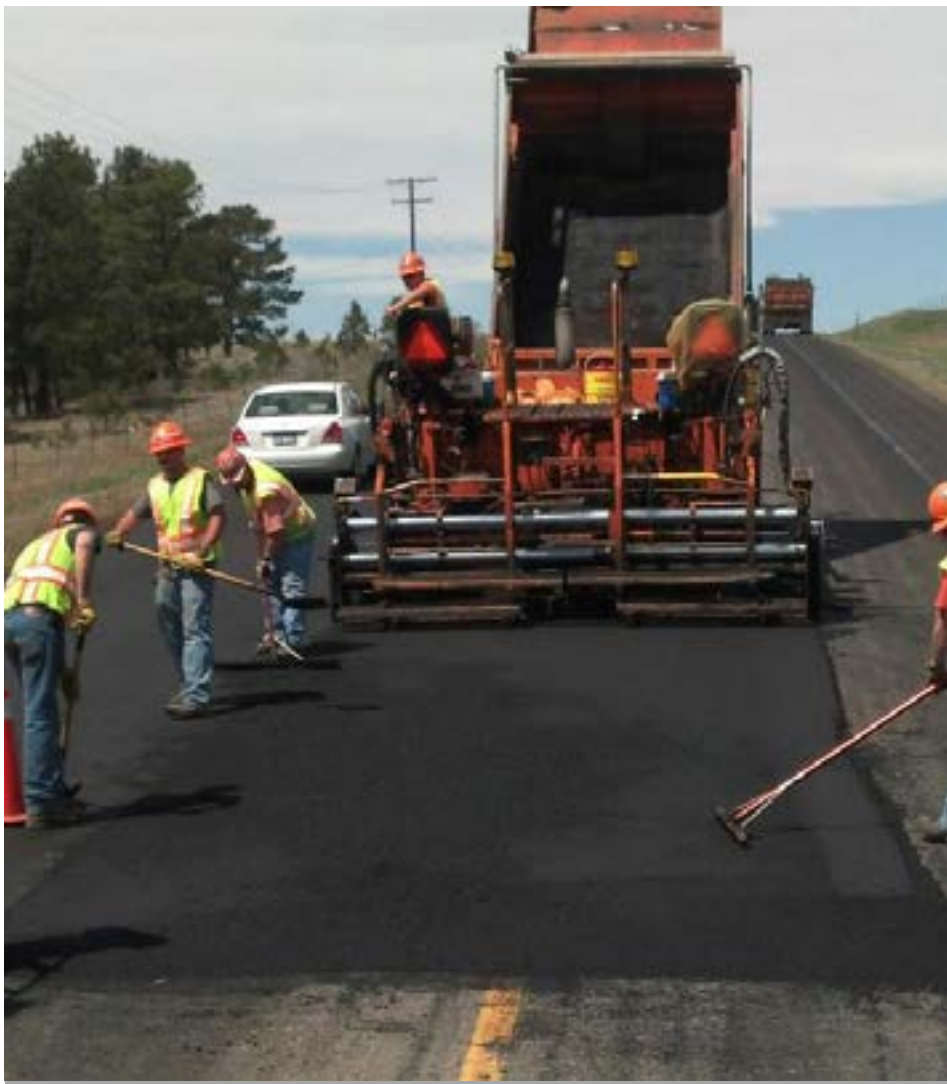
Construction on US 287 in Lamar.
