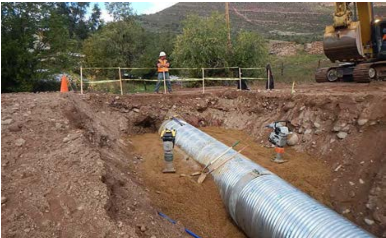
Figure 71 - MP 31.2, ER CMP Installation.
