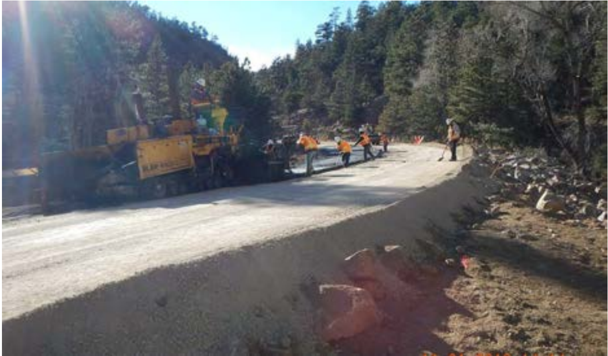
Figure 47 - MP 23.8 Facing west, Roadway repair.
