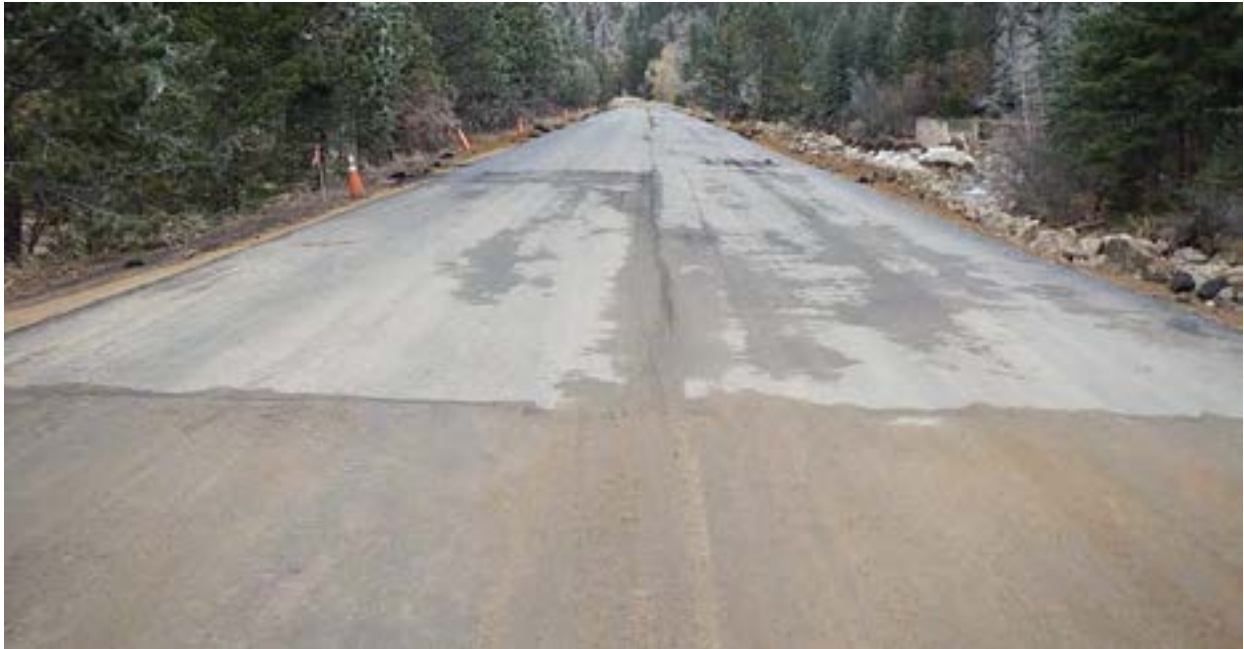
Figure 45 - MP 23.4 Facing east, Completed ER roadway section.
