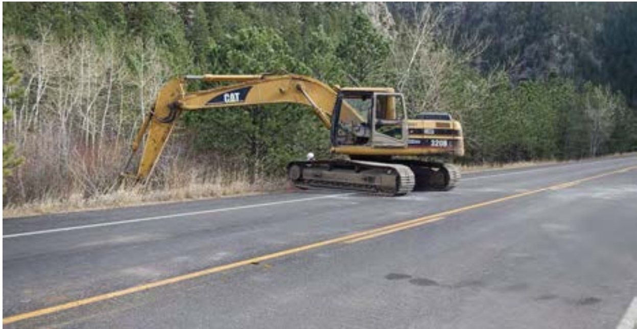
Figure 15 - MP 22, Emergency repair.
