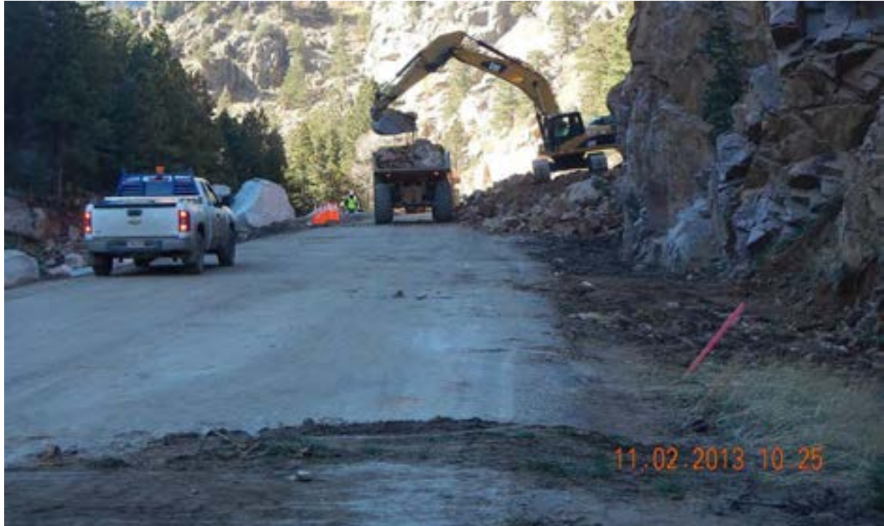
Figure 53 - MP 26.2 Facing west, Clearing rockfall.
