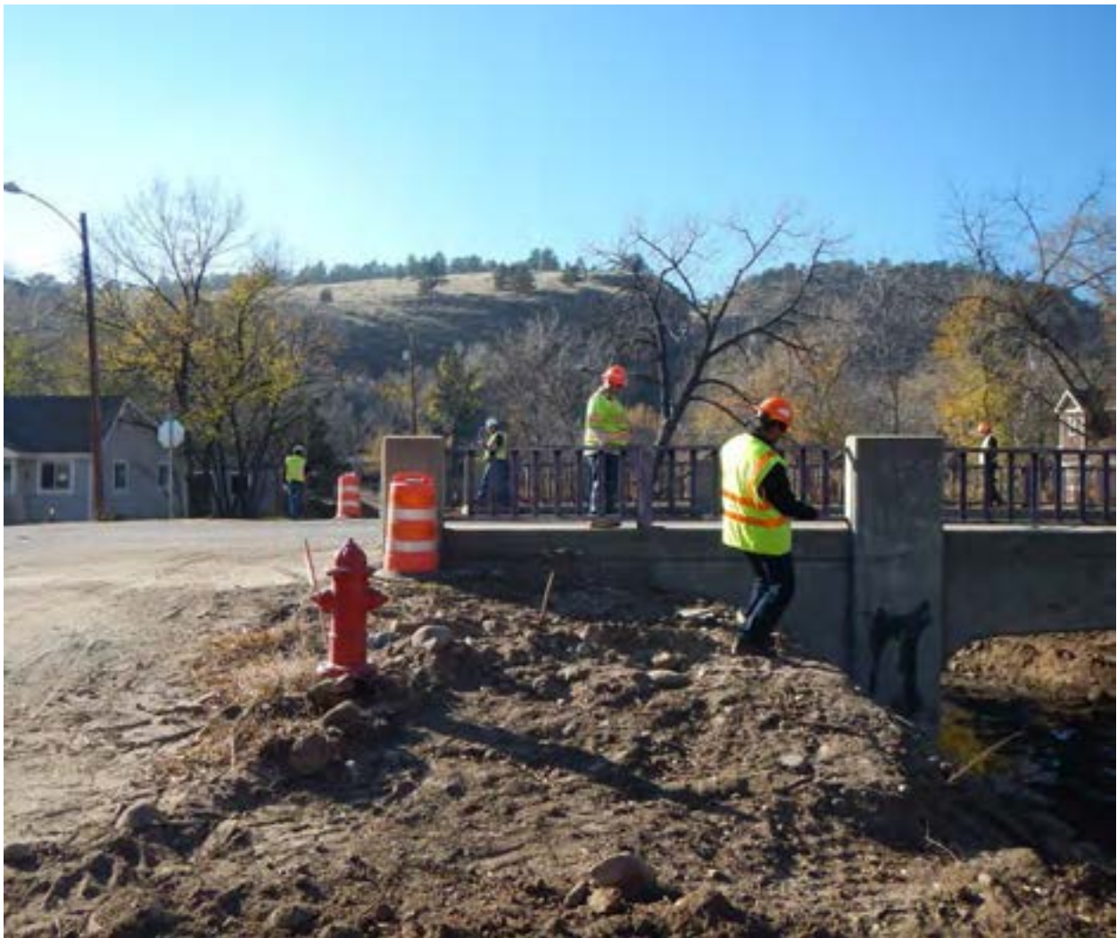
Figure 78 - MP 32.98, Facing west, Structure D-15-A embankment repair.
