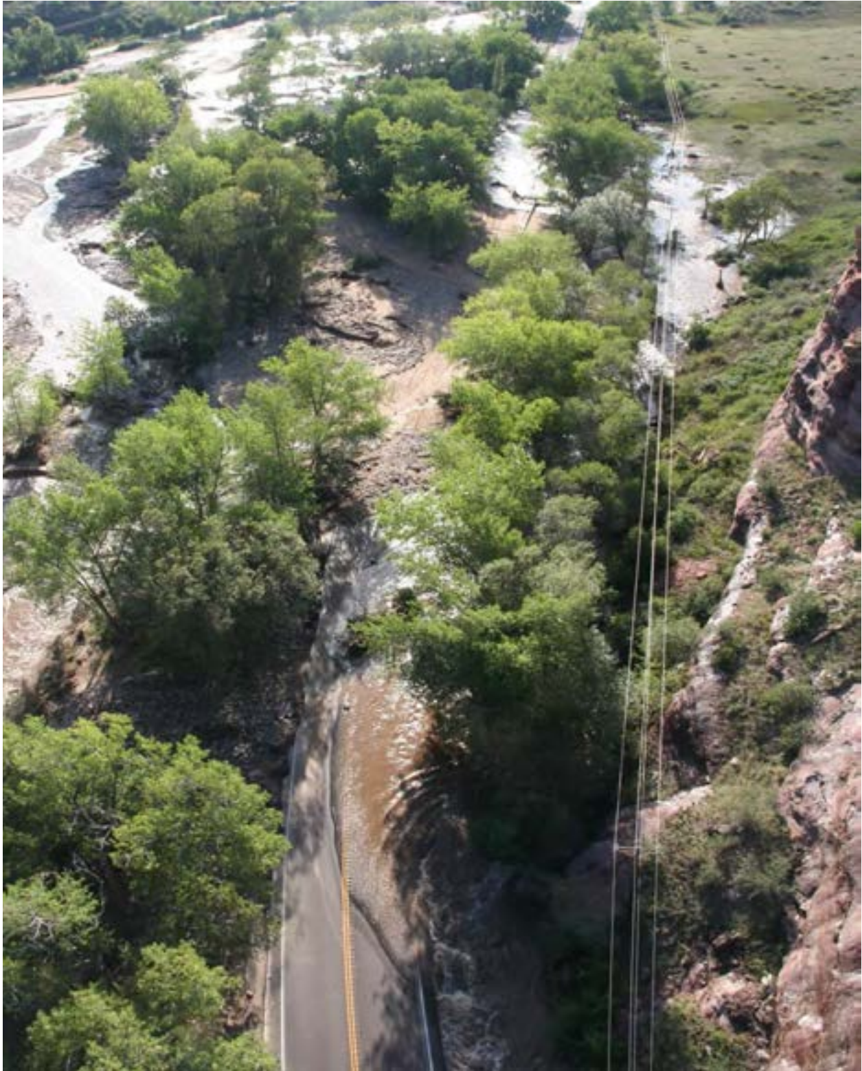
Figure 65 - MP 31.64, Roadway overtopped throughout section, shoulder and ditch washouts on both sides.
