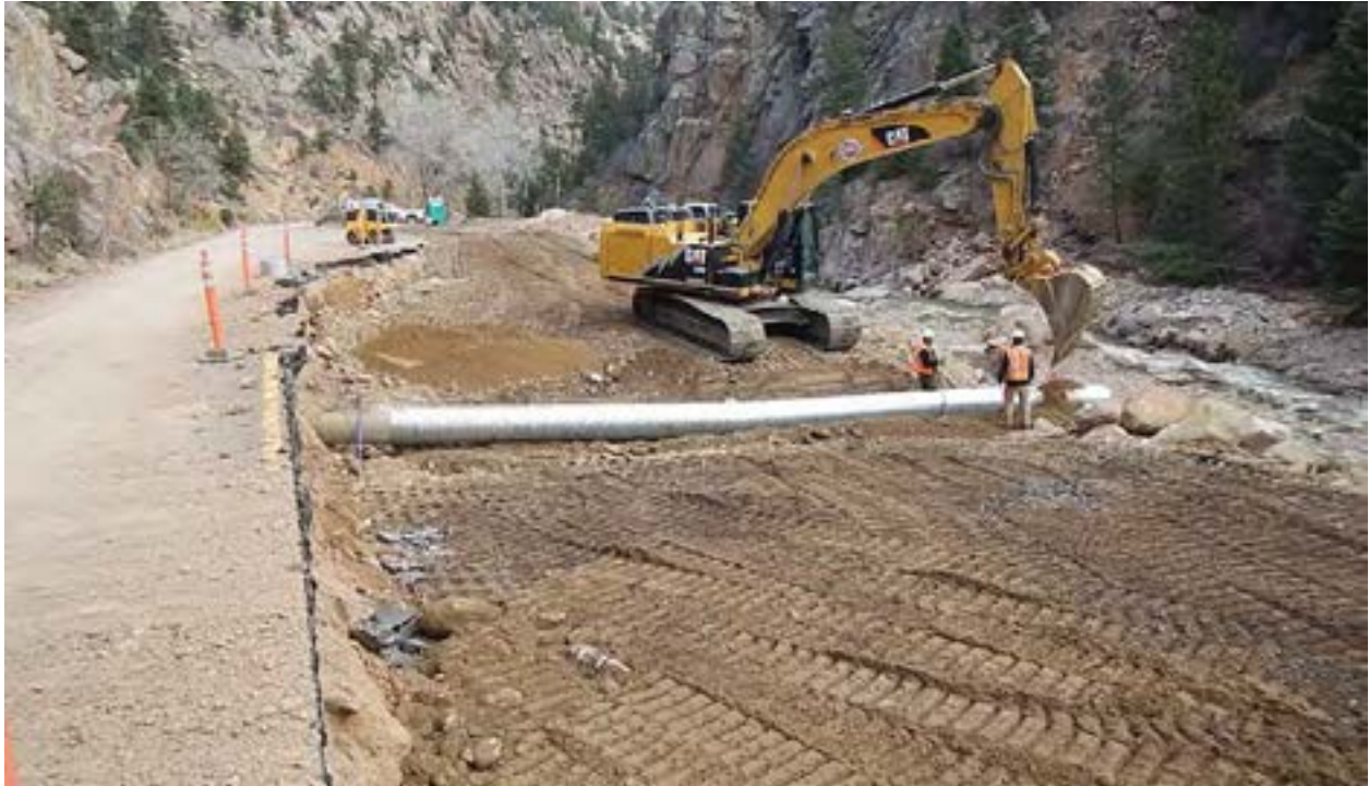
Figure 59 - MP 27.35, Facing North, Roadway and CMP repair.
