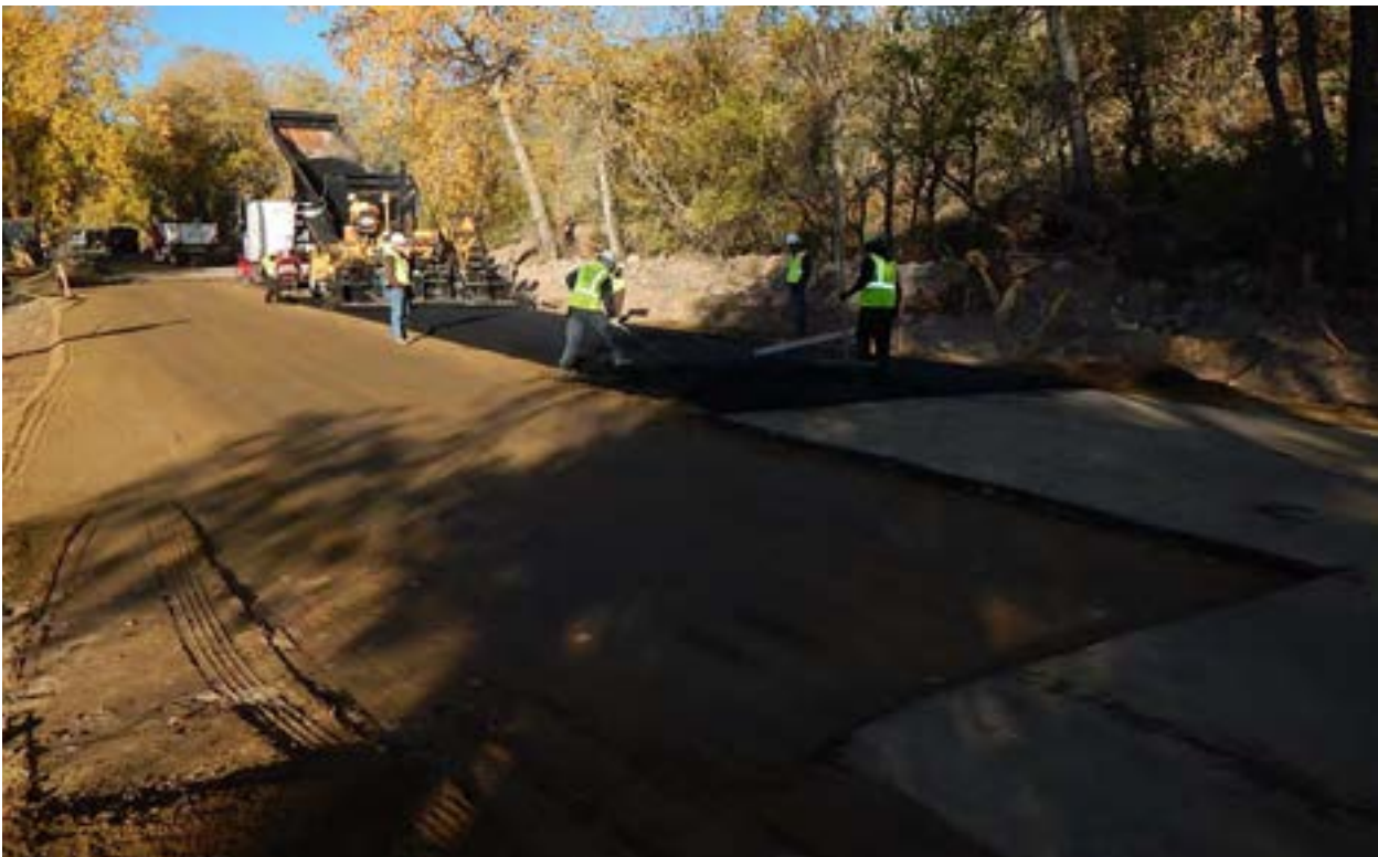
Figure 73 - MP 31.7, ER Paving operations.
