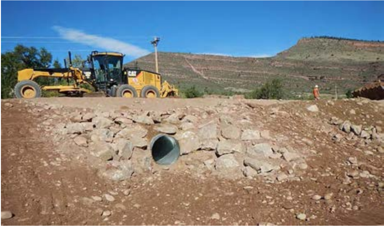
Figure 72 - MP 31.2, ER CMP installation complete.
