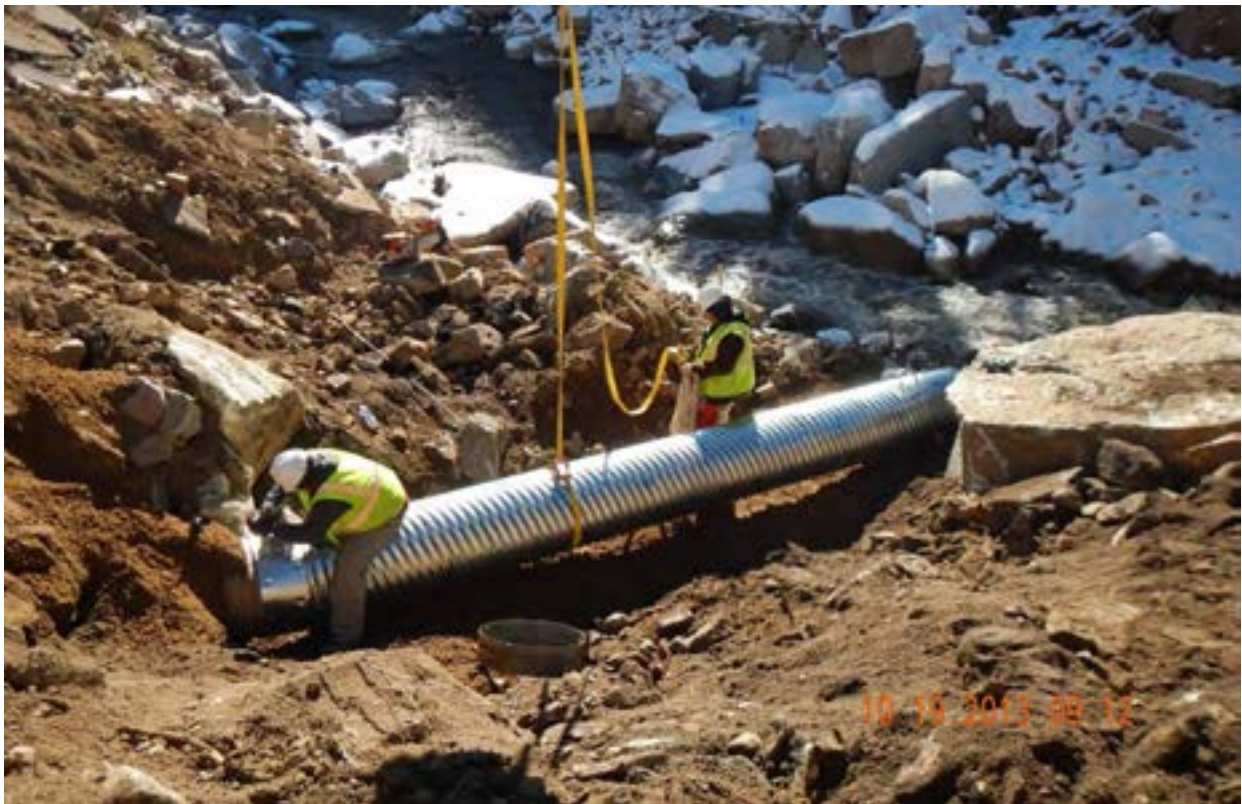
Figure 46 - MP 23.4, CMP repair.
