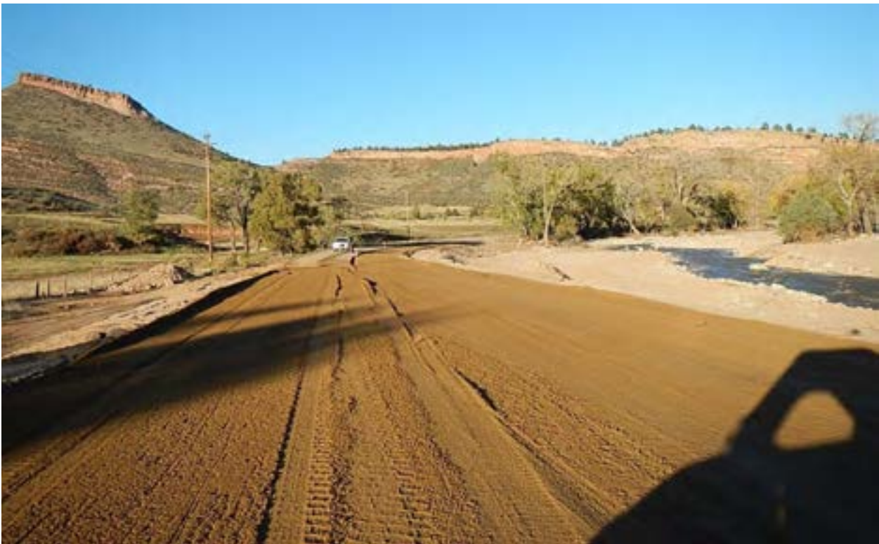
Figure 69 - MP 31.2, Facing northeast, ER Roadway repairs.
