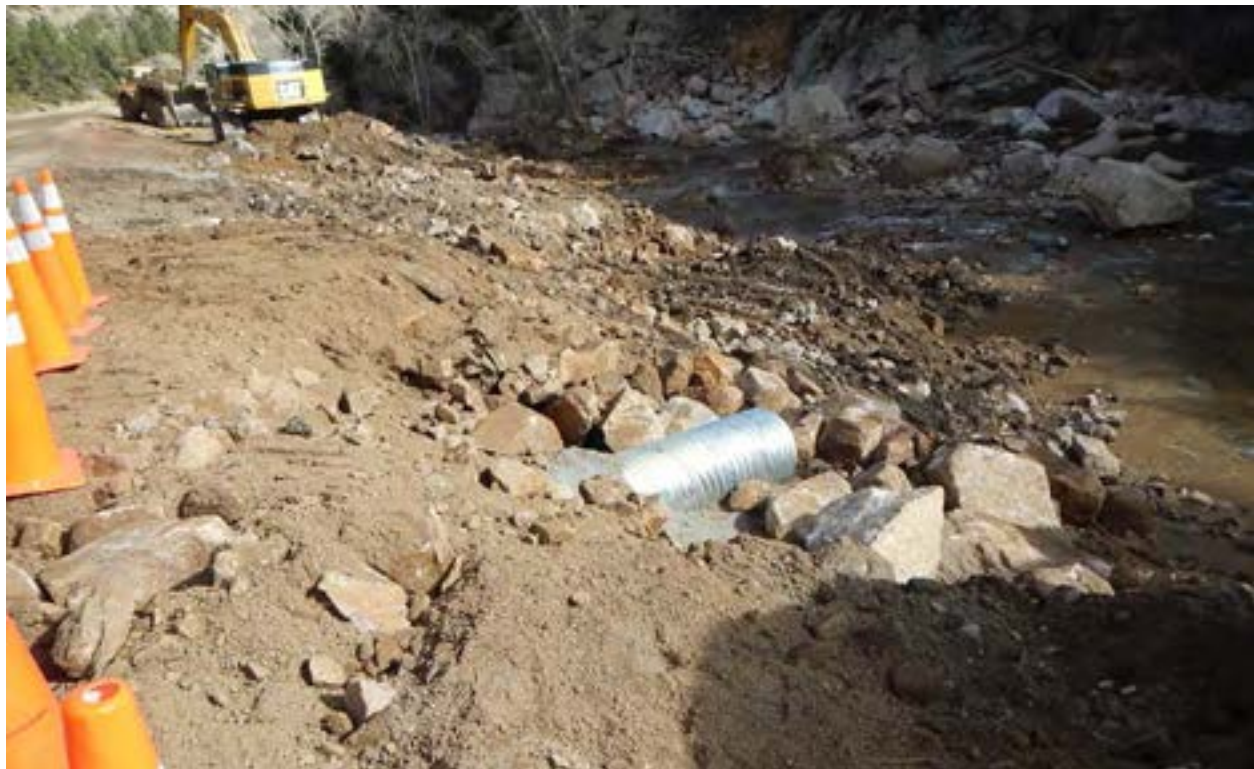
Figure 54 - MP 26.2, CMP Repair.
