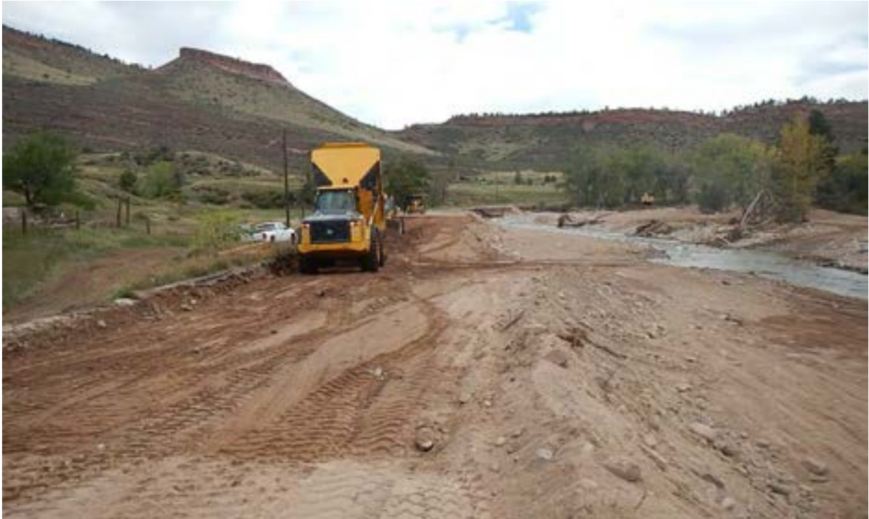
Figure 68 - MP 31.2, Facing northeast, ER Roadway repairs.
