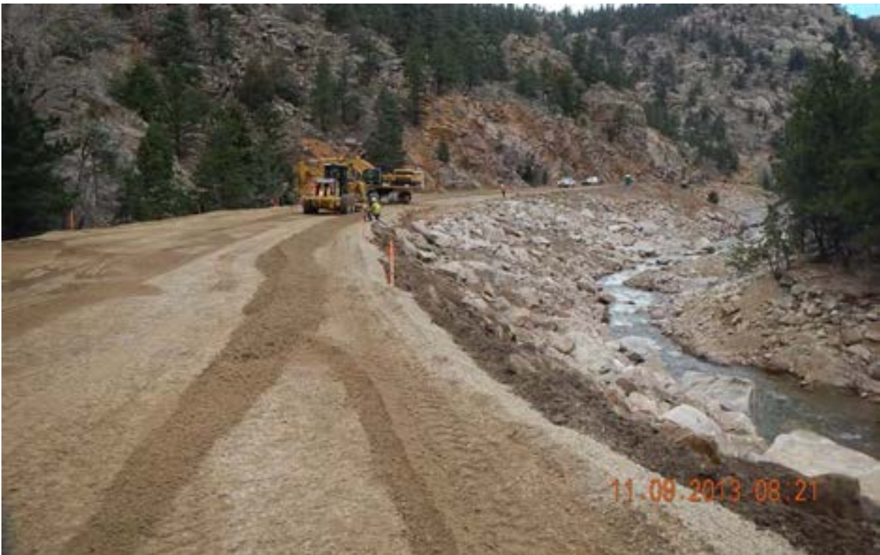
Figure 58 - MP 27.2, Facing north, Roadway repair.
