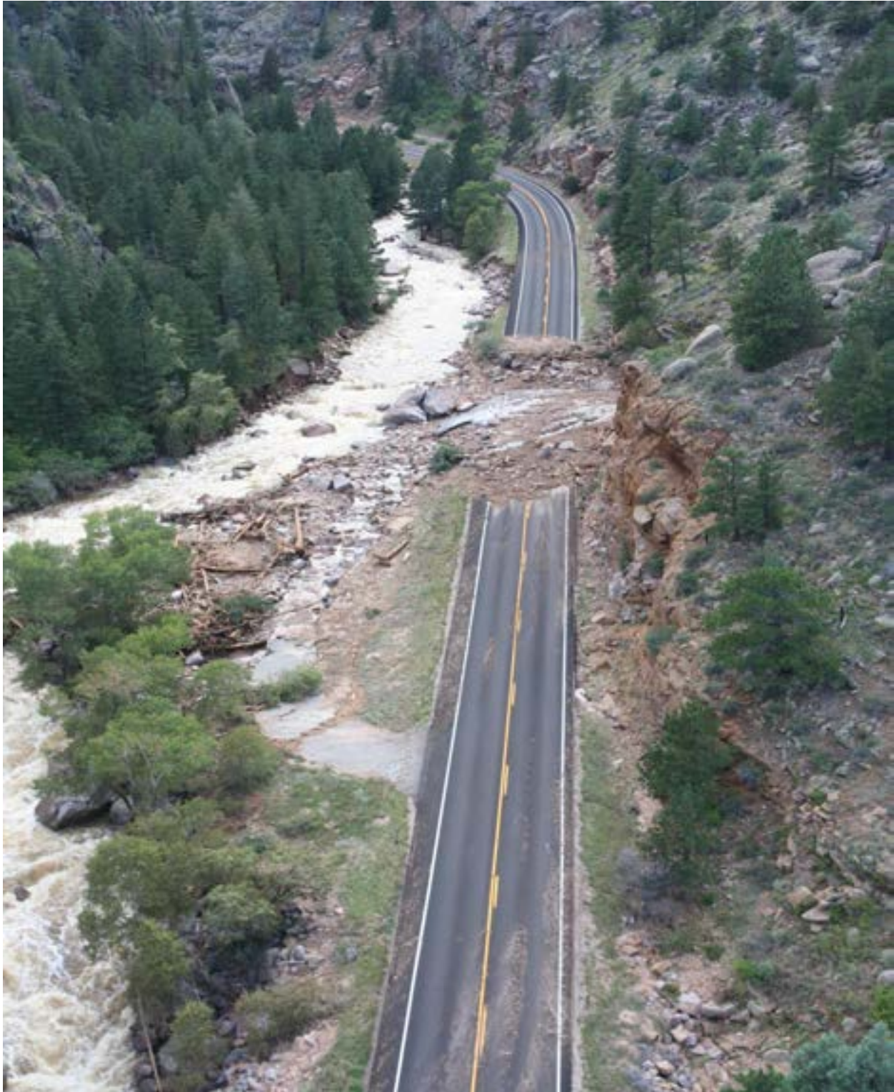
Figure 33 - MP 26.25, Rock slide and debris covering both roadway lanes.
