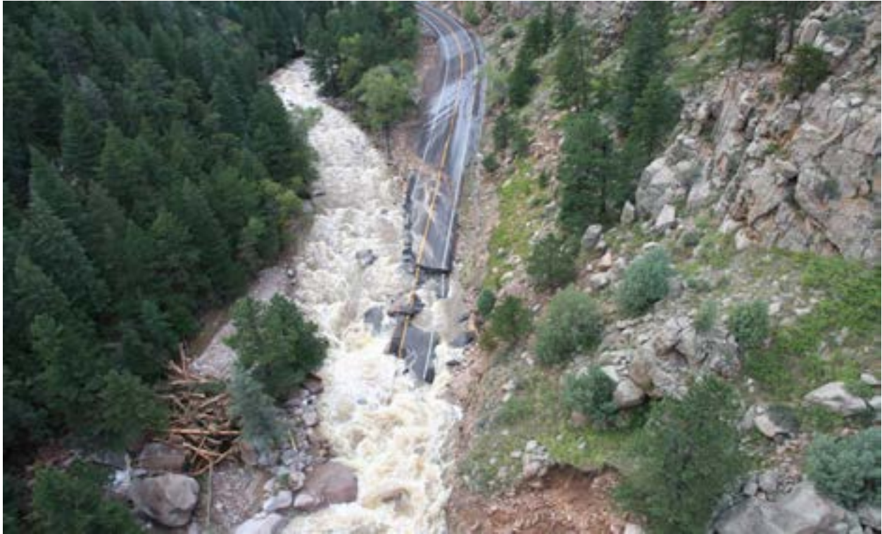
Figure 34 - MP 26.61, Complete roadway loss due to overtopping.
