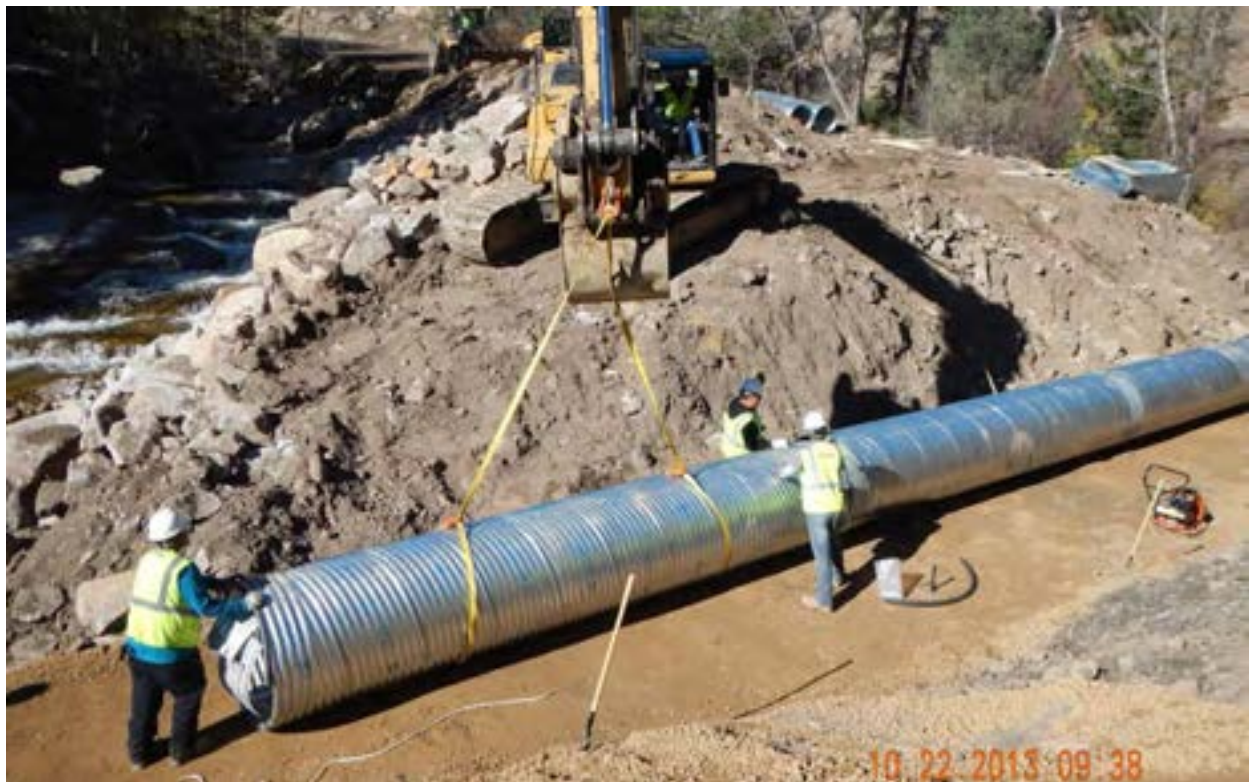
Figure 48 - MP 23.8 Facing northwest, CMP repair.
