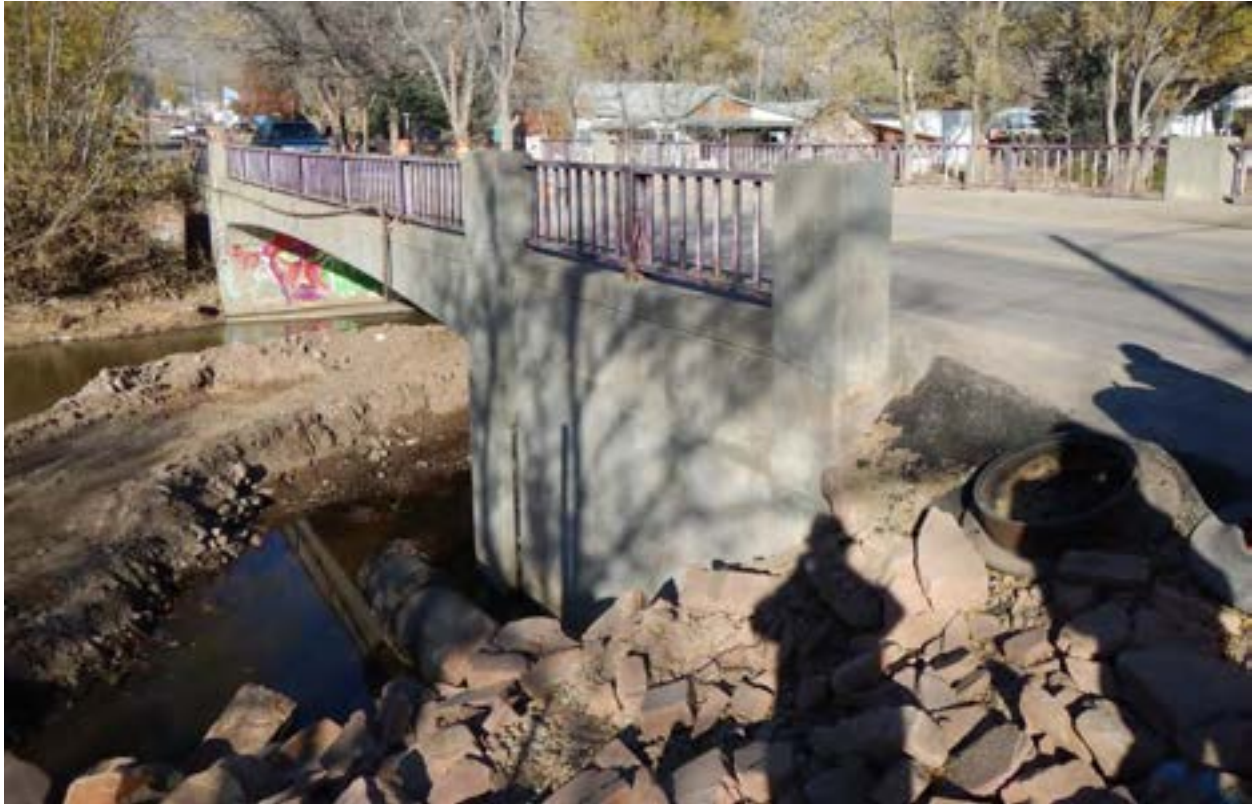
Figure 79 - MP 32.98, Facing northeast, Structure D-15-A temporary access.
