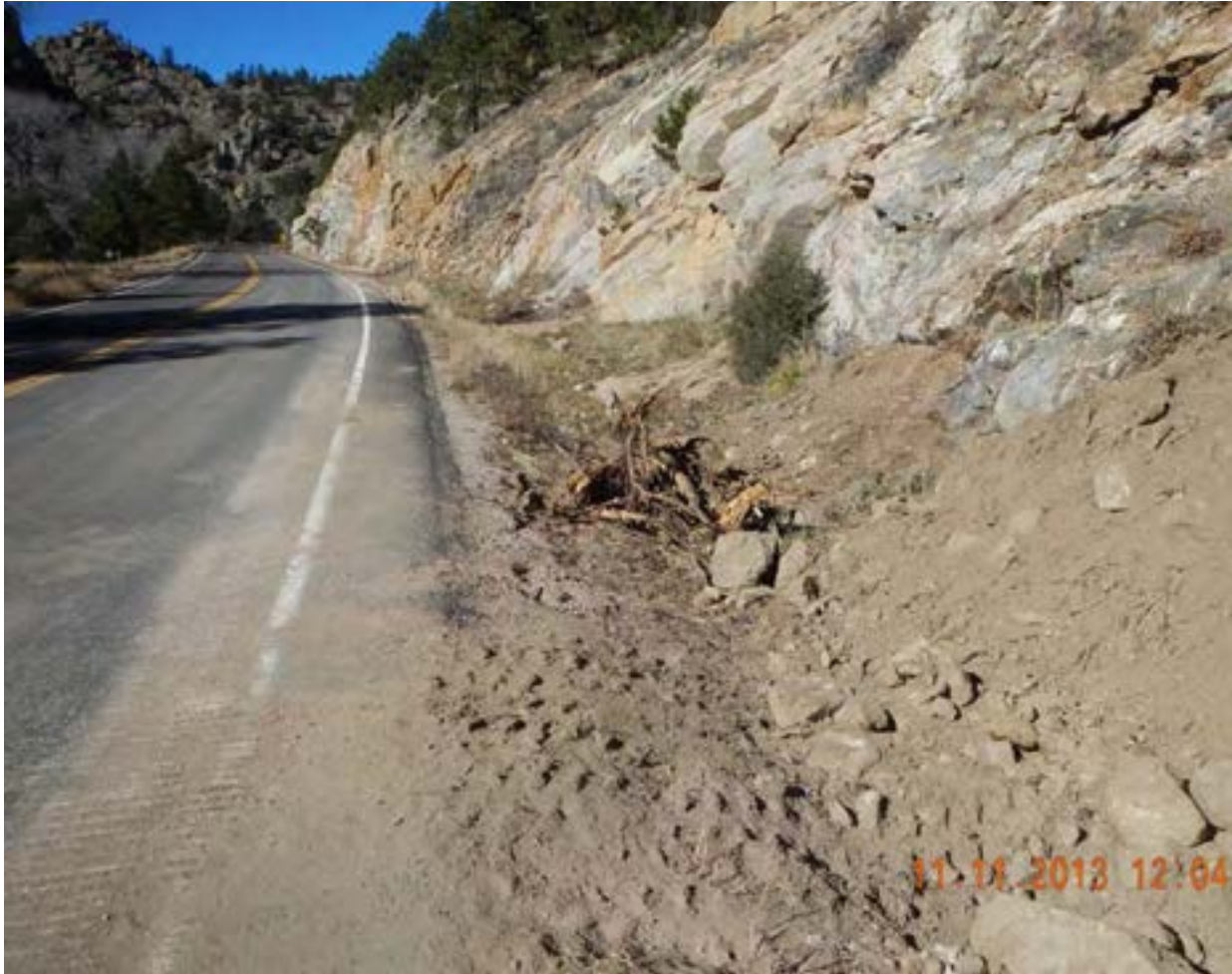
Figure 21 - MP 22.95, Removal of material from slide and regarding of westbound roadside ditch.
