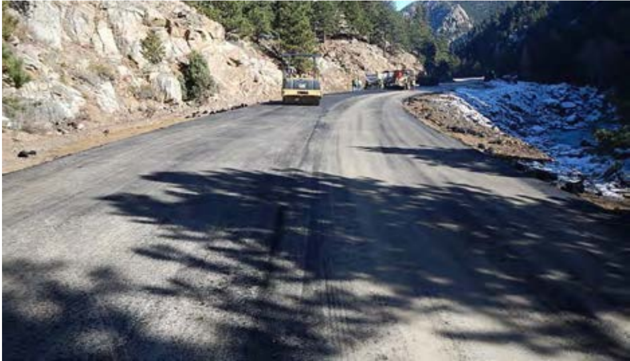
Figure 51 - MP 25.5 Facing east, Roadway repair.
