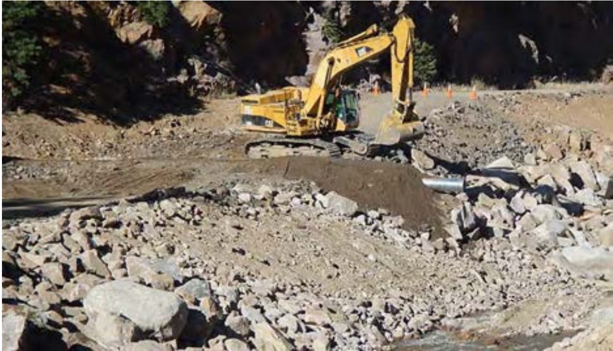
Figure 57 - MP 27.2, Facing north, Roadway and CMP repair.
