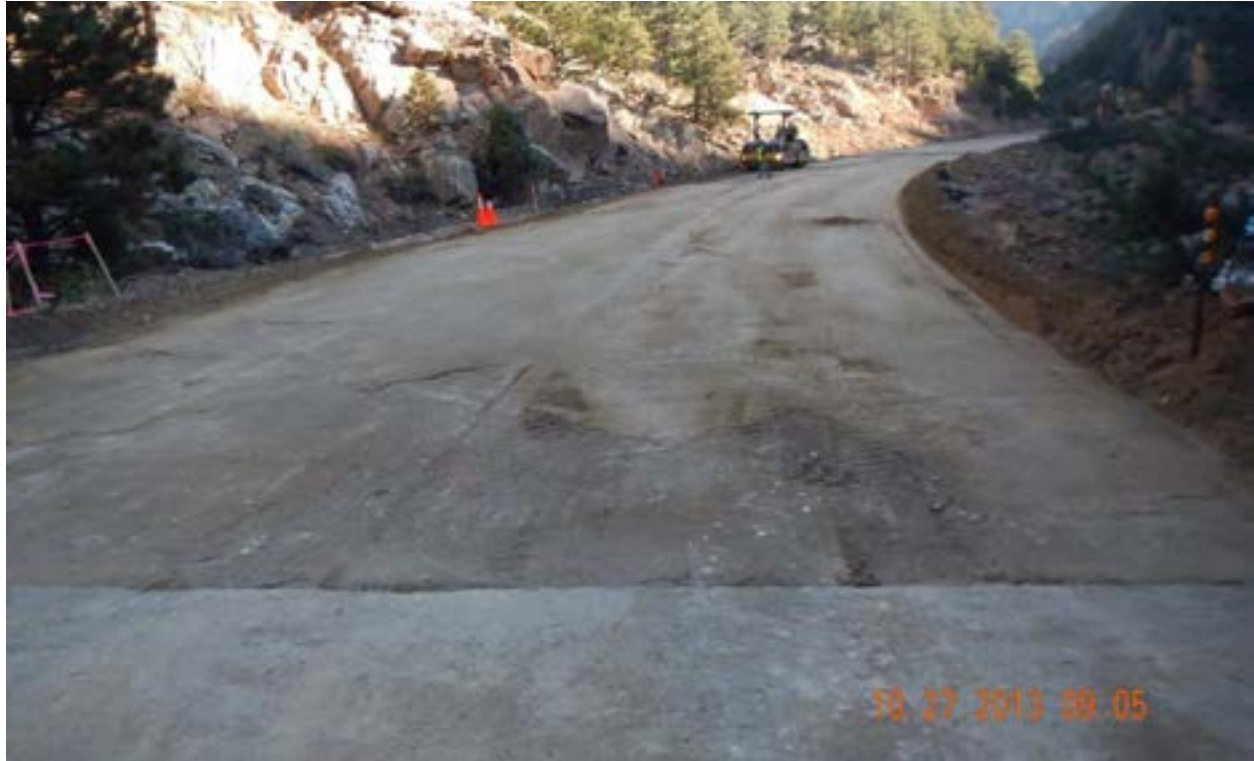
Figure 49 - MP 24.7 Facing northeast, Roadway repair.
