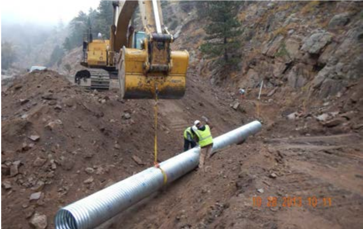
Figure 55 - MP 26.5, CMP repair.
