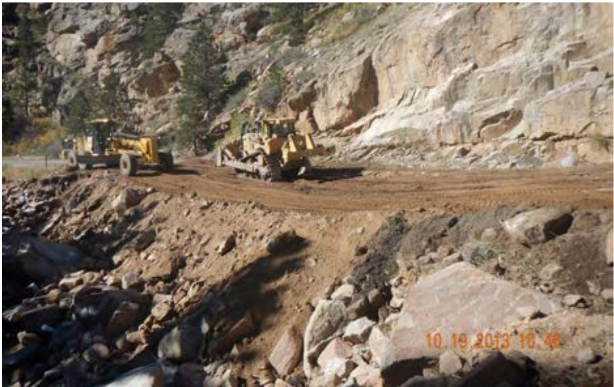
Figure 52 - MP 25.9 Facing west, Roadway repair.
