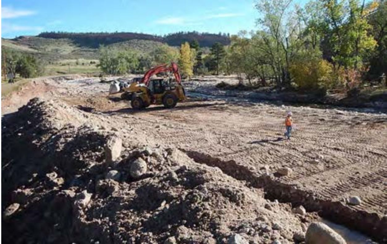
Figure 67 - MP 31.2, Facing southwest, ER Roadway repairs.
