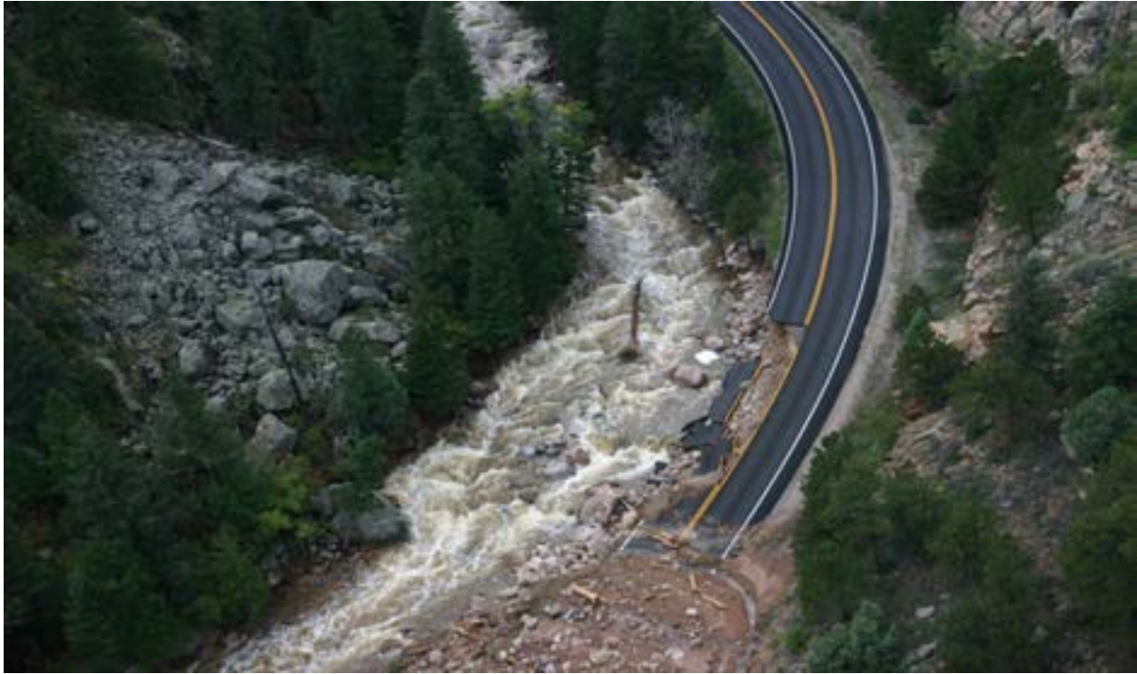
Figure 28 - MP 24.75, Rock slide and debris covering roadway lanes, embankment and roadway washout.
