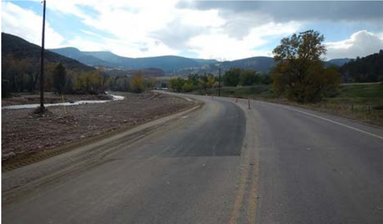
Figure 70 - MP 31.2, Facing southwest, ER Roadway repairs.
