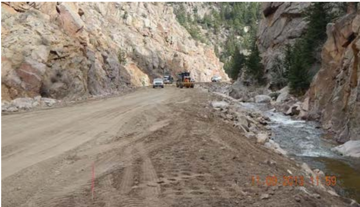
Figure 56 - MP 26.9, Facing northeast, Roadway repair.
