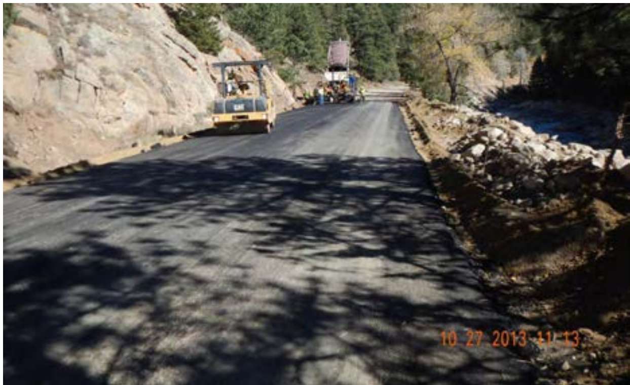
Figure 50 - MP 25.3 Facing east, Roadway repair.
