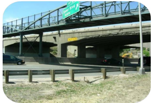
Existing Speer Blvd over I-25 ML; Central Denver
