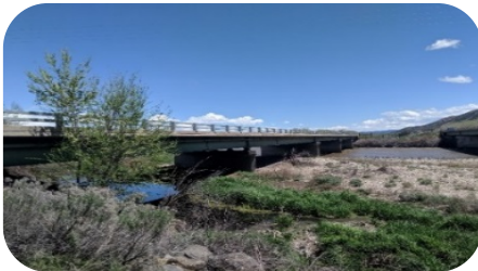
I-70 WB over Colorado River; Garfield County
