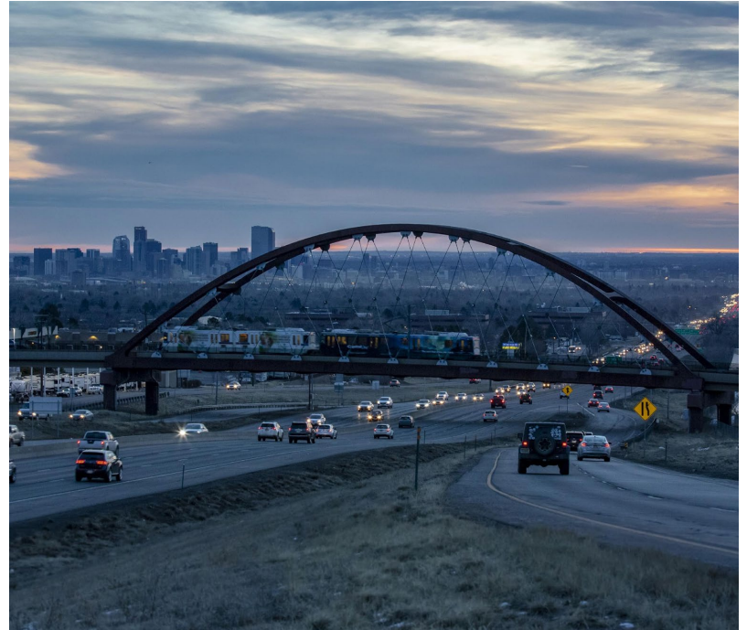
Light Rail bridge over 6th Avenue with view of downtown
