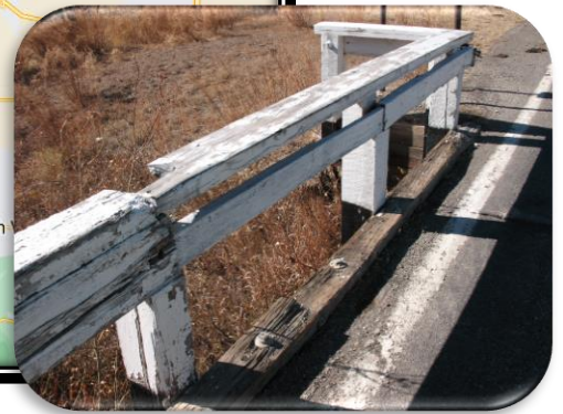
Splintering and Damage to L-11-C Rail
