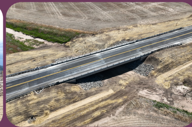
SH 61 ML over Surveyor Creek Region 4 | Washington
