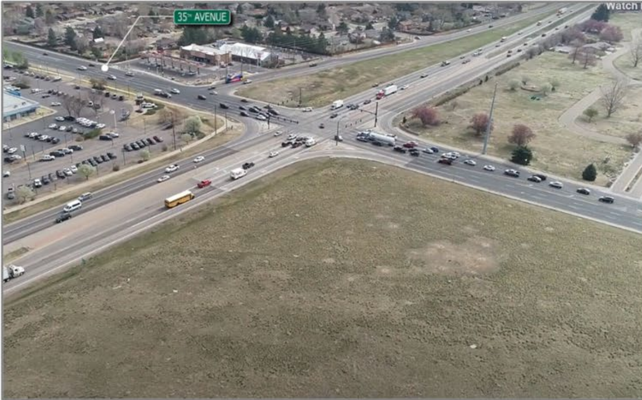
Current At-Grade Signalized Intersection
