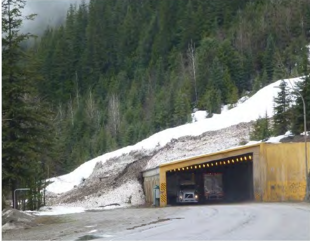
Figure 6. CDOT has a long history of avalanche research. A 2020 research report examined the design and use of snow sheds to protect traffic, such as this one near Rogers Pass in British Columbia.
