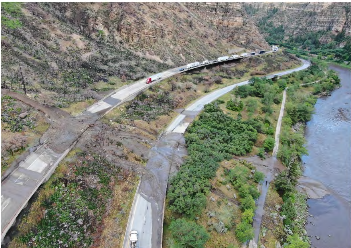
Figure 5. Debris flow damage to Interstate 70 through Glenwood Canyon, CO following heavy rain on the Grizzly Creek fire burn scar.
