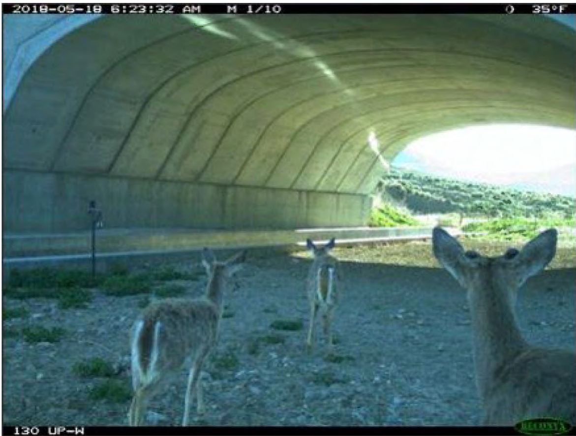
Figure 7. Mule deer approaching the new wildlife underpass for State Highway 9. CDOT research documented a 92% reduction in wildlife-vehicle crashes following the addition of wildlife crossings, fencing, escape ramps, and other treatments at key locations along SH9.
